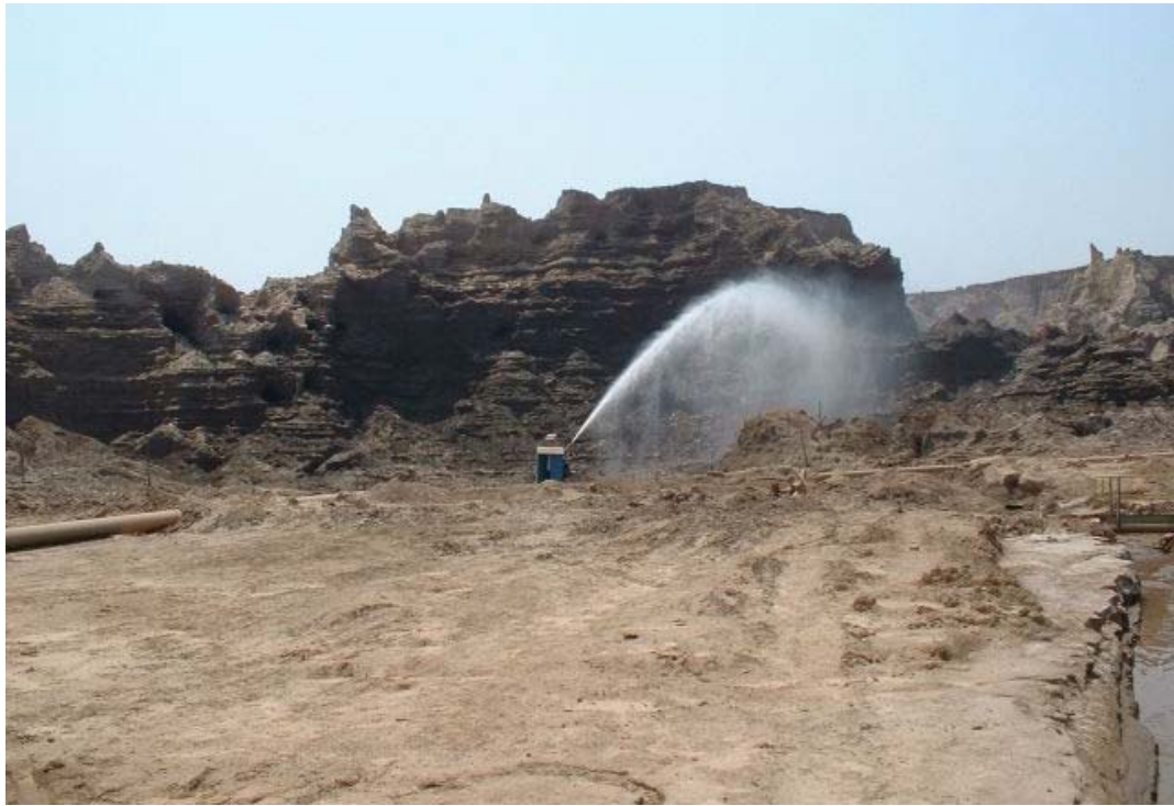
Photo 3.2a: Hydraulic monitoring from the bottom up.
