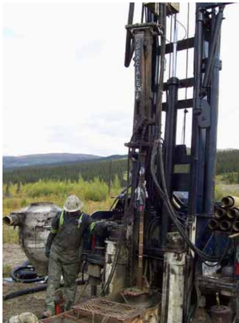
Photo II-4 Photo II-5 SPT Data Set up with Automatic Trip Hammer and Instrumented Rod for Energy Measurements During Mud Rotary Drilling at the Cross Valley Dam
