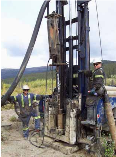
Photo II-3 SPT Data Set up with Automatic Trip Hammer and Instrumented Rod for Energy Measurements During Becker Open Hole Test at the Cross Valley Dam
