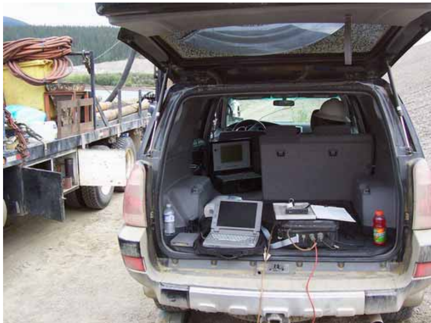
Photo II-2 PDA Data Acquisition System and Monitoring Equipments at the Intermediate Dam
