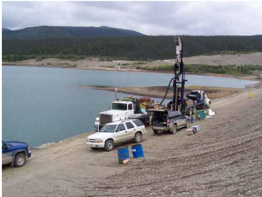
Photo II-1 BPT at the Intermediate Dam Downstream Berm Using HAV180 Drill Rig and Instrumented Casing
