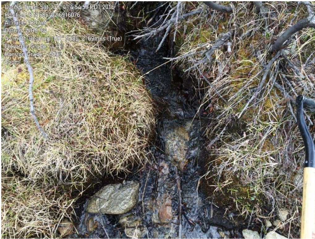
Photo 19. Seep on the east bank of the FCD
