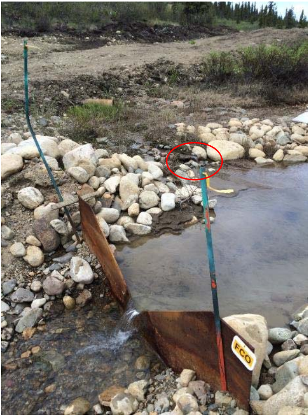
Photo 21. FCO weir with West Ditch culvert and discharge point (circled)
