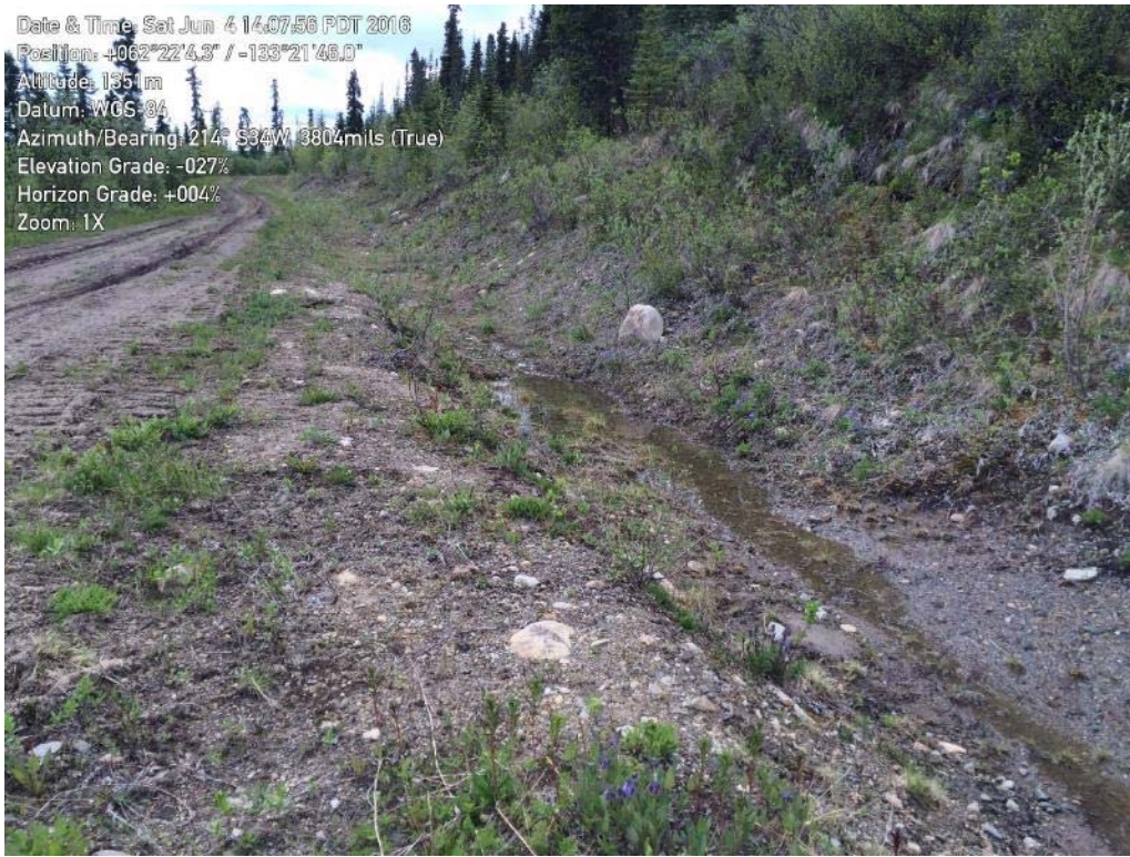
Photo 35. Beginning of flow in West Valley Interceptor Ditch, looking upstream
