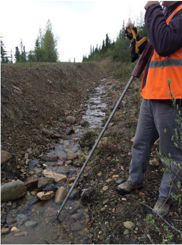
Photo 37. Streambed piezometer, ready for installation
