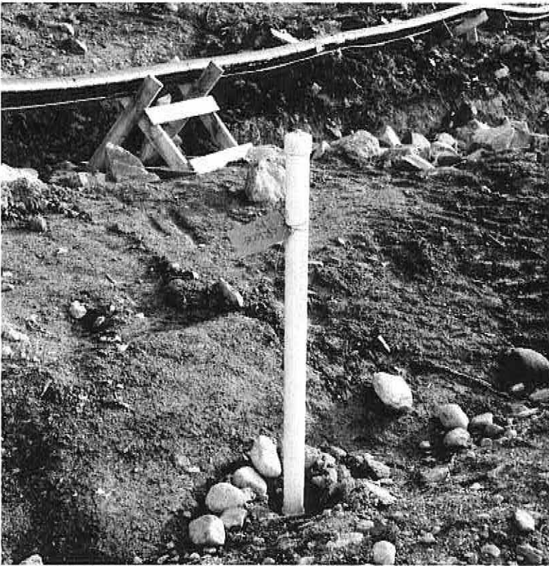
The repaired monitoring well, SRK09-SP5, Sept 11, 2009.
