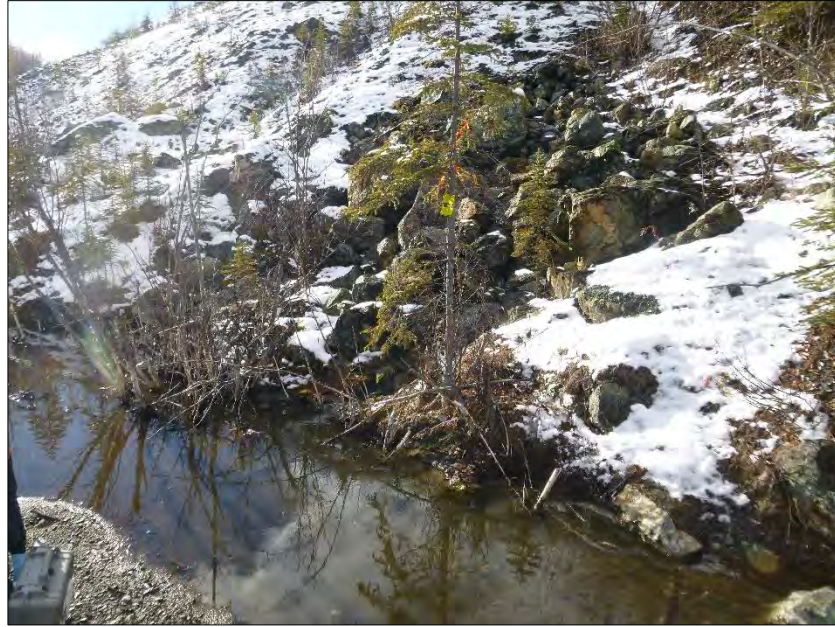
Photo 17: View of seepage site GWCC-2 (toe of waste rock dump, flowing into ponded area). Photo taken and staff gauge installed on October 2 nd , 2015.
