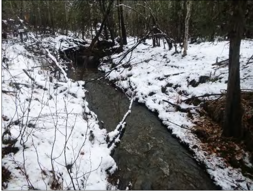
Photo 11: Downstream view of Site R4 (Eagle Creek, upstream of culvert). Photo taken on September 30 th , 2015
