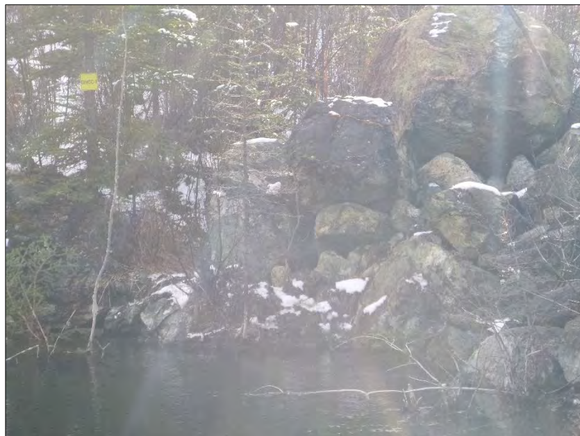
Photo 16: View of seepage site GWCC-1 (toe of waste rock dump, flowing into ponded area). Photo taken and staff gauge installed on October 2 nd , 2015.
