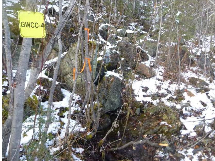
Photo 19: View of seepage site GWCC-4 (toe of waste rock dump, flowing into seepage channel northwest of ponded area). Photo taken and staff gauge installed on October 2 nd , 2015.
