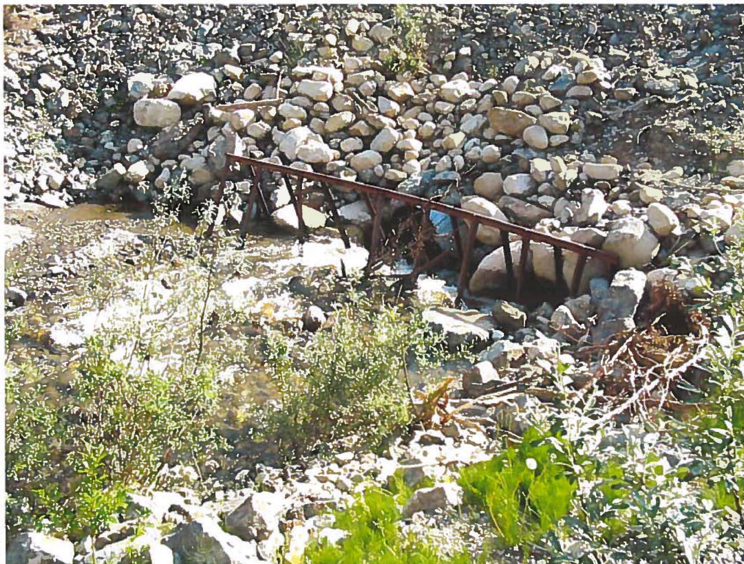
Photo 27: Trash rack at inlet to 1800mm Ø culvert at headworks embankment.
