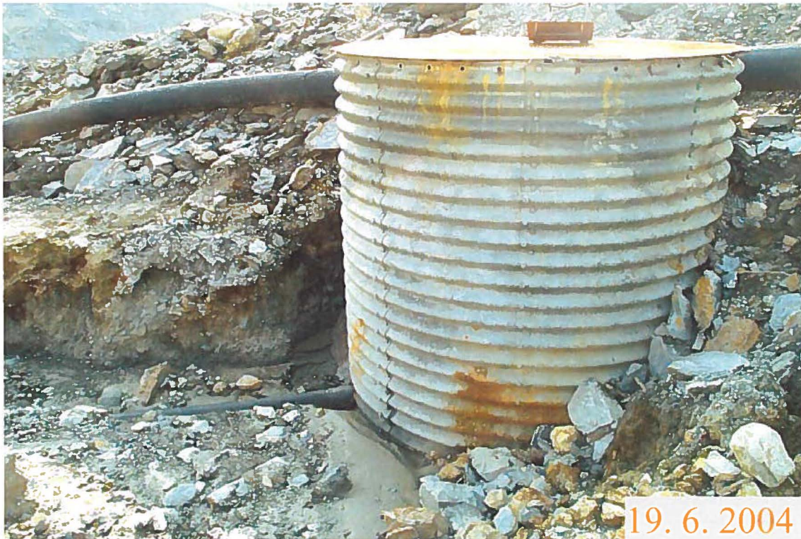
Photo 2: Drop structure
