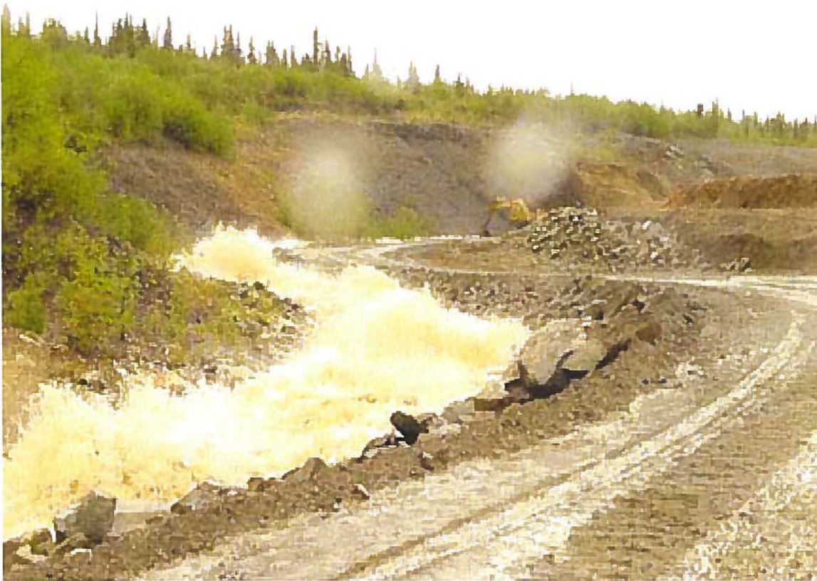
Photo 3: Outfall from 1600mm Ø culvert. (June 8, 2004)
