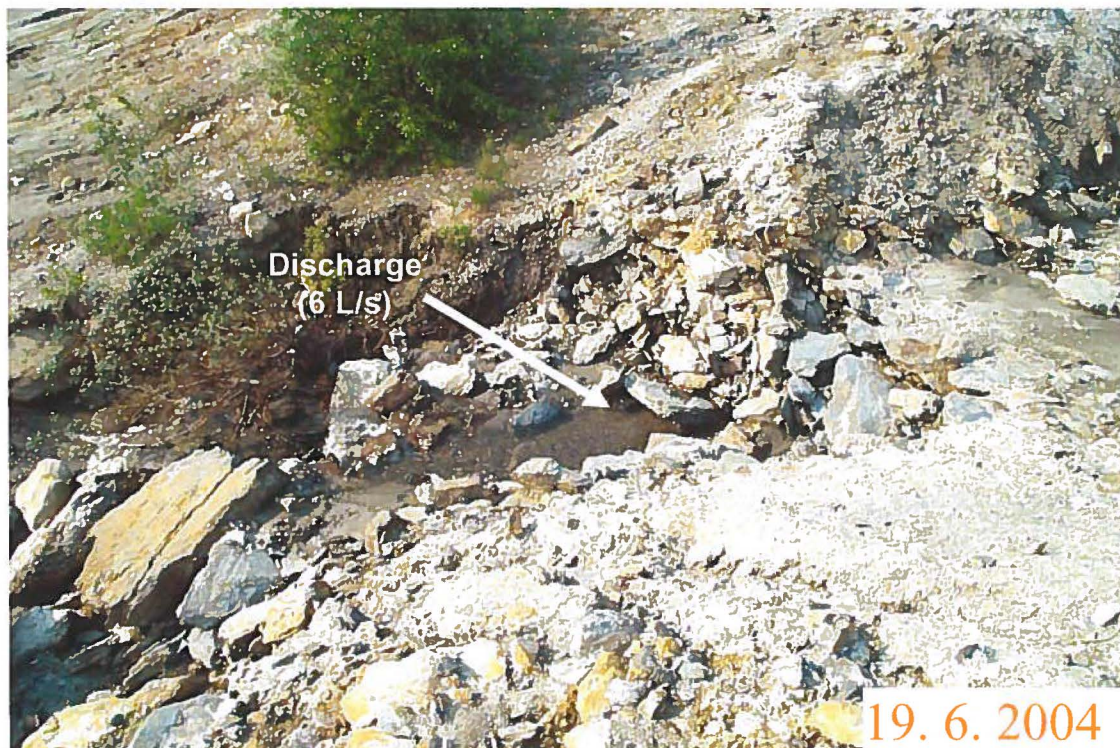
Photo 16: Discharge zone below drop structure.
