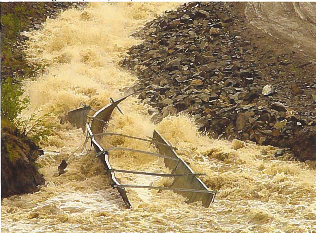
Photo 8: Flume sections at entrance to Plunge Pool (June 8, 2004).
