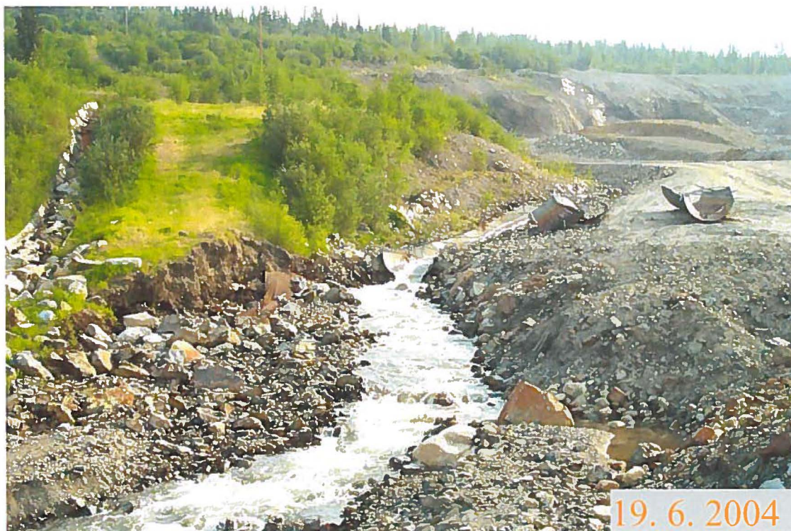
Photo 28: Plunge Pool at bottom of flume.
