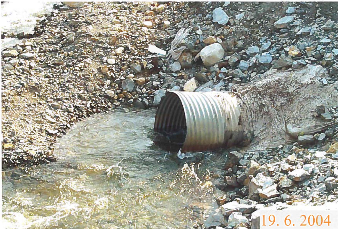
Photo 4: Inlet to 2000mm Ø culvert at Plunge Pool.
