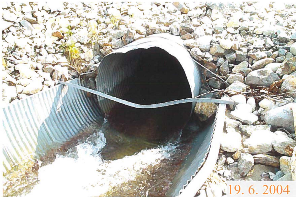
Photo 5: Outlet of 1500mm Ø culvert beneath Headworks Embankment.
