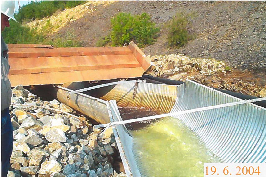
Photo 33. Connection between original and recently installed flume sections.
