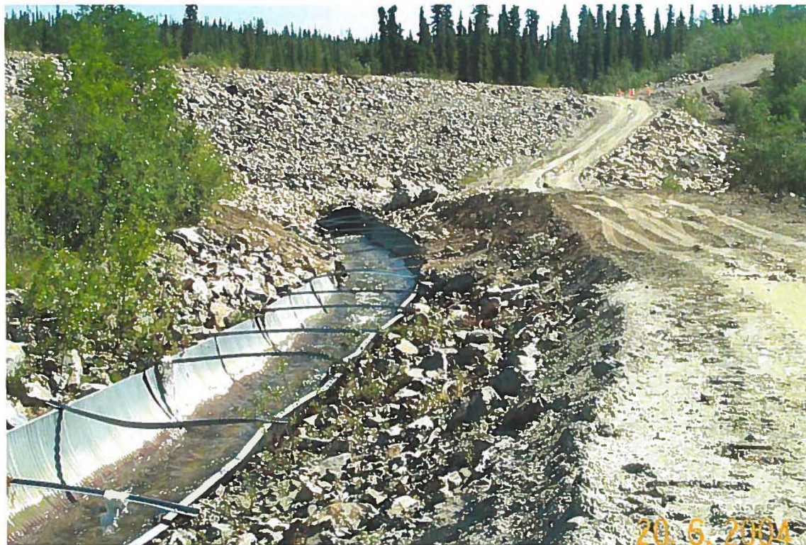
Photo 6: Transition from 1500mm Ø culvert to 2400mm ½ culvert.
