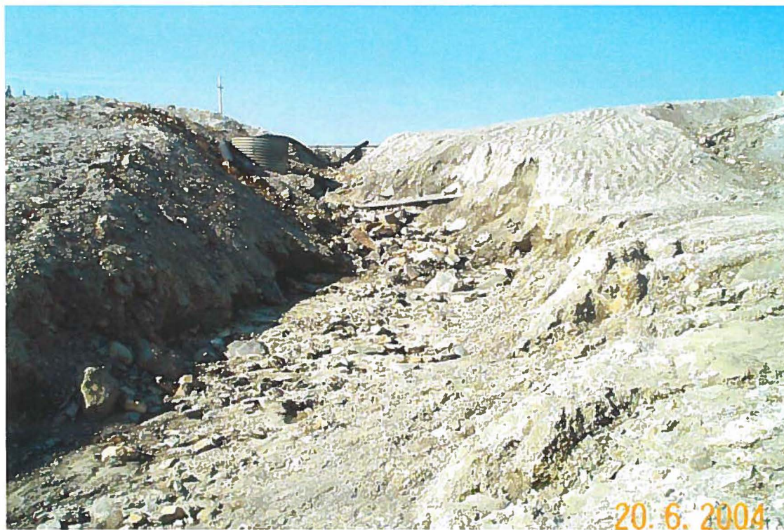
Photo 18: Discharge channel below drop structure.
