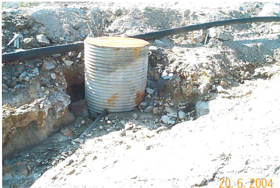
Photo 17: Drop structure.
