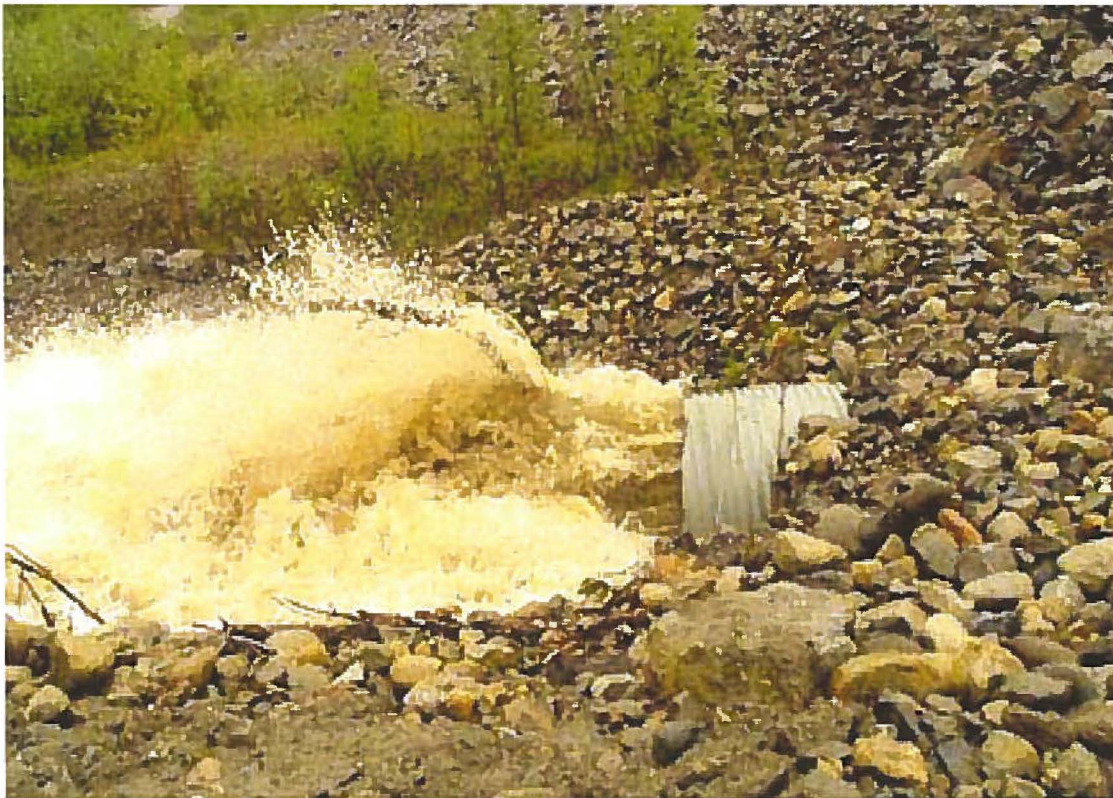
Photo 38: Outlet of 1500mm Ø culvert beneath Headworks Embankment (June 8/04)
