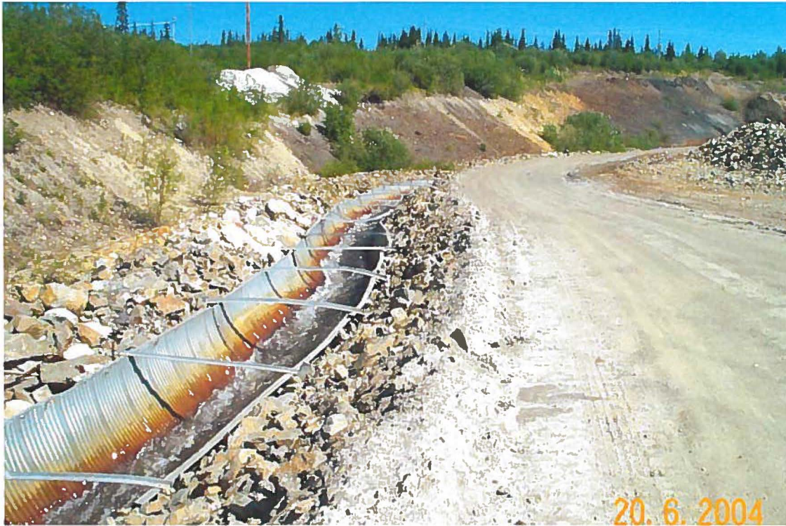
Photo 31: Middle section of flume and channel.
