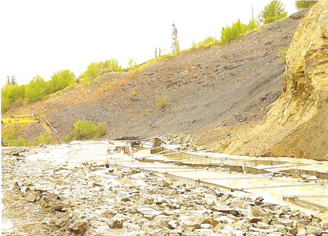
Photo 13: Backhoe restraining flume section from lifting (June 8, 2004).
