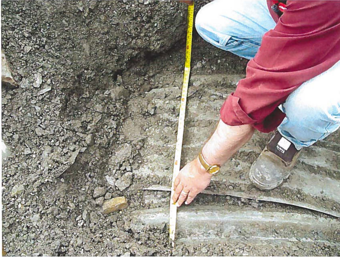
Photo 23: Coupling at 2000mm Ø joint with nipple.
