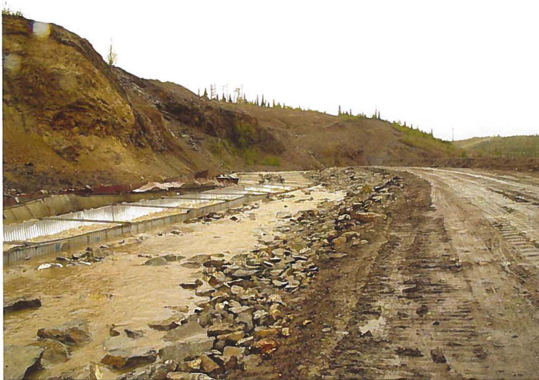
Photo 11: New flume section with old flume still in place (June 8, 2004).
