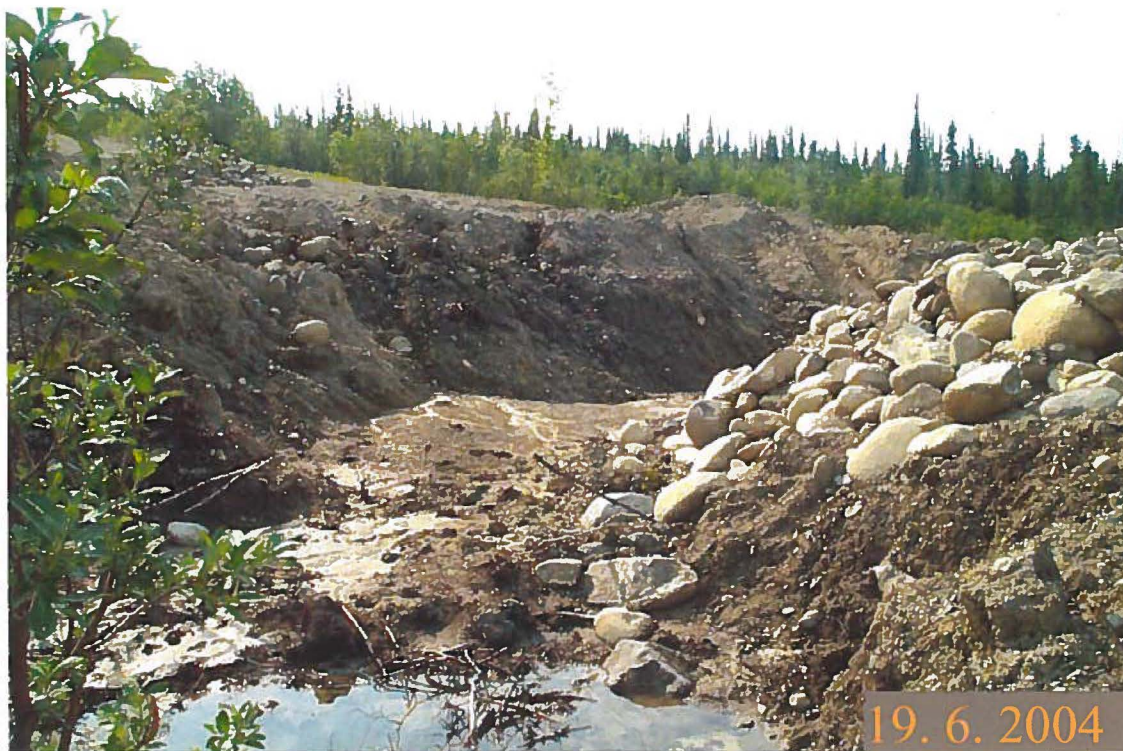
Photo 25: Excavated channel on south abutment of headworks embankment.
