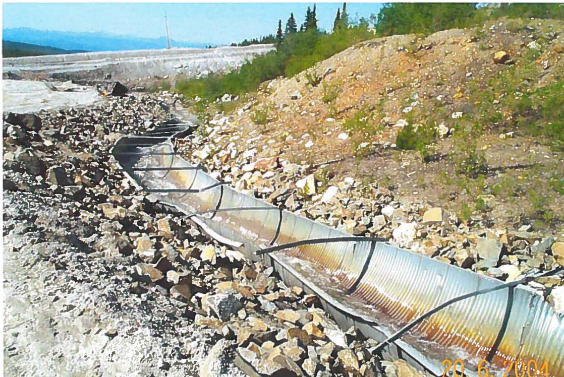
Photo 29: Lower sections of flume and channel.
