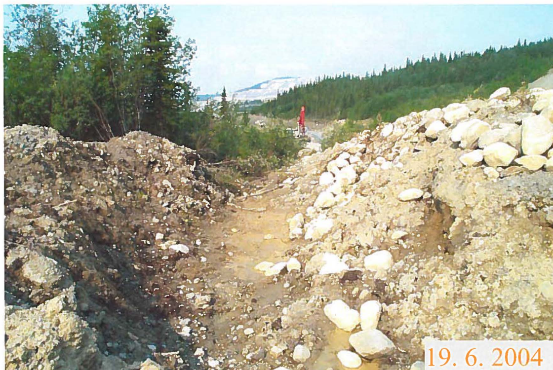
Photo 26: Excavated channel on south abutment of headworks embankment.
