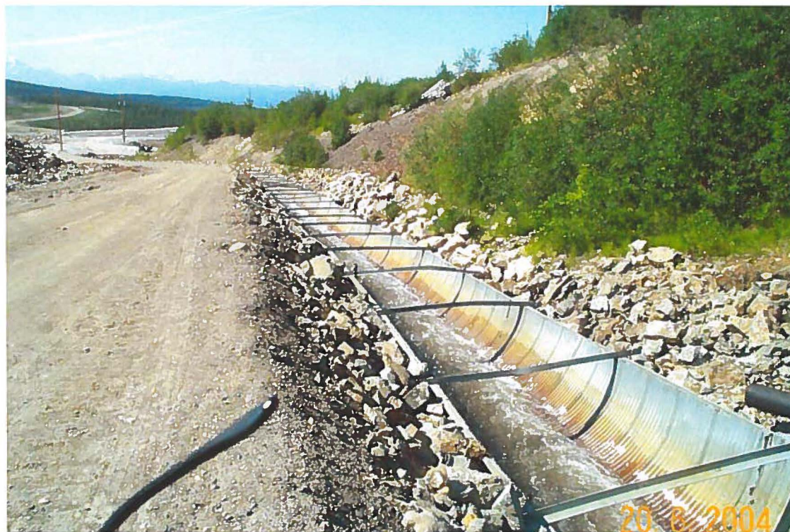
Photo 30: Transition between lower and middle reaches of flume and channel.
