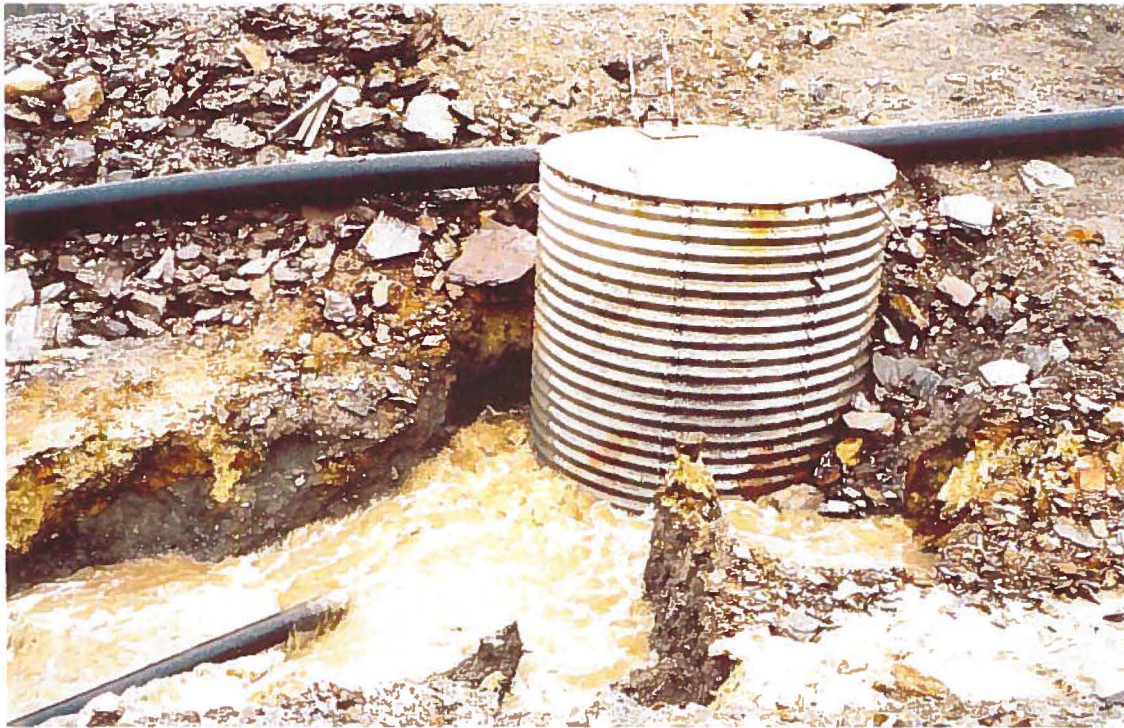
Photo 37: Drop structure during flood event. (June 8, 2004)
