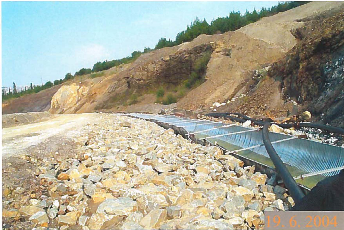
Photo 35: New flume section.
