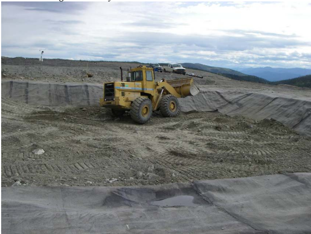
Photo 16: Placing the second layer of Waste Rock Backfill on L#2
