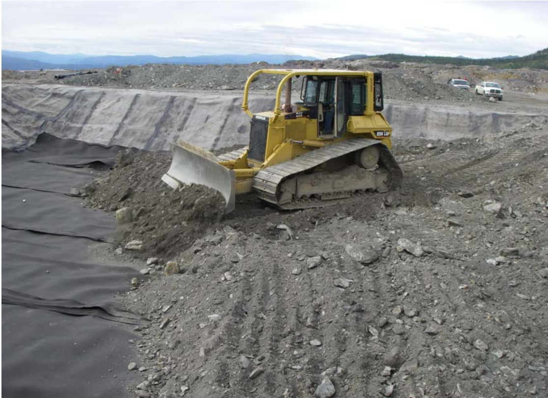
Photo 15: Placing the First Layer of Waste Rock backfill in L#1
