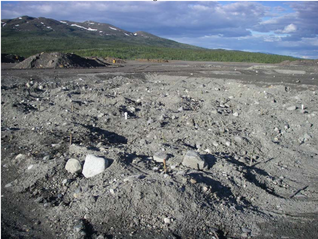
Photo 26: Hummocky finish of Till Surface on L#1
