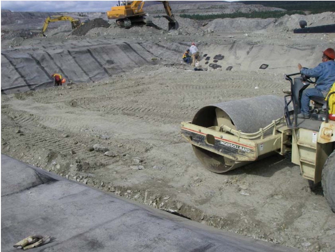
Photo 17: Compacting the Waste Rock Backfill
