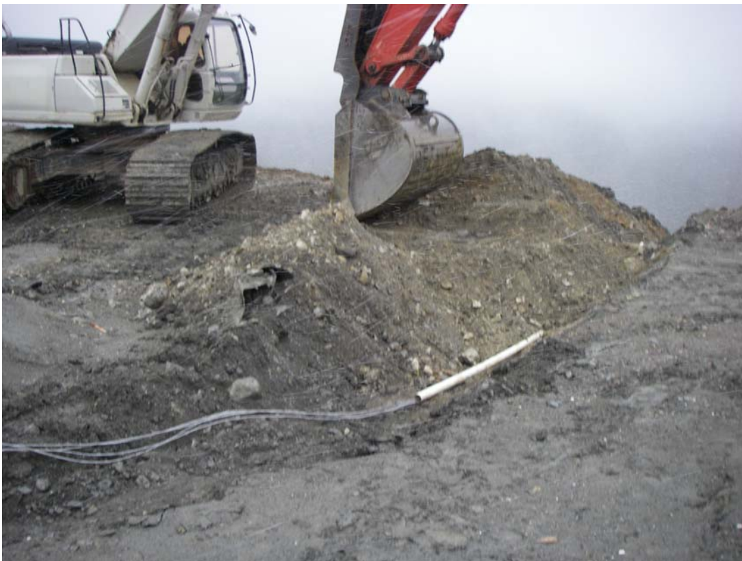
Photo 20: Backfilling the Wiring Trench
