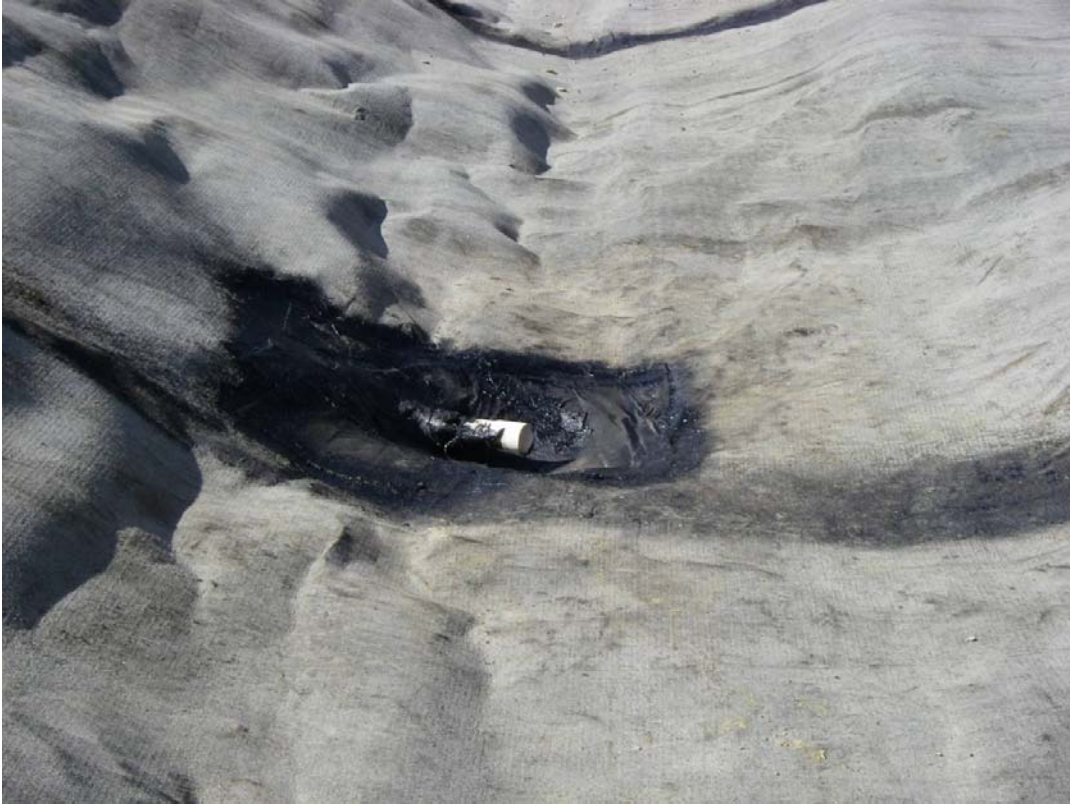
Photo 11: Perimeter Drainage Pipe welded into the Liner
