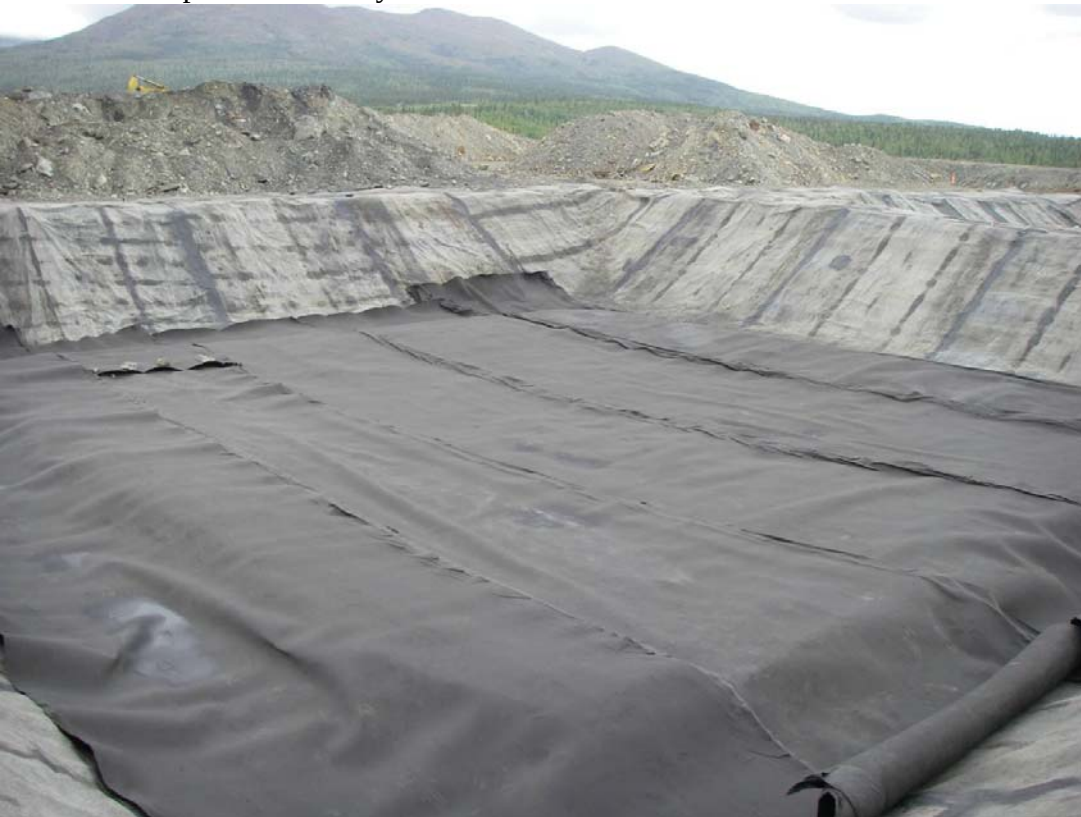
Photo 10: Drainage Geo-Net placed in L#1
