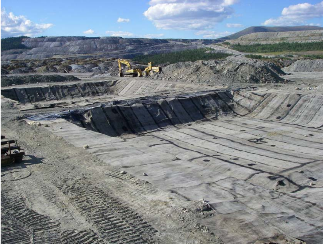
Photo 9: Liner place in both Lysimeters
