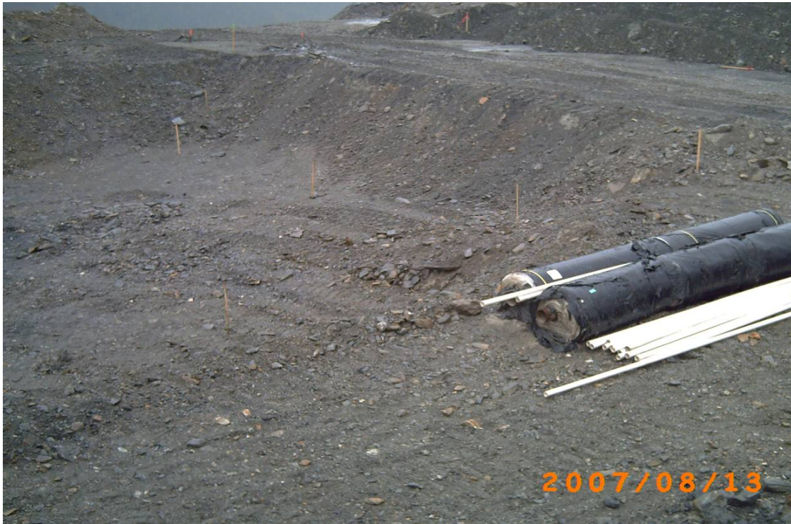
Photo 3: L#1 roughly excavated (Rolls of Bitumen Liner in the right hand side of the picture)
