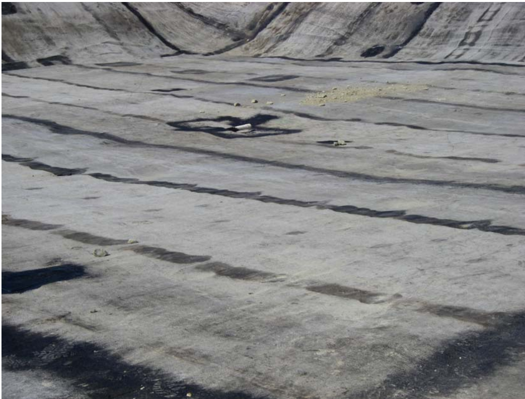
Photo 12: Central Drainage Pipe intake installed and welded into the liner of L#2
