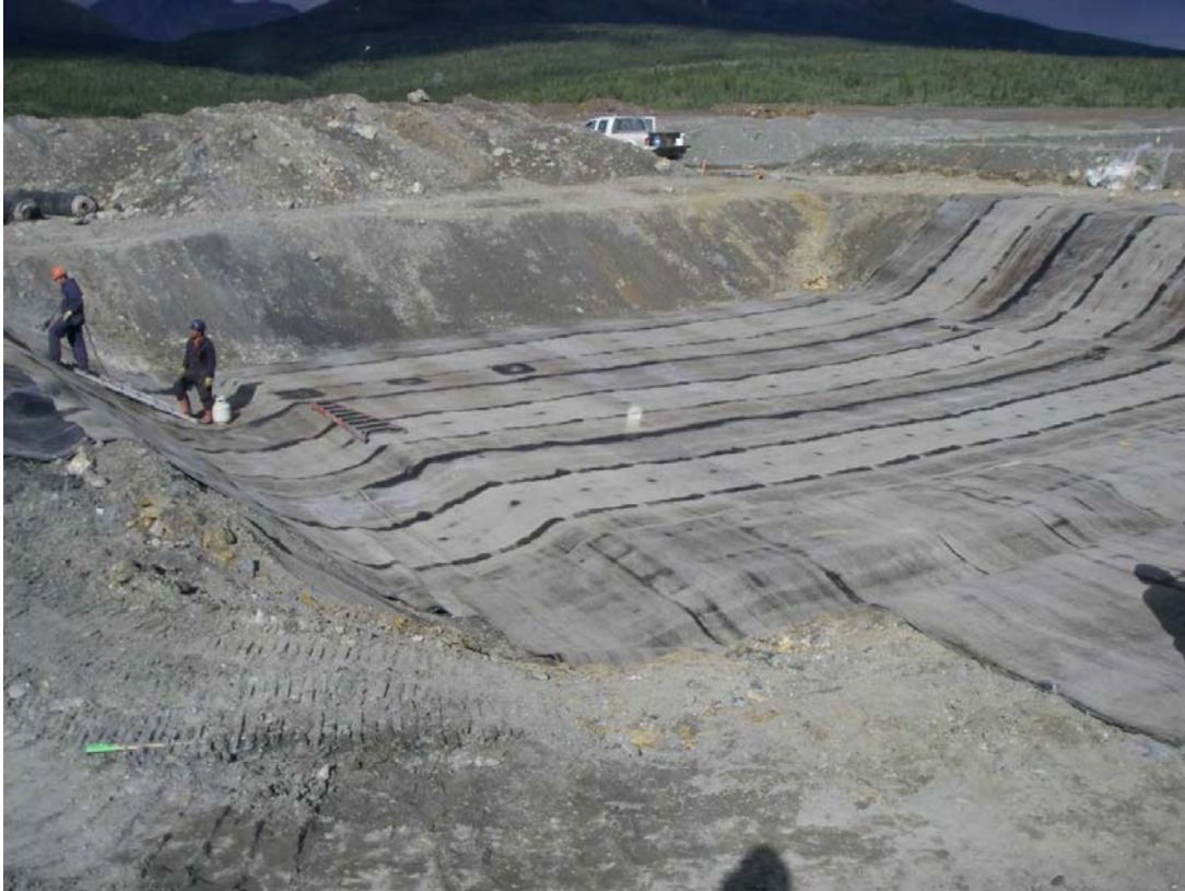
Photo 7: Partially placed liner in L#2
