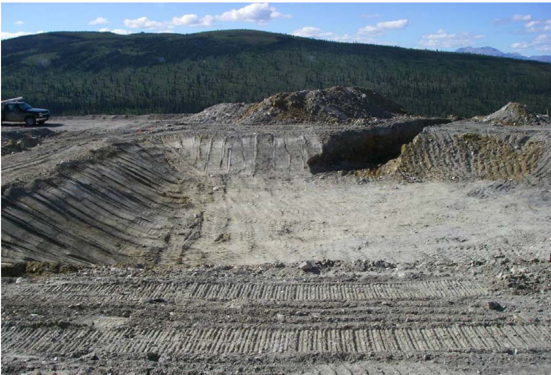
Photo 6: L#2 excavated with drainage pipe trench open
