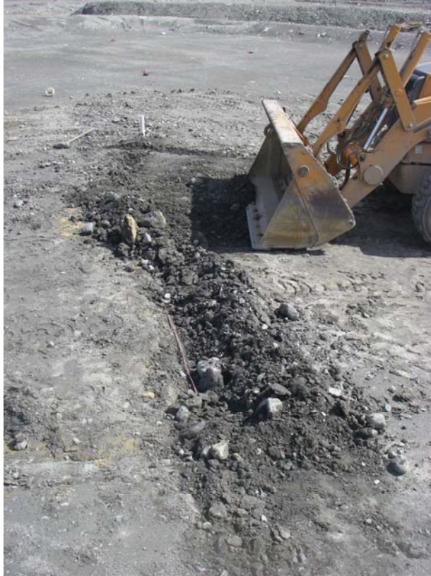
Photo 23: Backfilling the Wire Trench on L#2
