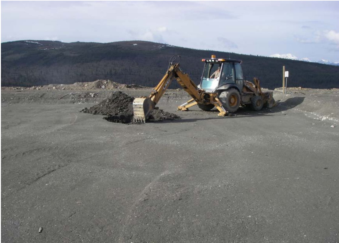
Photo 21: Excavating the Test Pit on L#2 for installation of the Matric Suction Sensors
