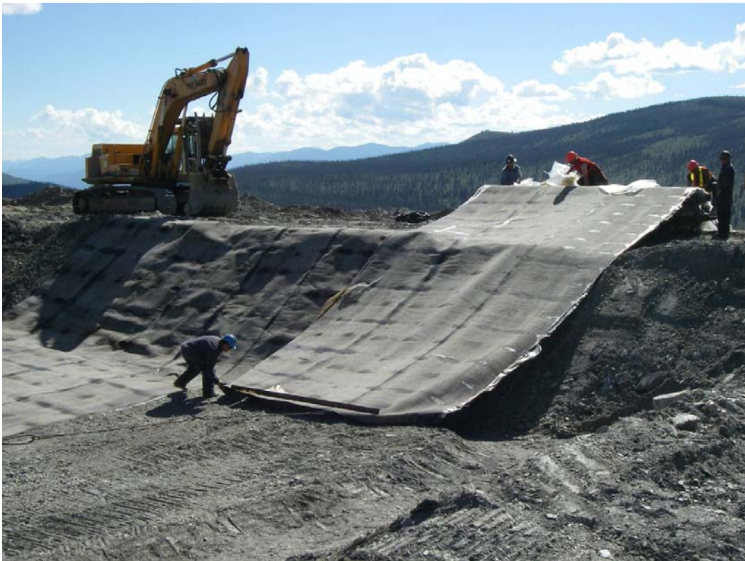
Photo 8: Placing the liner in L#1
