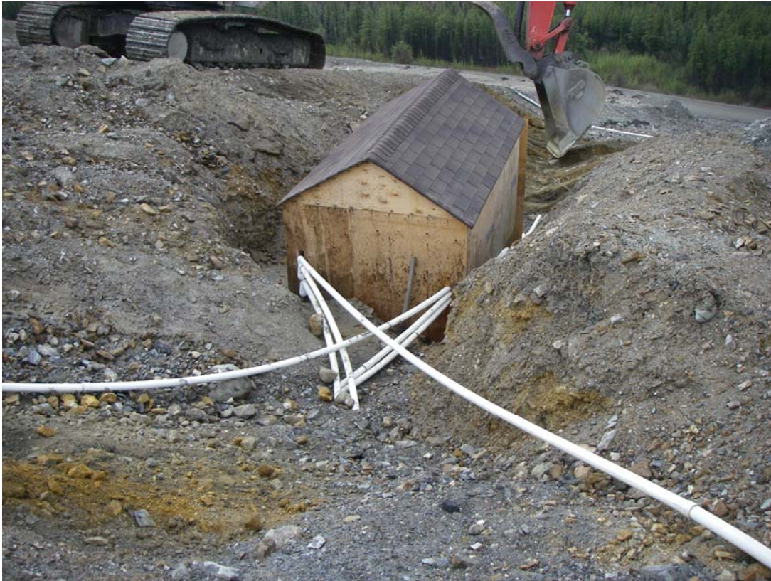
Photo 19: Rear View of Instrument Hut
