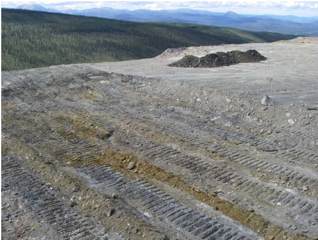
Photo 2: Top layer of Waste Rock removed from the surface of L#1
