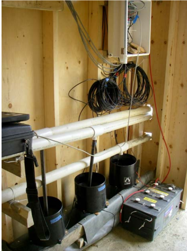
Photo 29: Detail of the Instrument Hut with the CR1000 data logger Housing box on top and the Tipping Bucket Flow Gauges on the Bottom of the photo
