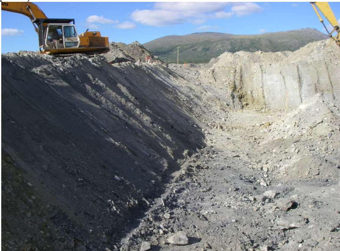
Photo 4: Sloping the sides of L#2
