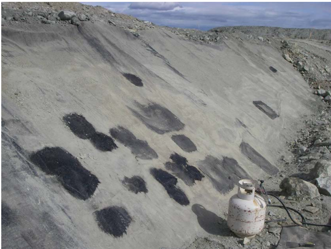
Photo 14: Repaired tears in the Liner on L#2
