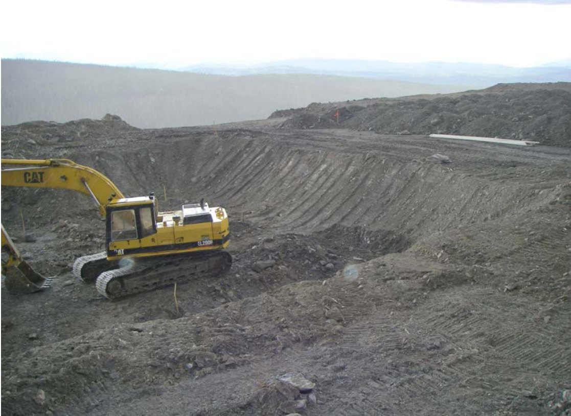
Photo 5: Reshaping the slopes of L#1
