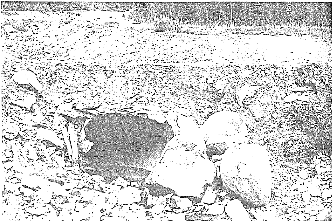
Photo 24 - Outlet of damaged culvert adjacent to Sheep Pad Settling Pond.
