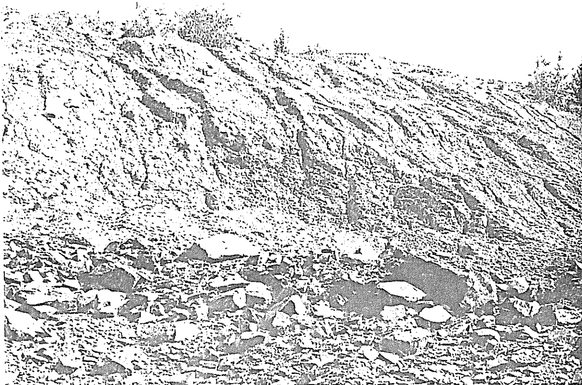
Photo 6 - Excavation above weir 3.
