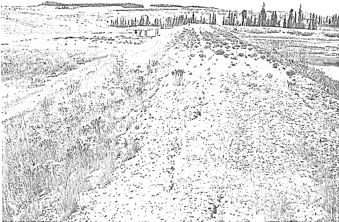
Photo 20 - Crest of sludge pond embankment at treatment plant.
