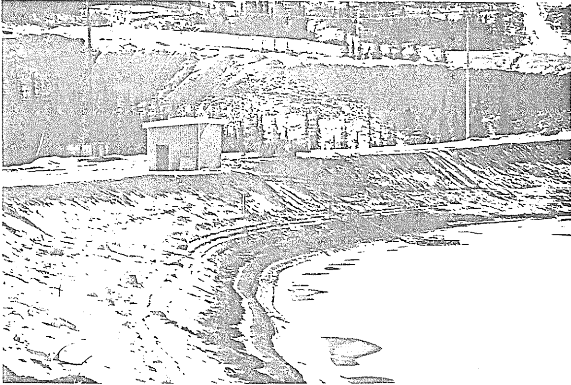
Photo 11 - View of pumphouse on Little Creek Dam
