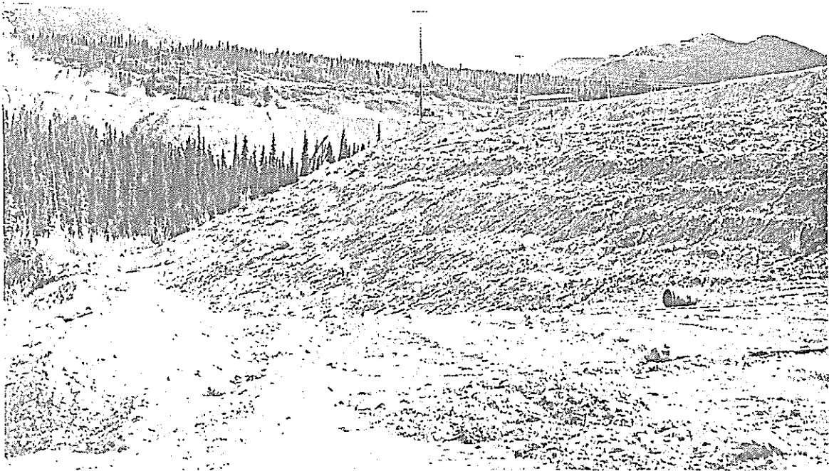
Photo 9 - Downstream slope of Little Creek Dam.
