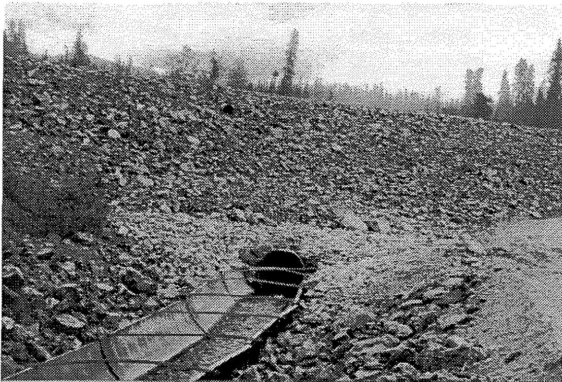
Photo #4b, Vangorda Creek flow restored into flume
