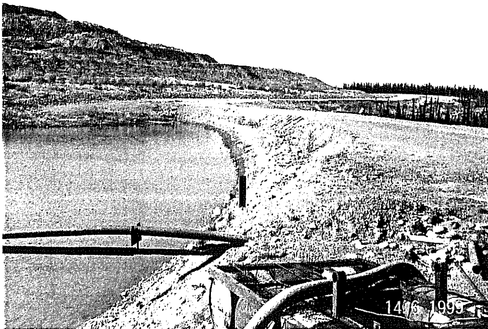
Photo 12: Upstream Face of Little Creek Dam
