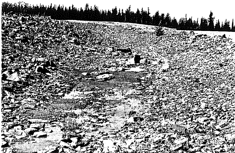
Photo 7: Seepage Collection Ditch on Northside of Waste Dump
