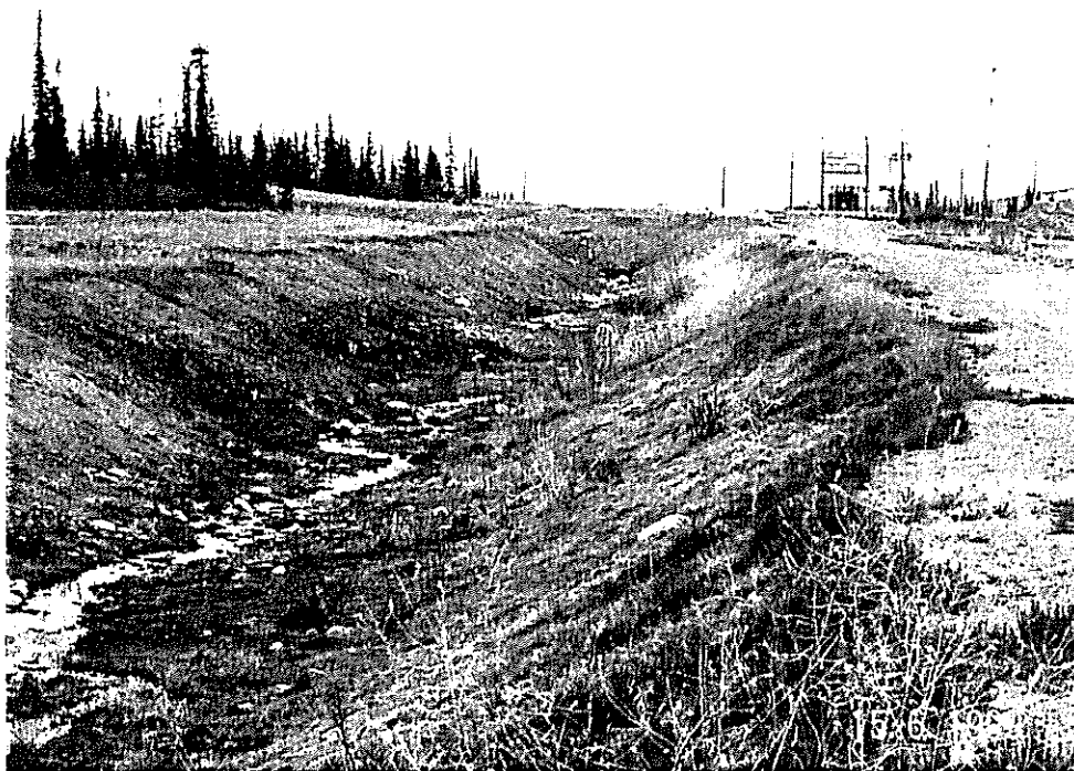
Photo 28: Grum Interceptor Ditch above Treatment Plant
