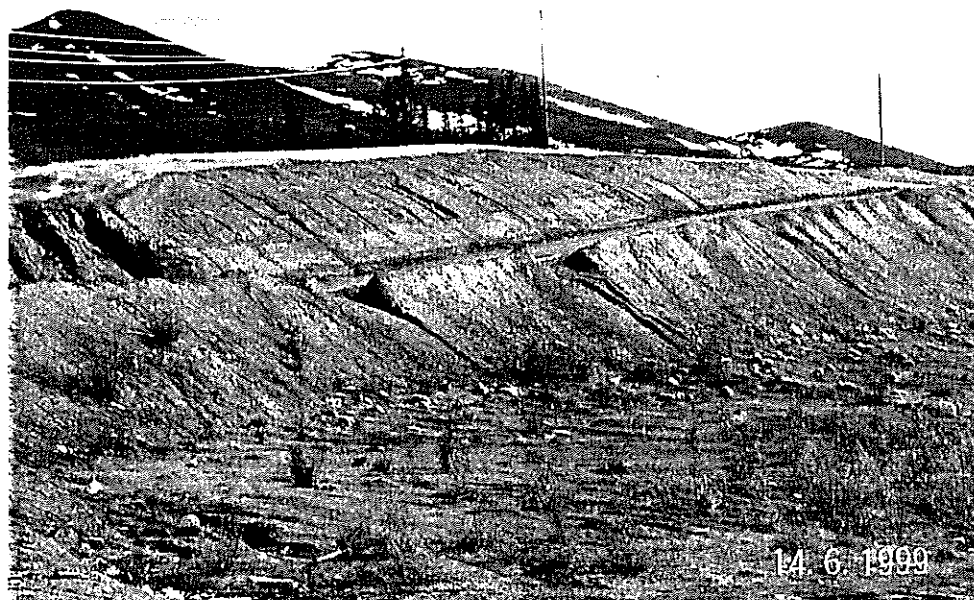
Photo 13: Erosion Gullies in Approach Road to Little Creek Dam
