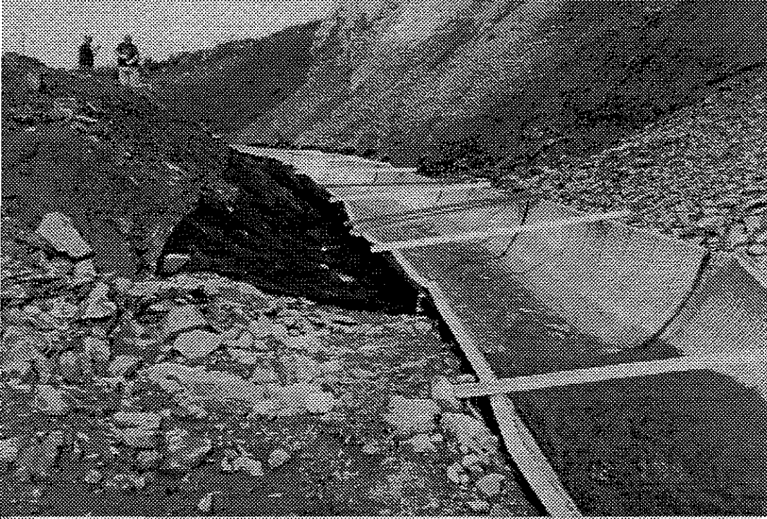
Photo #6a, placement of filter fabric
