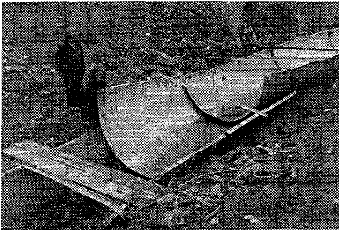
Photo #5b, installation of replacement flume sections
