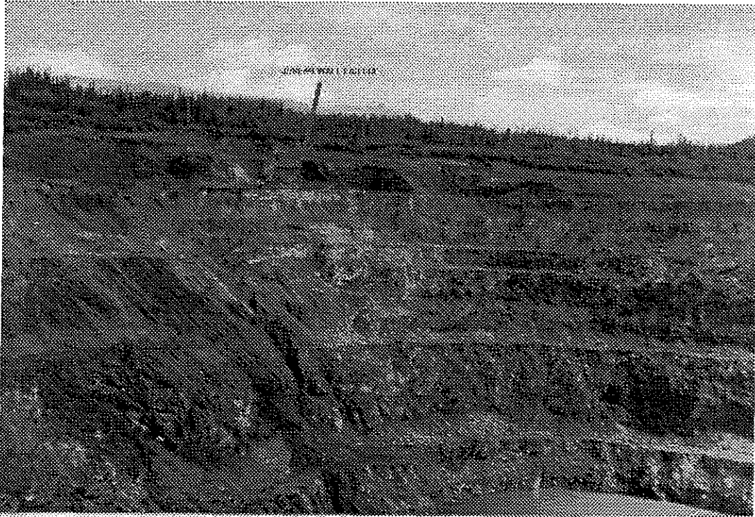
Photo #2, location of work area wrt Vangorda pit
