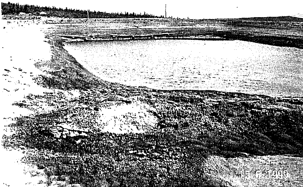
Photo 26: Sludge Pond at the Treatment Plant
