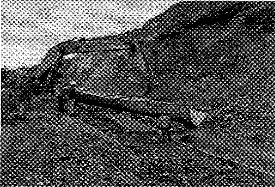
Photo #5a, installation of replacement flume sections
