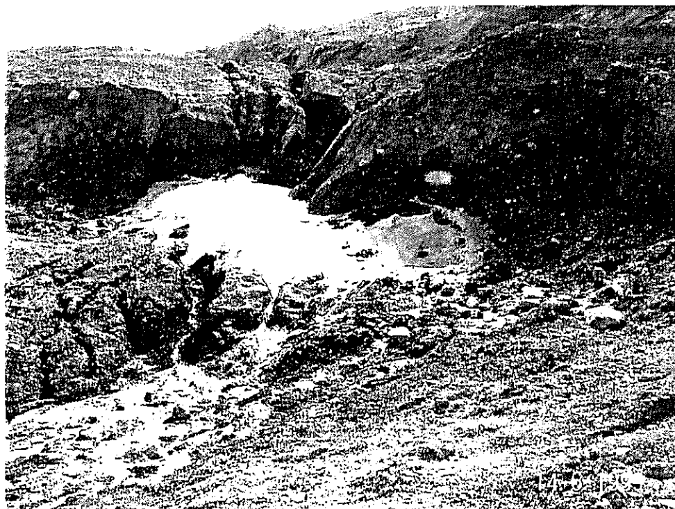
Photo 4: Erosion above Weir 6
