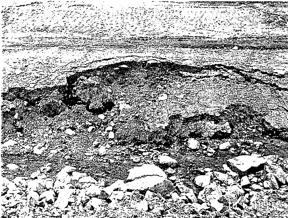
Photo 29: Erosion in GID Sideslopes below Treatment Plant
