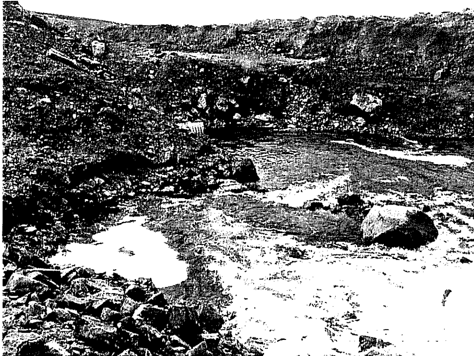
Photo 25: Erosion of the Sideslopes at the Stilling Basin below the Vangorda Creek Diversion
