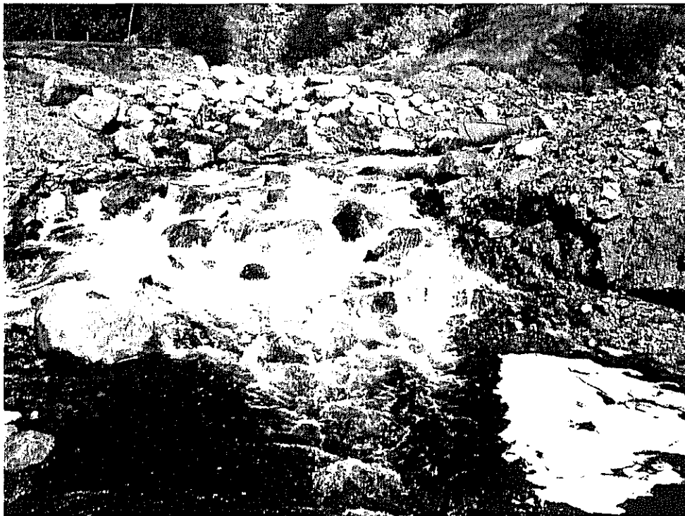
Photo 24: Outlet of the Vangvorda Creek Diversion
