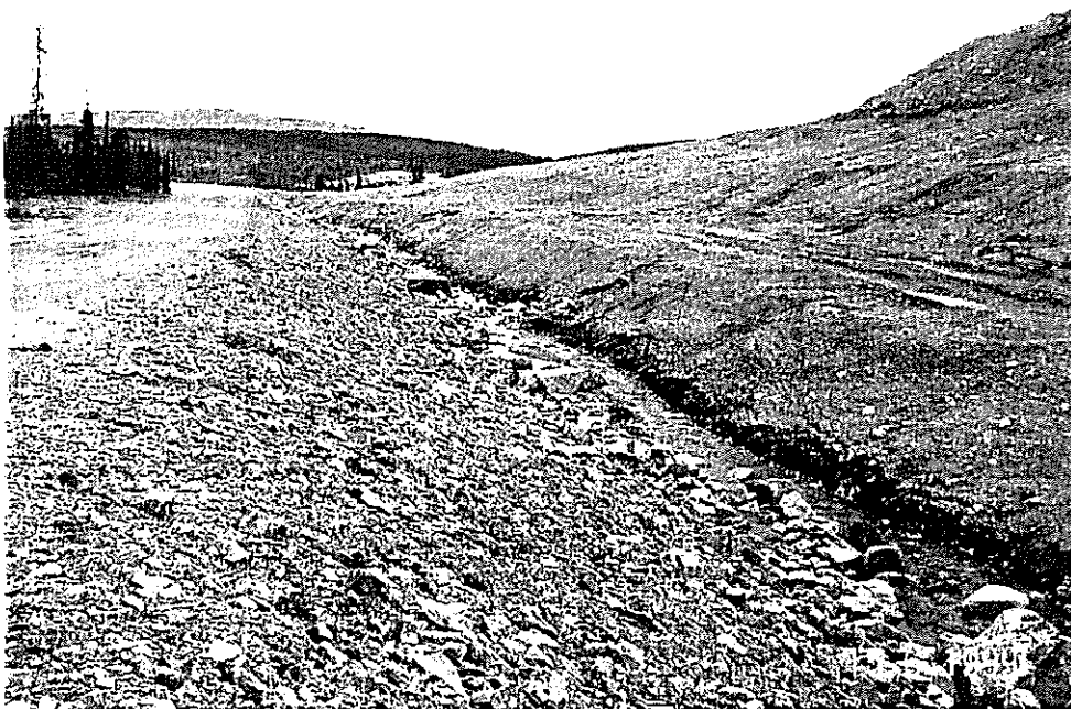
Photo 30: Grum Interceptor Ditch
