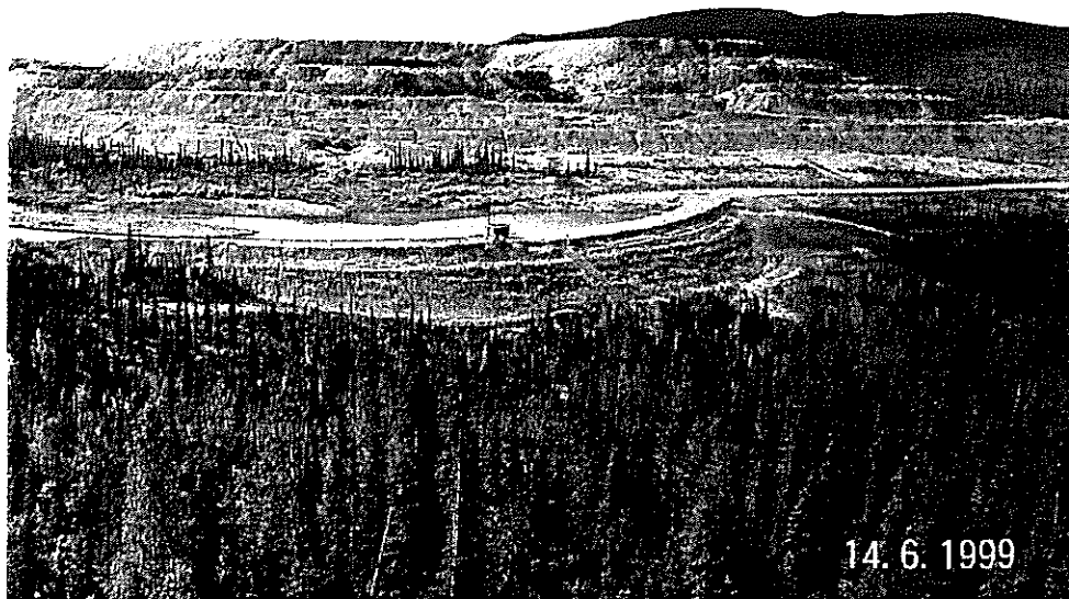
Photo 9: Little Creek Dam
