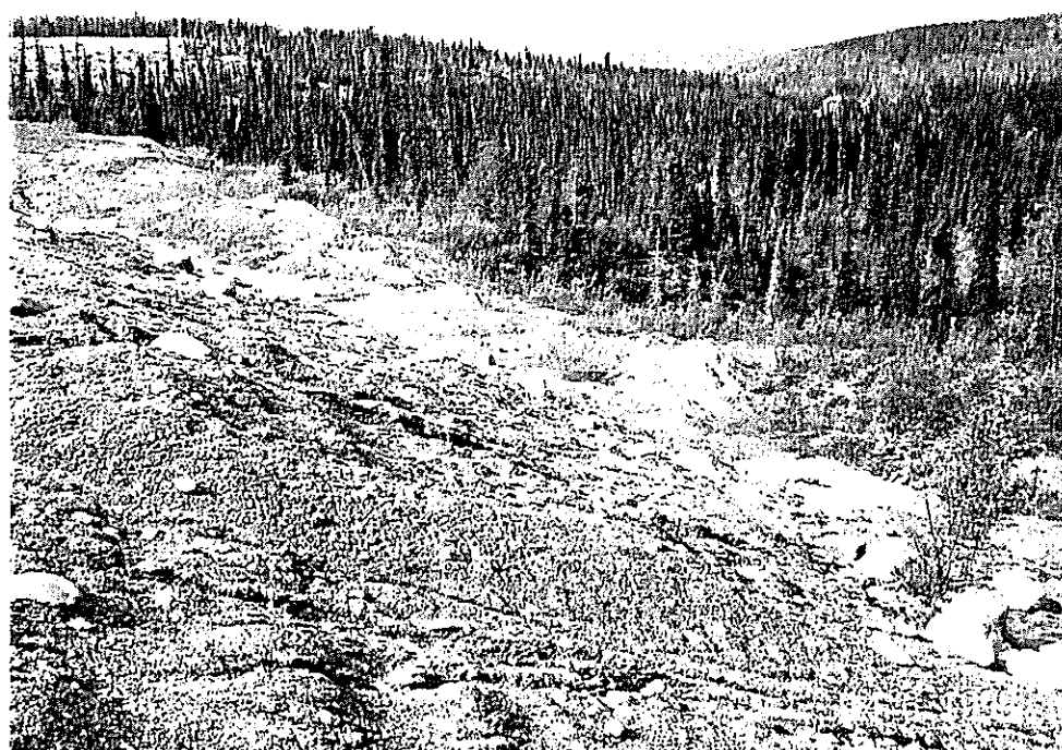
Photo 14: Downstream Face of Little Creek Dam
