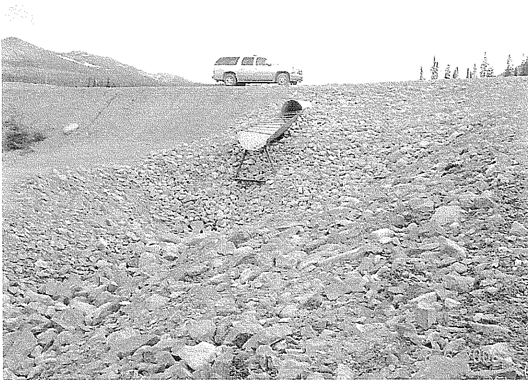
Photo 15 Emergency Spillway Culvert and chute at Little Creek Dam
