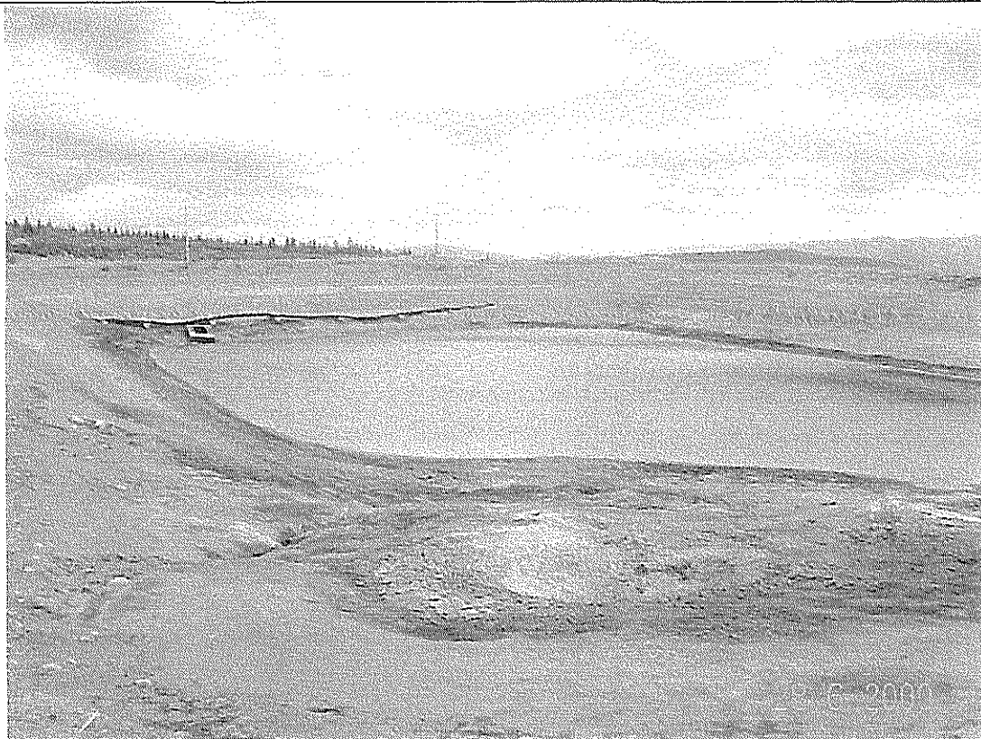
Photo 23 Sludge Pond at the Treatment Plant
