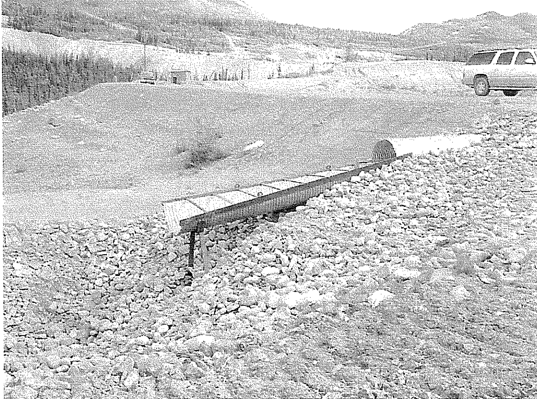
Photo 16 Emergency Spillway at Little Creek dam
