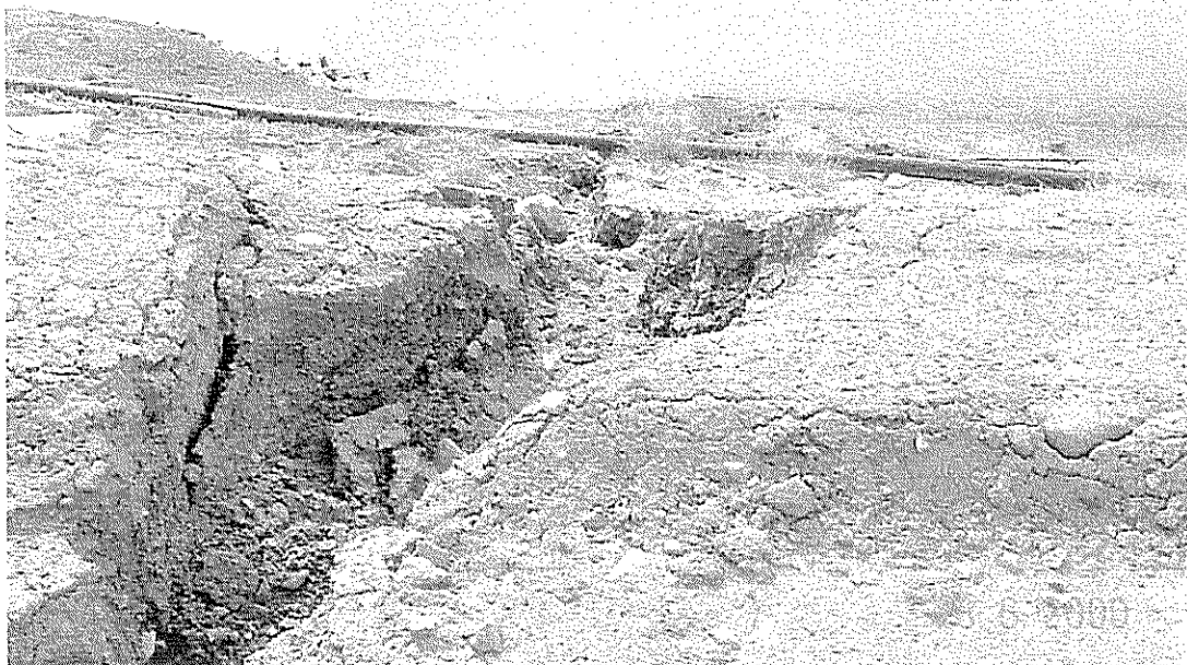
Photo13 Erosion Gully on the upstream face of Little Creek Dam
