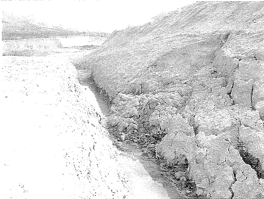
Photo 8 Subsidence in the Diversion ditch
