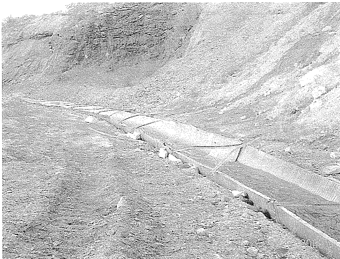
Photo 19 Lower Reaches of Vangorda Creek Diversion
