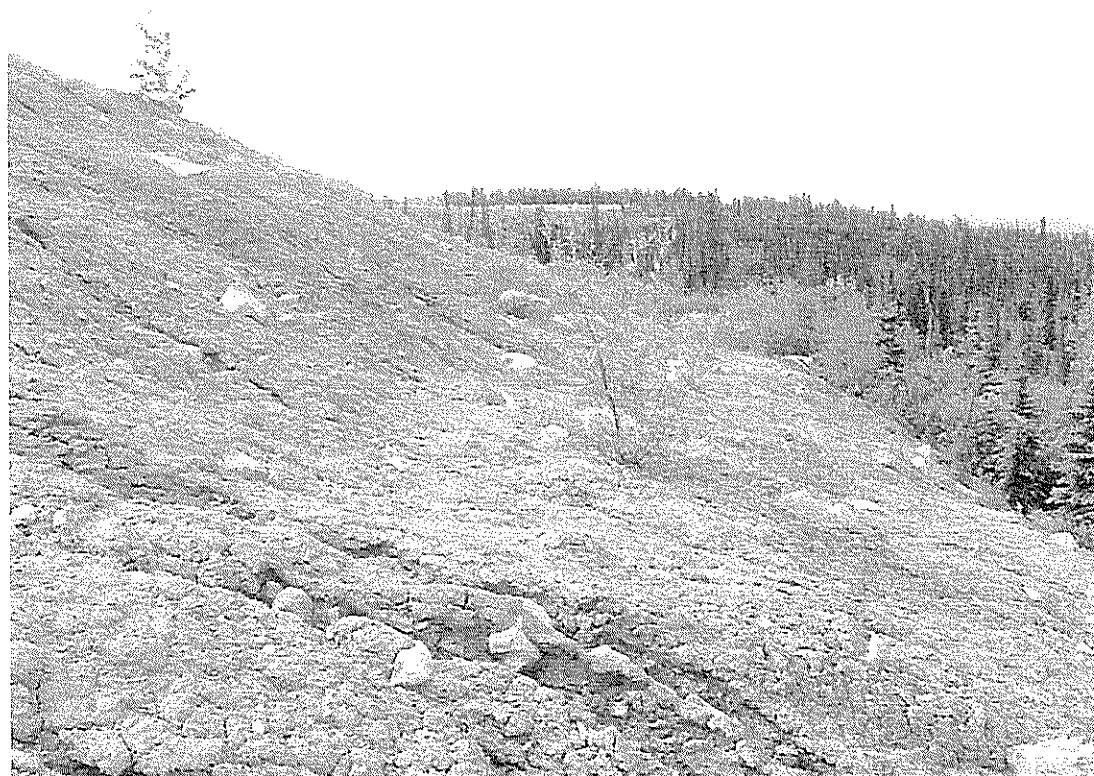
Photo 14 Downstream face of Little Creek Dam
