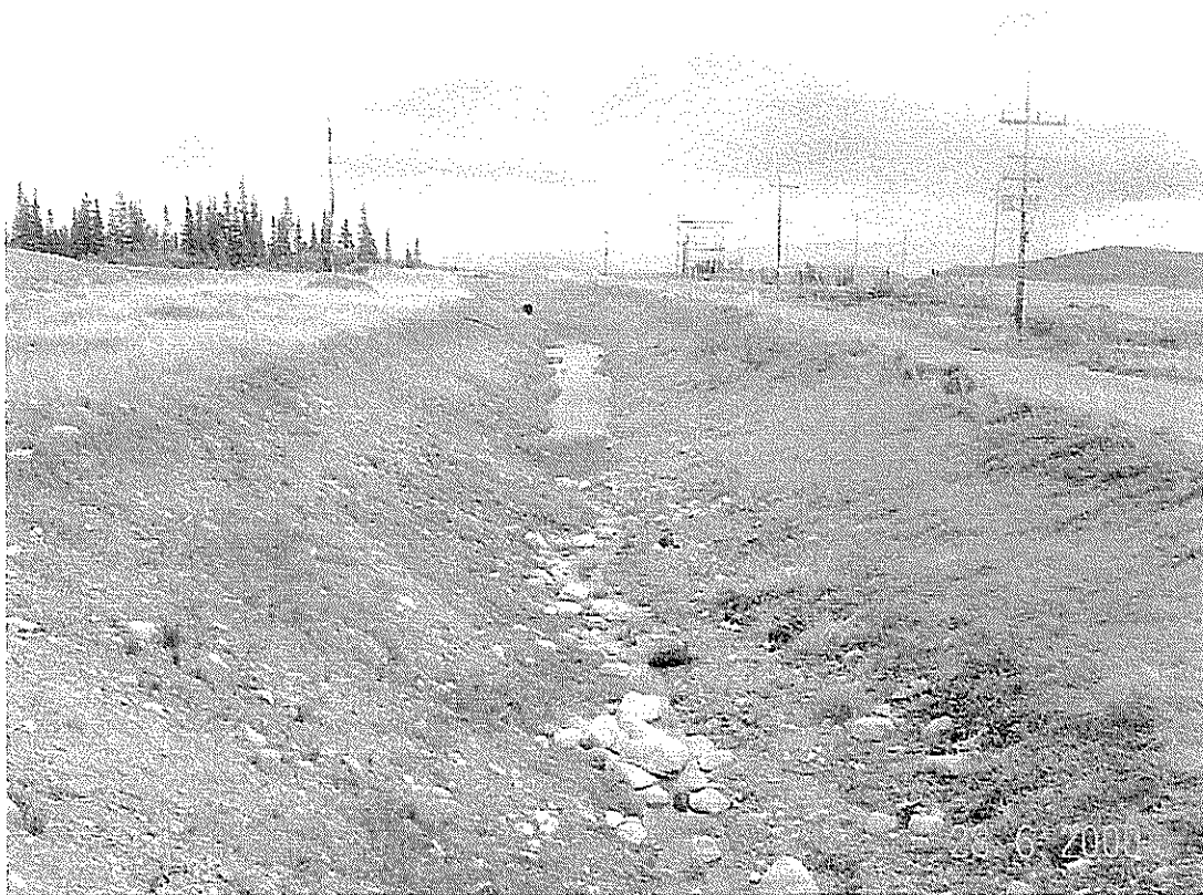
Photo 27 Grum Interceptor Ditch
