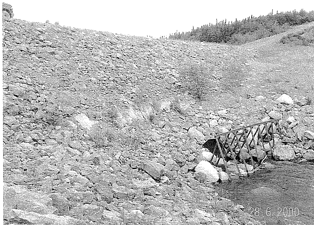
Photo 20 Headworks of the Vangorda Creek Diversion
