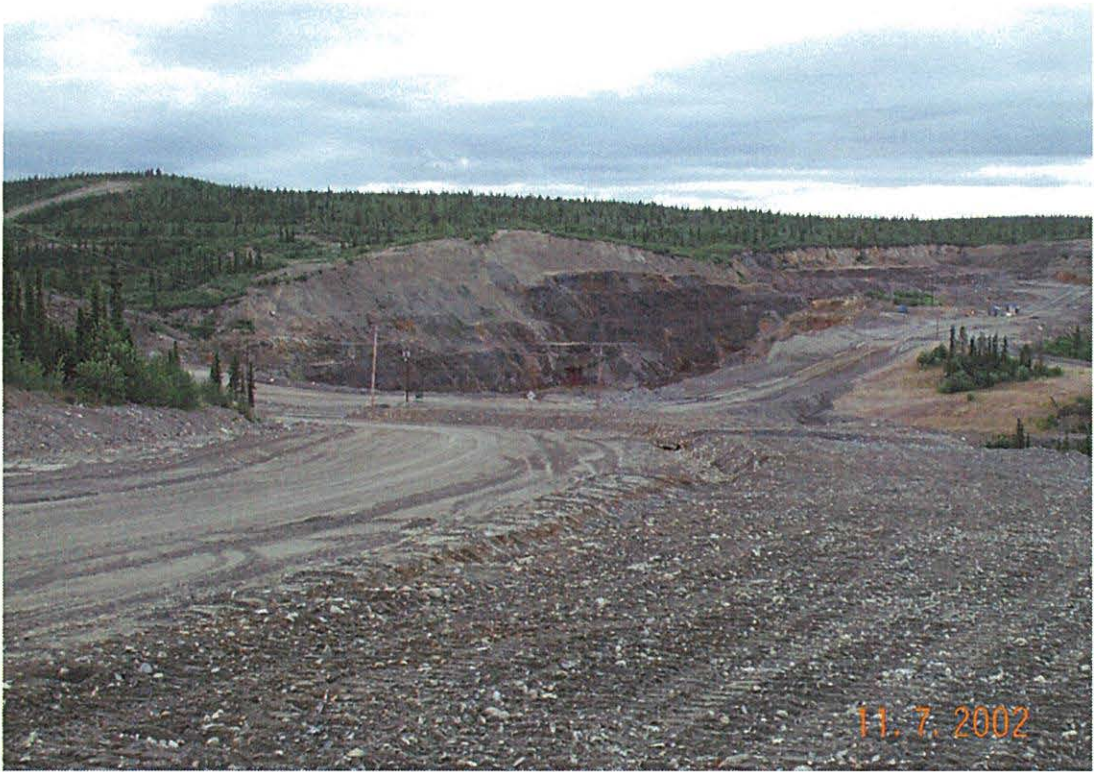
Photo 29: New water collection ditch along haul road
