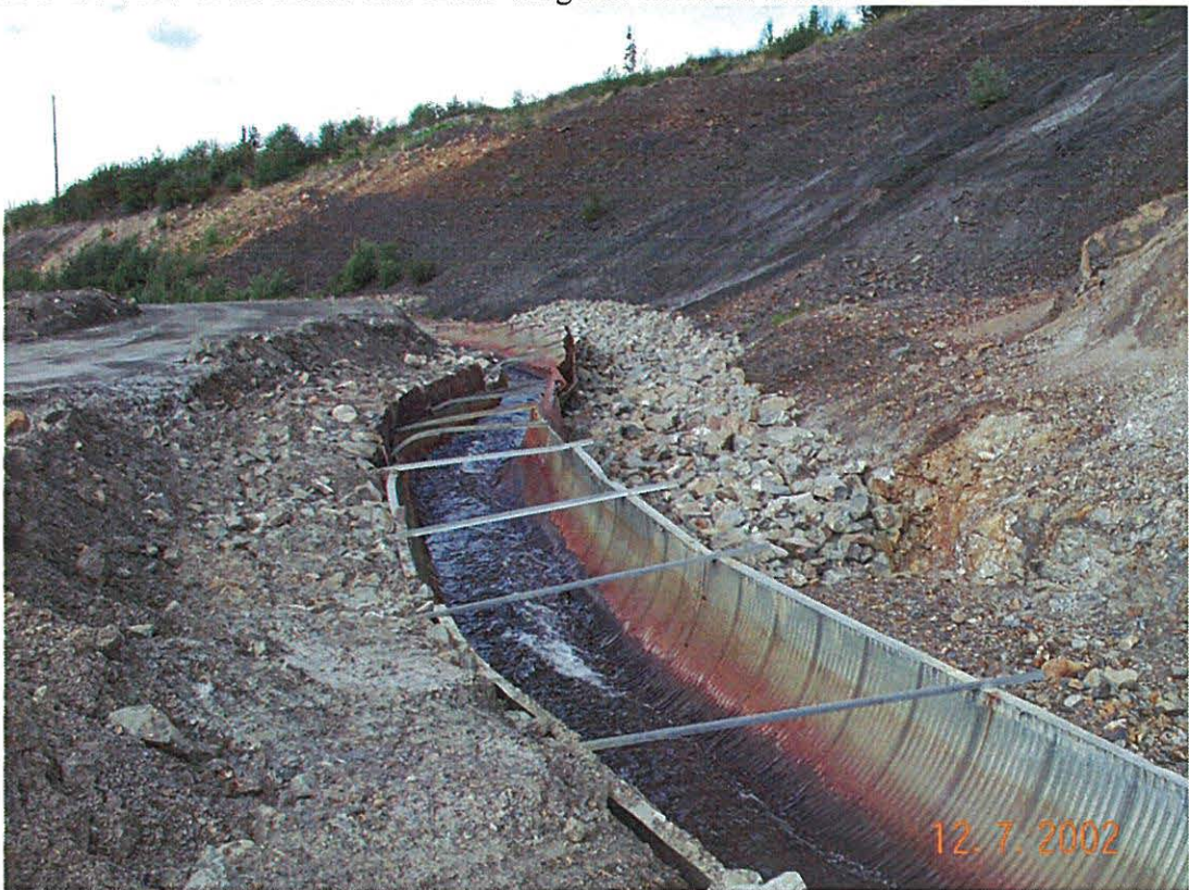
Photo 20: Middle reaches of the Vangorda Creek Diversion
