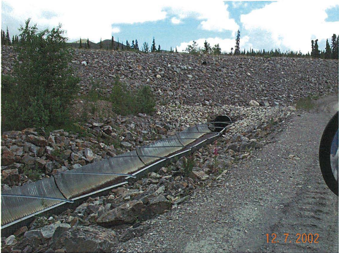
Photo 19: View of the headworks of the Vangorda Creek diversion
