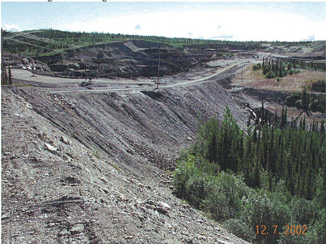
Photo 22: Outfall from the Drop Box Structure with the Vangorda Pit in the background.
