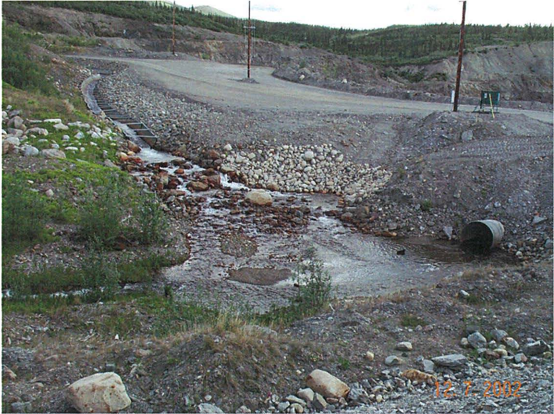
Photo 21: Plunge Pool on Vangorda Creek Diversion
