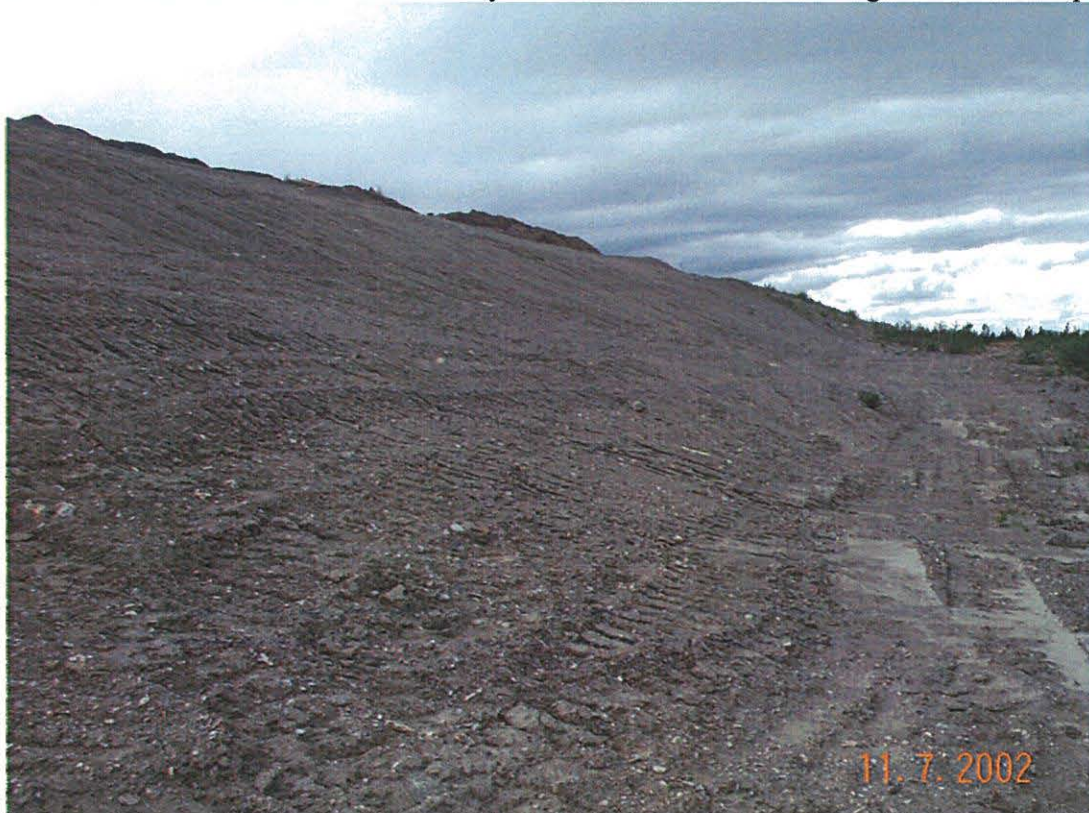
Photo 4: Resloped areas of the Starter Dyke
