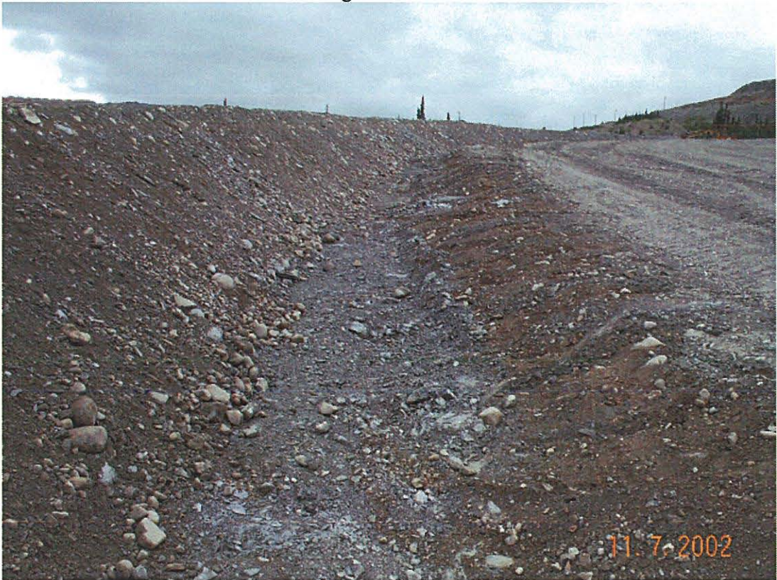
Photo 30: Collection Ditch along the Haul Road at Vangorda
