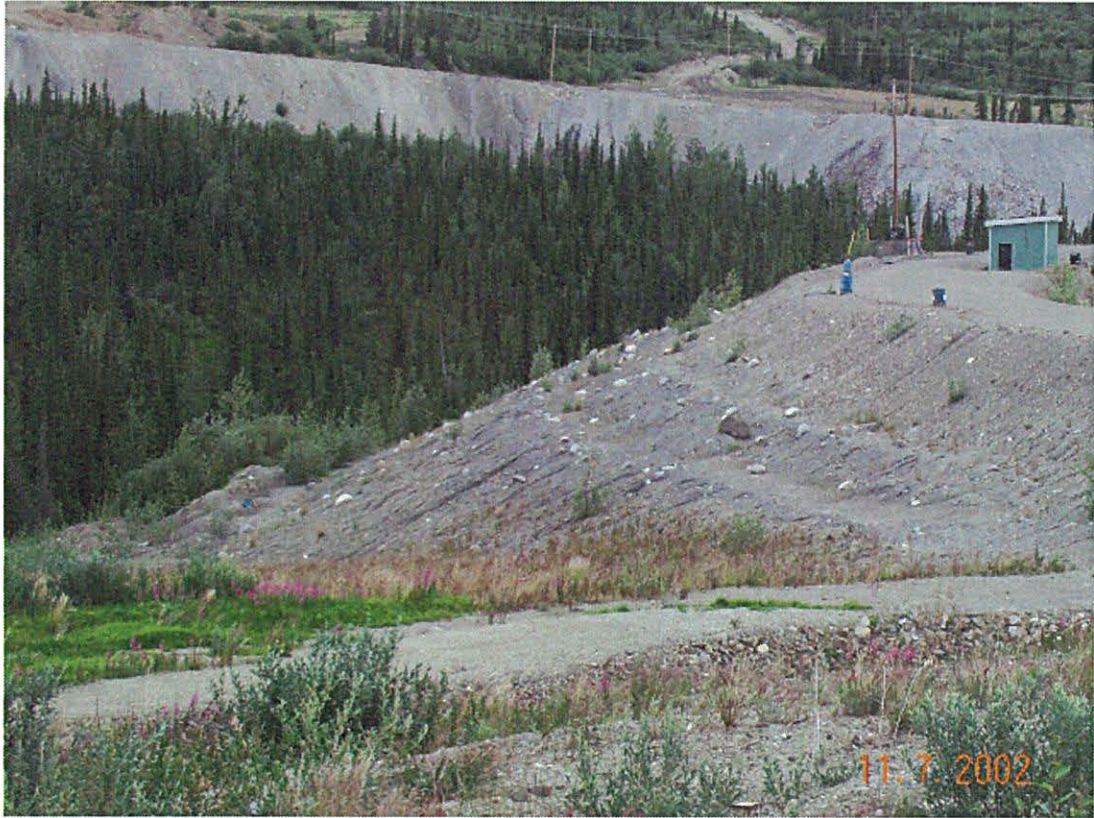
Photo 15: Downstream slope of Little Creek Dam
