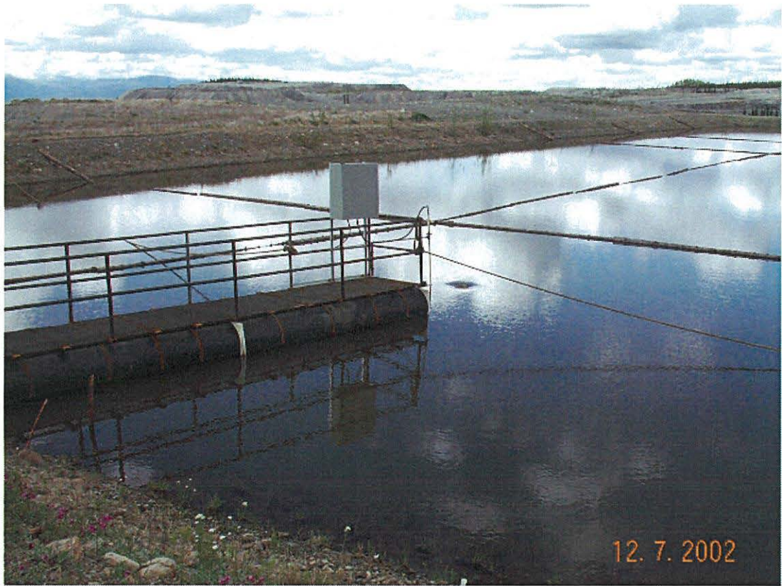
Photo 23: Walkway and intake pipe at the Water Treatment Plant Sludge Pond
