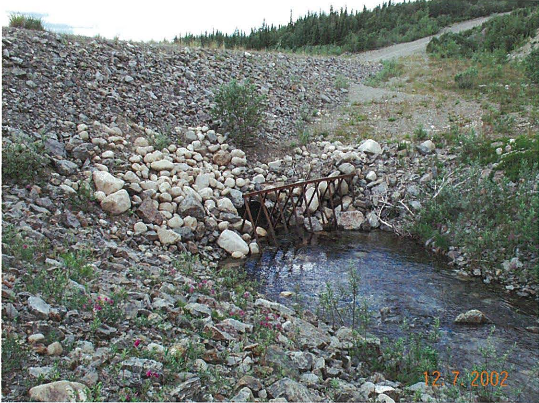
Photo 17: Trash rack at headwaters of the Vangorda Creek Diversion.
