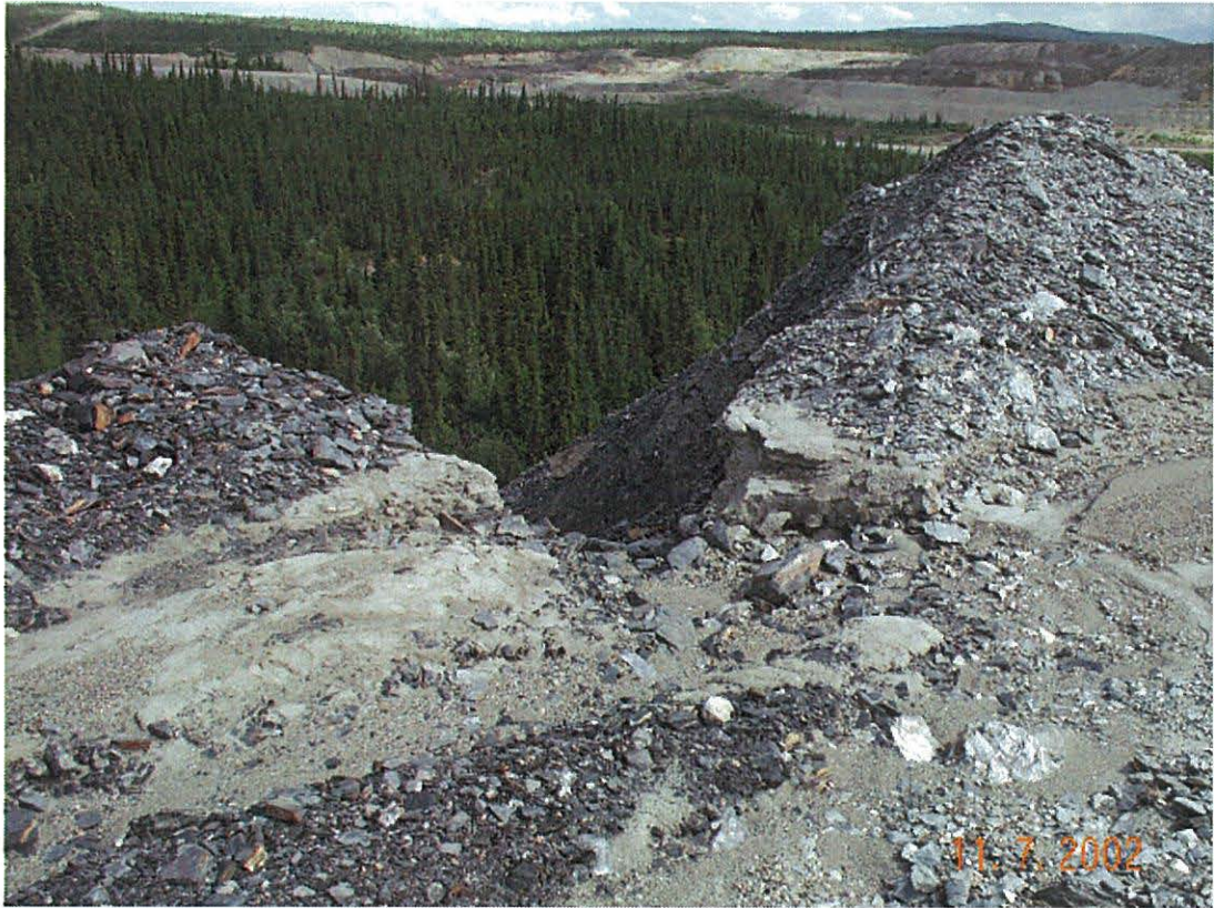
Photo 27: Erosion gully in lower bench of the Grum waste dump above Seep #1
