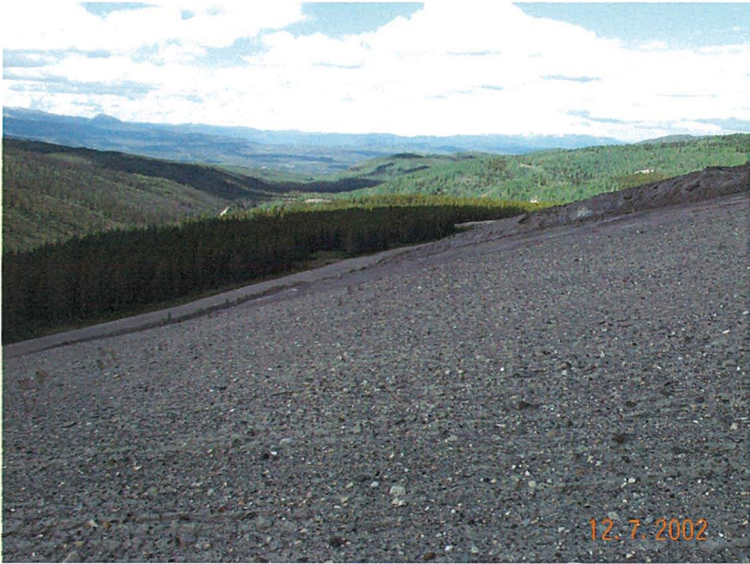
Photo 13: Till cover over waste rock on the resloped section of the Vangorda Waste dump
