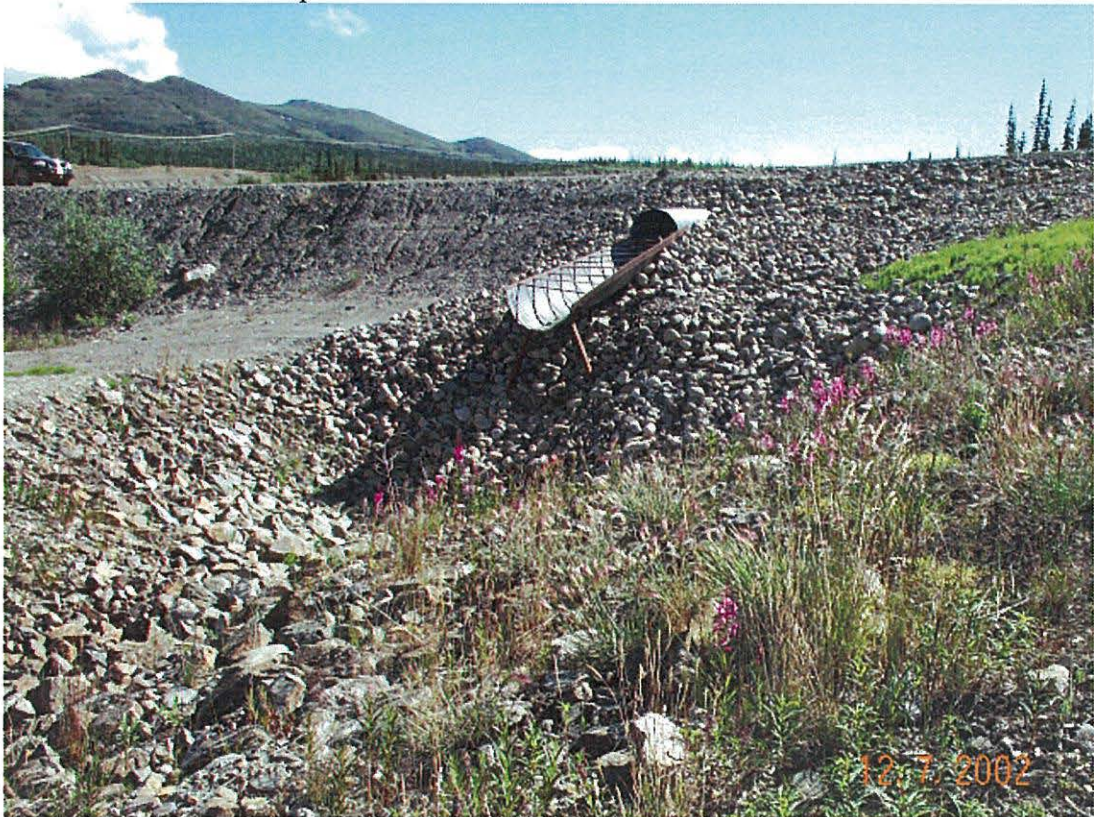
Photo 16: Emergency Spillway at Little Creek Dam
