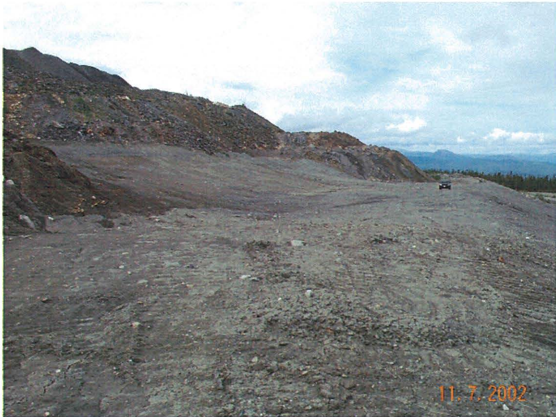
Photo 3: Recontoured section of the Till dyke on the north side of the Vangorda waste Dump
