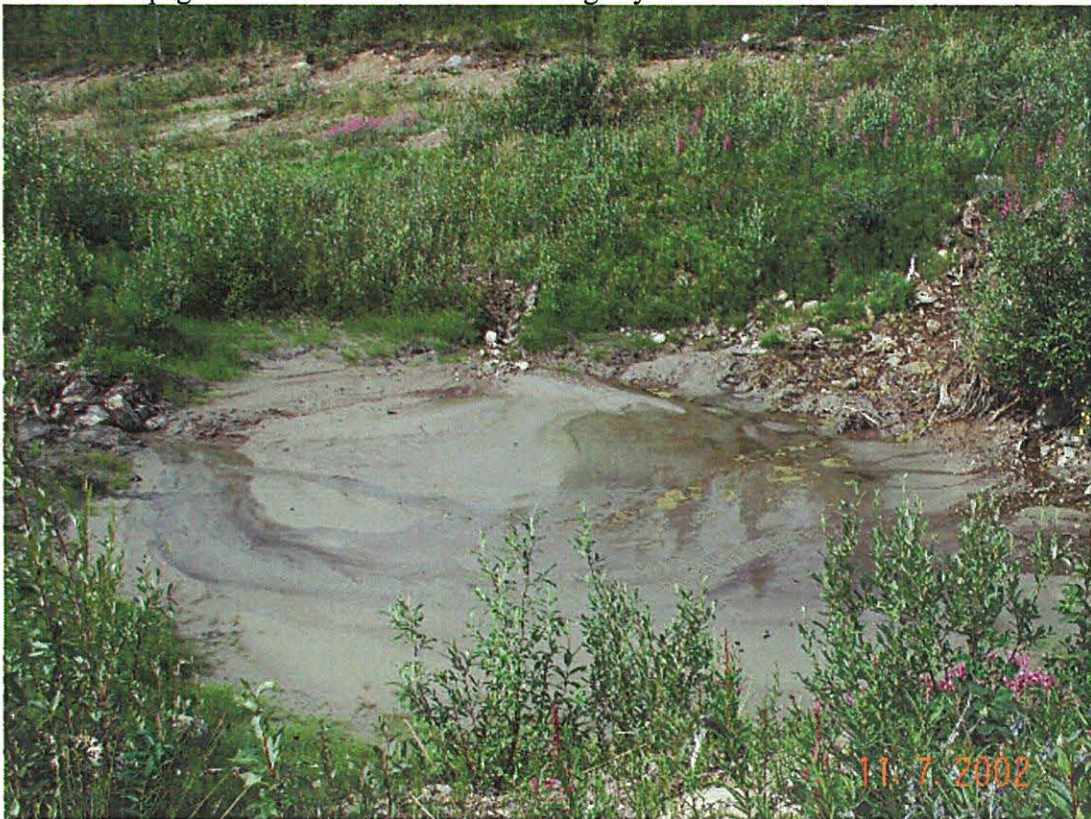
Photo 26: Sediment basin at the toe of the Grum Dump
