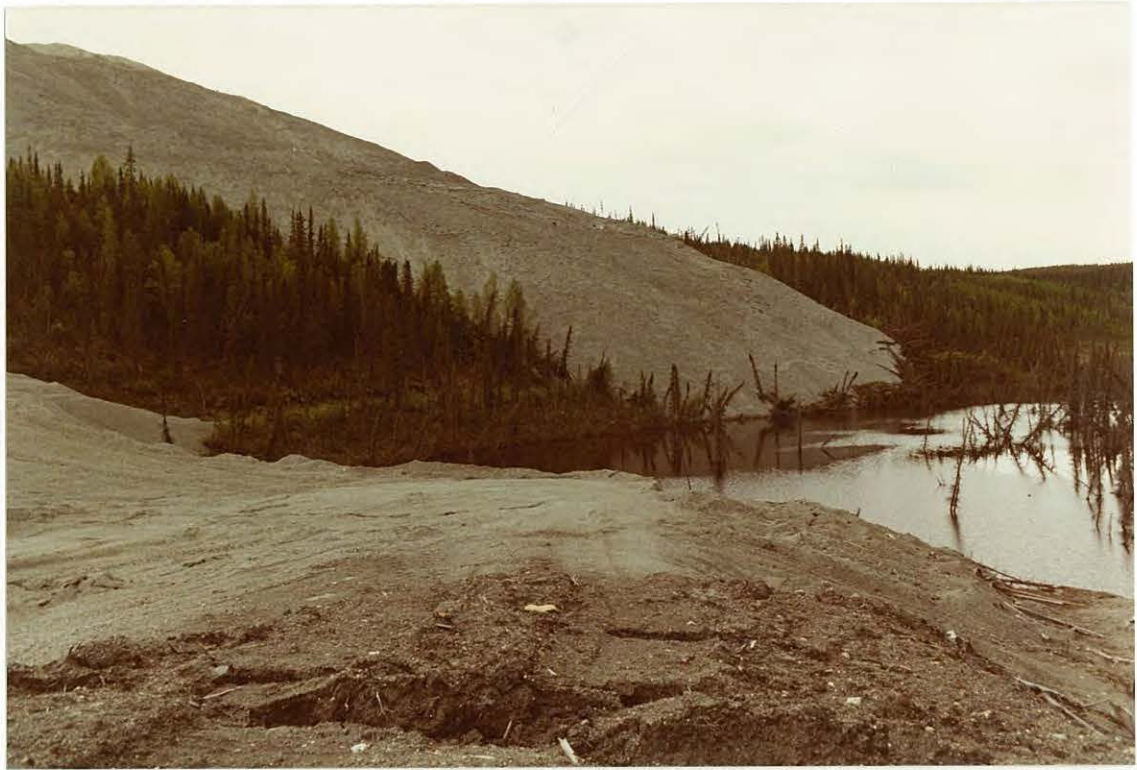
Photo 7: Toe of north tailings lobe extending into lake. June 14, 1984.
