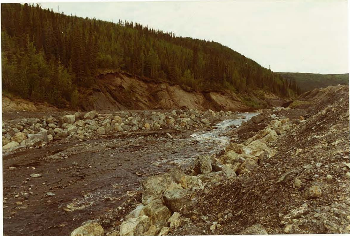
Photo 1: Upstream end of Clinton Creek channel, looking downstream. Note narrow channel opposite bank protection section construction in 1983. June 14, 1984.
