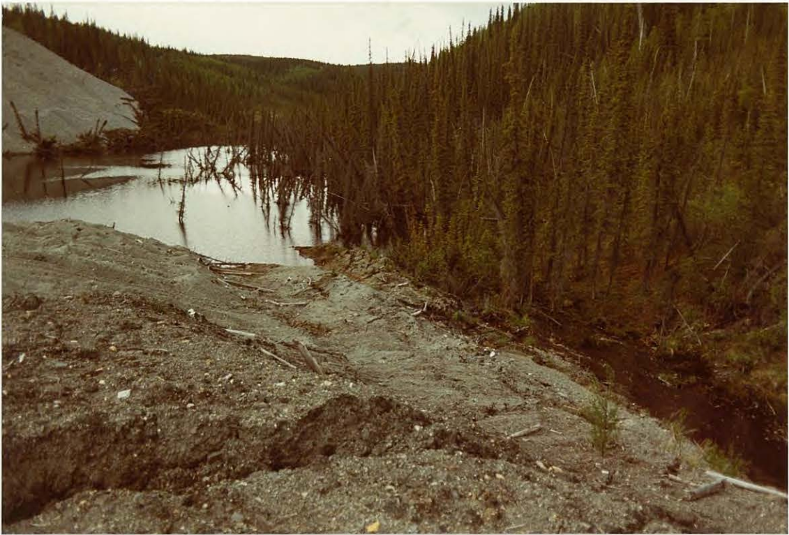
Photo 5: Wolverine Creek at outlet of lake formed by south tailings lobe. Note channel squeezing and upthrust foundation material from tailings pile movements. June 14, 1984.
