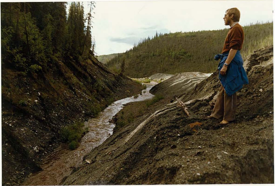
PHOTO 5: Channel at toe of south lobe of tailings pile with inlet to lined channel in distance.
