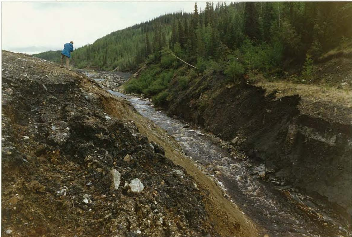
PHOTO 2: Waste Dump channel looking upstream. Erosion protection works in distance.
