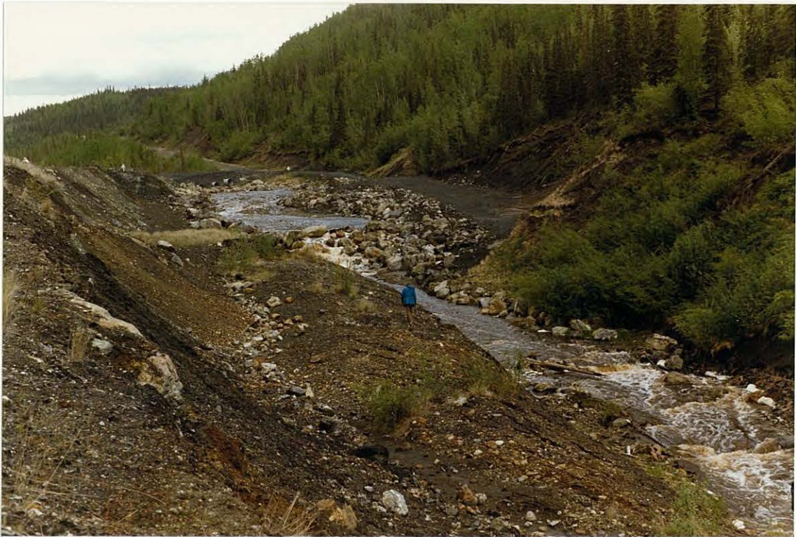
PHOTO 1: Waste Dump channel inlet area looking upstream to channel protection works and inlet culverts.
