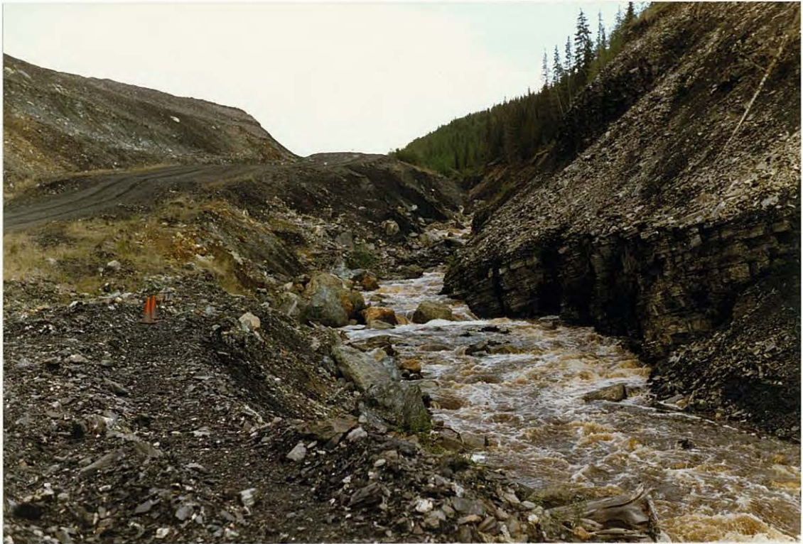
PHOTO 3: Waste Dump channel further downstream.
