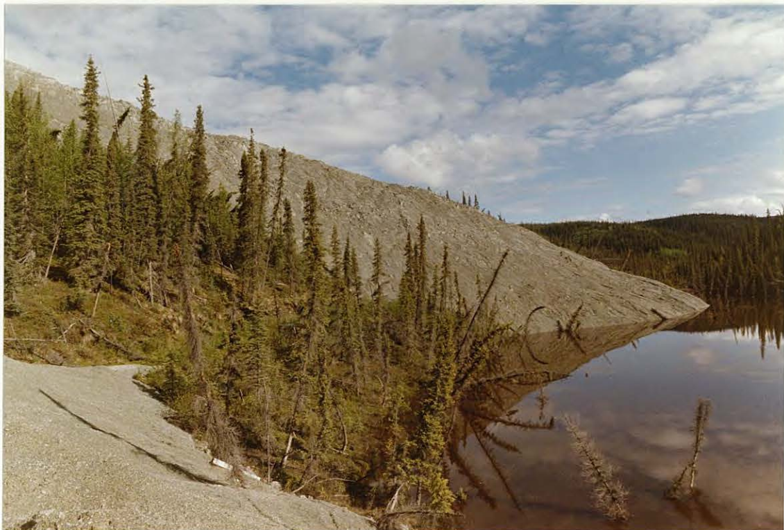
PHOTO 4: North lobe of tailing pile at toe of slope. Toe is now well into lake and slope is flattening.
