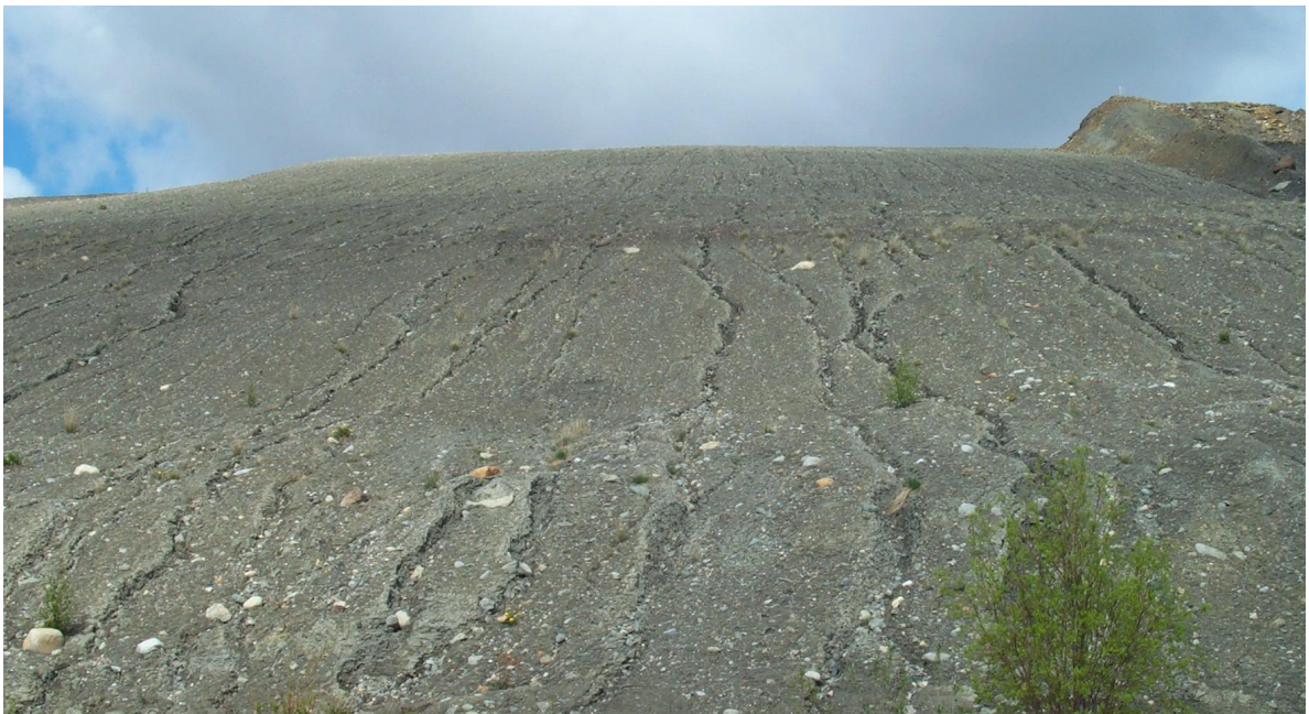
Photo 3: View of the 10 year old till cover on the Vangorda waste rock pile as seen from the base of the pile.
