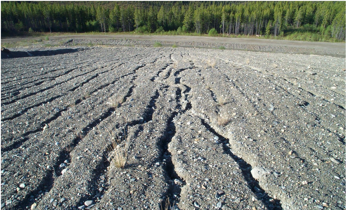
Photo 2: Erosion gullies on the 10 year old till cover on the Vangorda waste rock pile, as seen from the crest of the pile.
