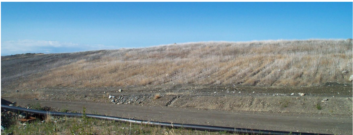
Photo 7: View of re-sloped and re-vegetated slope on the Overburden dump. Note the abrupt edge of the vegetation, confirming that without active seeding, natural re-vegetation potential is low.
