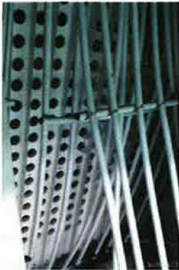
Figure 4 Interior misting system for old grow unit.
