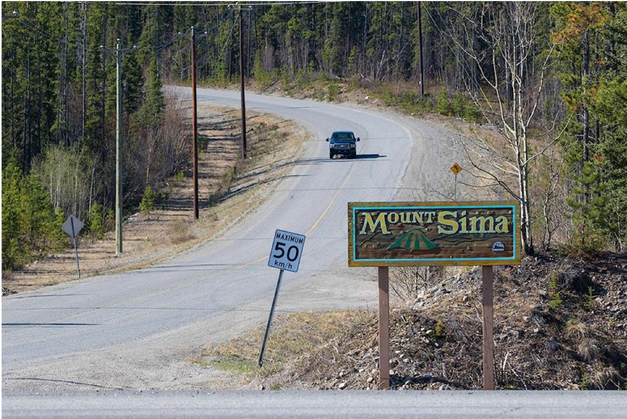
FIGURE 8: EXAMPLE OF RURAL INDUSTRIAL ROAD AT THE ENTRANCE TO MOUNT SIMA SUBDIVISION (YUKON NEWS, 2020)
