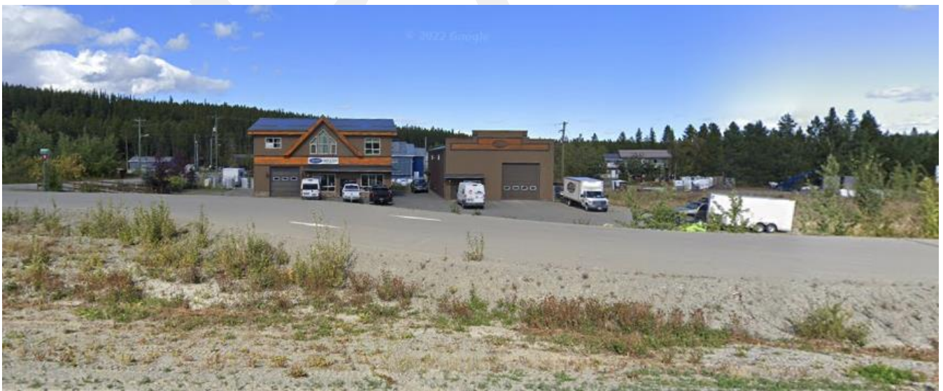
FIGURE 9: EXAMPLE OF HIGHWAY COMMERCIAL DEVELOPMENT (METROPOLIT LANE) (GOOGLE, 2022)
