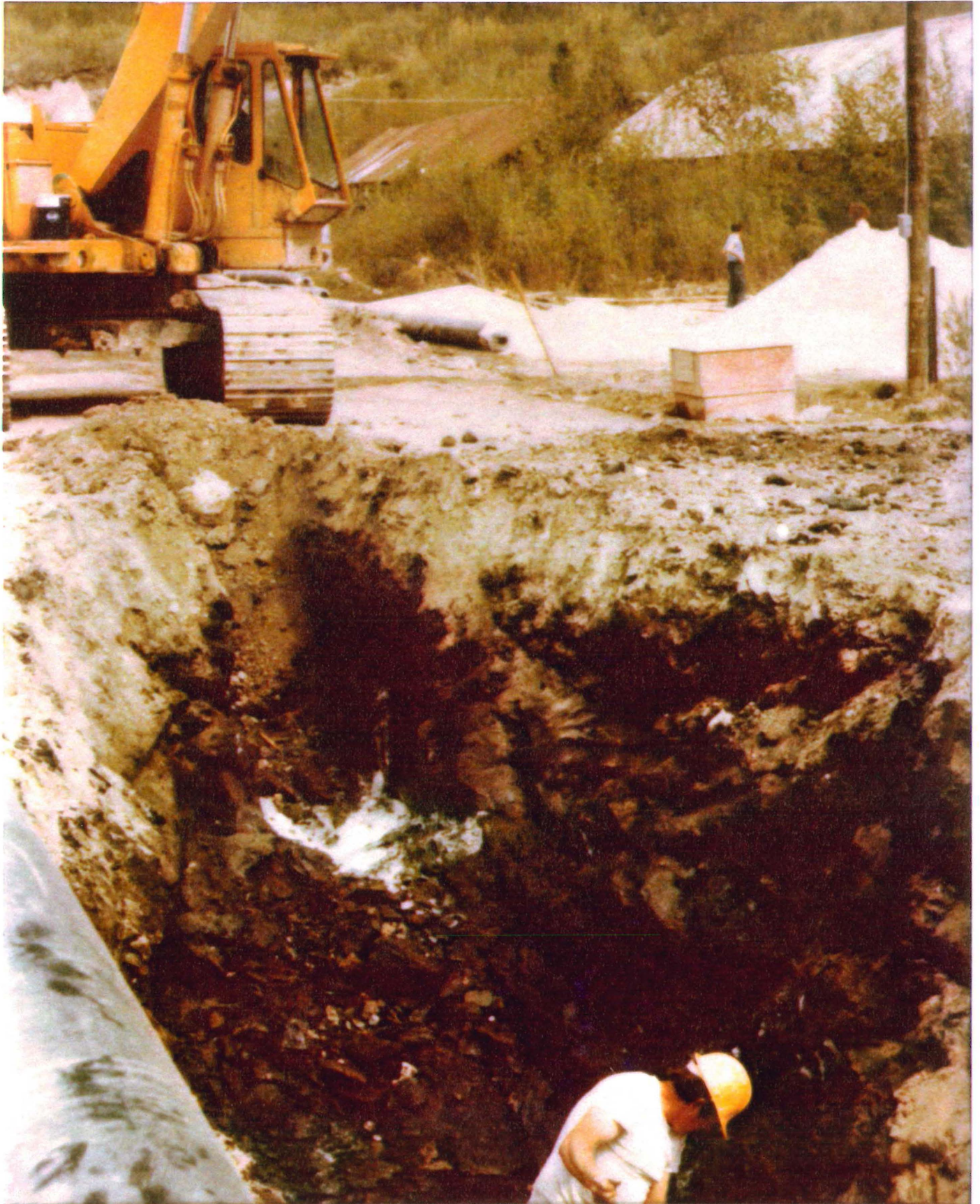
EXCAVATION IN PERMAFROST – Dawson City
