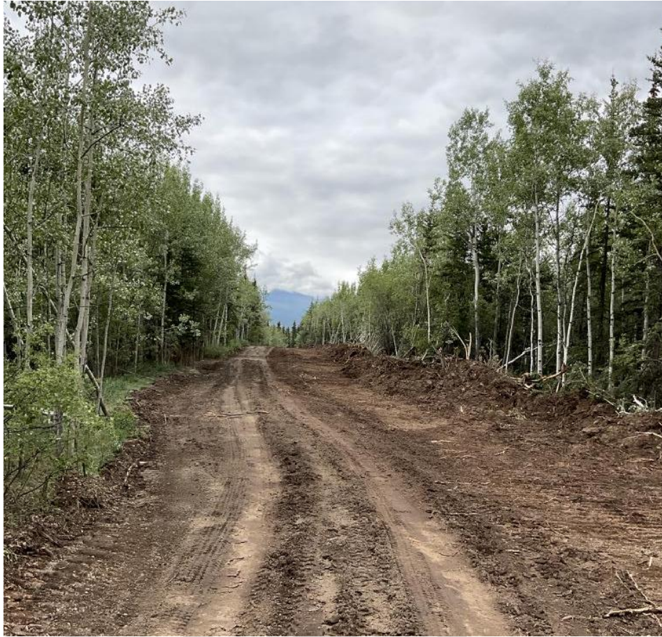
Figure 10: Example of a fire guard constructed during a wildfire response in Southern Yukon. Preventative fire guards have the benefit of time to construct in a clean, tidy manner and considering community values versus fire guards constructed in haste of an emergency situation.
