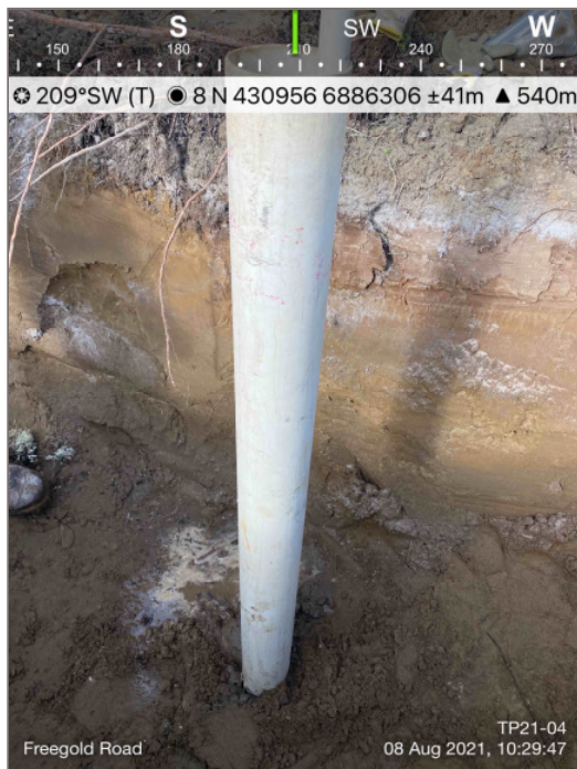
Photo 3: Freegold Road Area – Testpit 4 (TP21-04) percolation rates testing.
