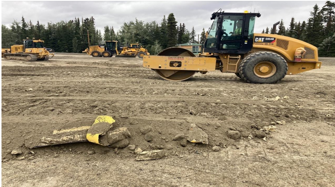
On-Going Site Grading and Debris Removal
