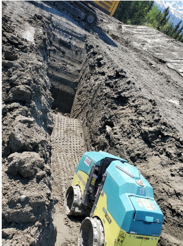
Photo 1: Ammann 1575 Robotic Trench Packer in TP03
