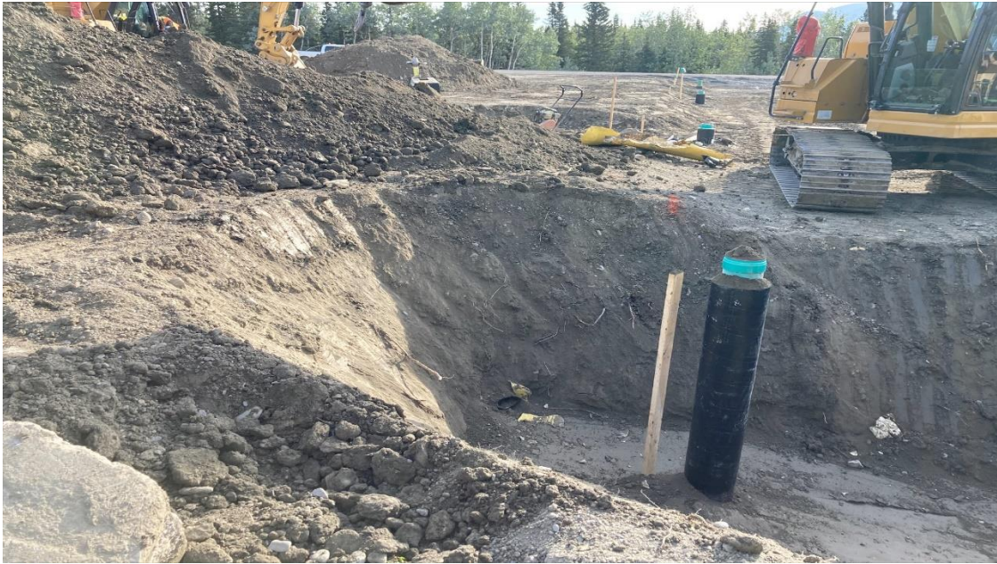
Services Being Installed
