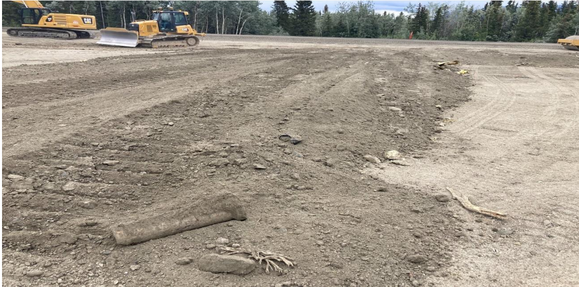
Lot Fill and Debris Removed From Lift
