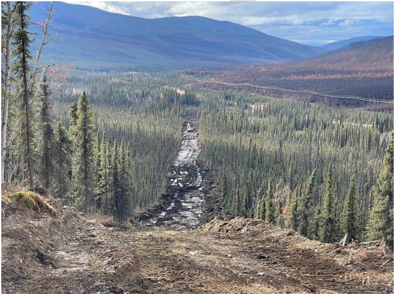
Figure 3: Example of a fire guard constructed during a wildfire response to MA011 near the Victoria Gold Mine Site. Preventative fire guards have the benefit of time to construct in a clean, tidy manner and considering community values versus fire guards constructed in haste in an emergency.
