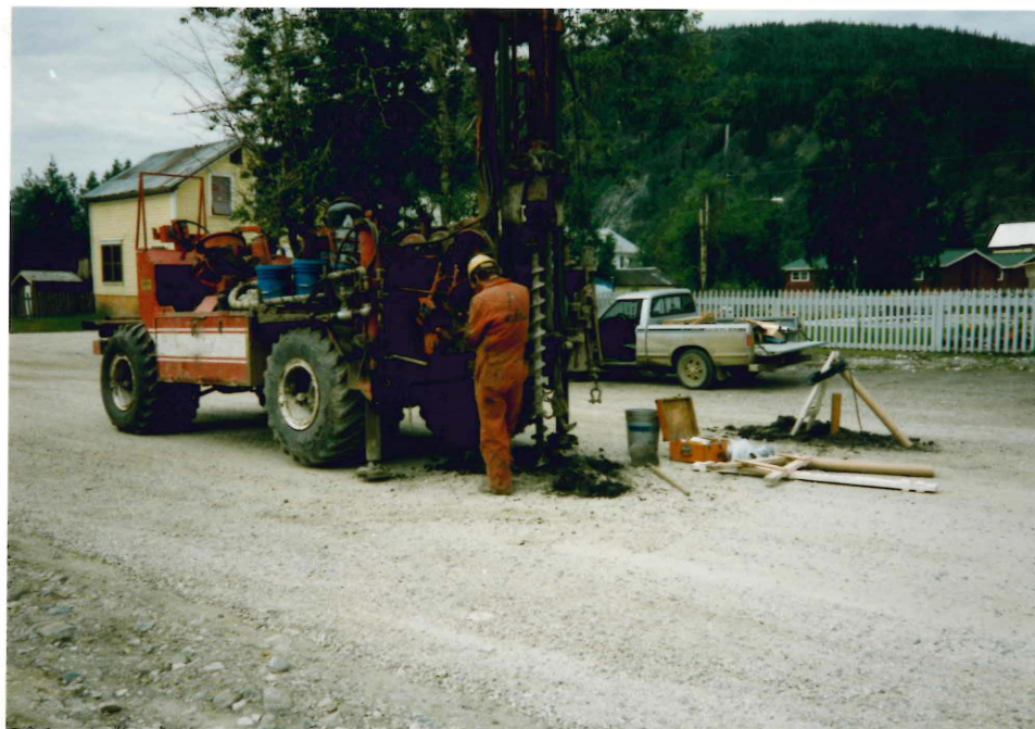
PLATE 1: Installing vertical thermistor cables on 4th Avenue near Church Street (1985-07-04).
