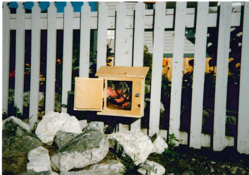
PLATE 6 : Read-out box containing thermistor cable plugs (4th Avenue near Church St., 1985-07-06).
