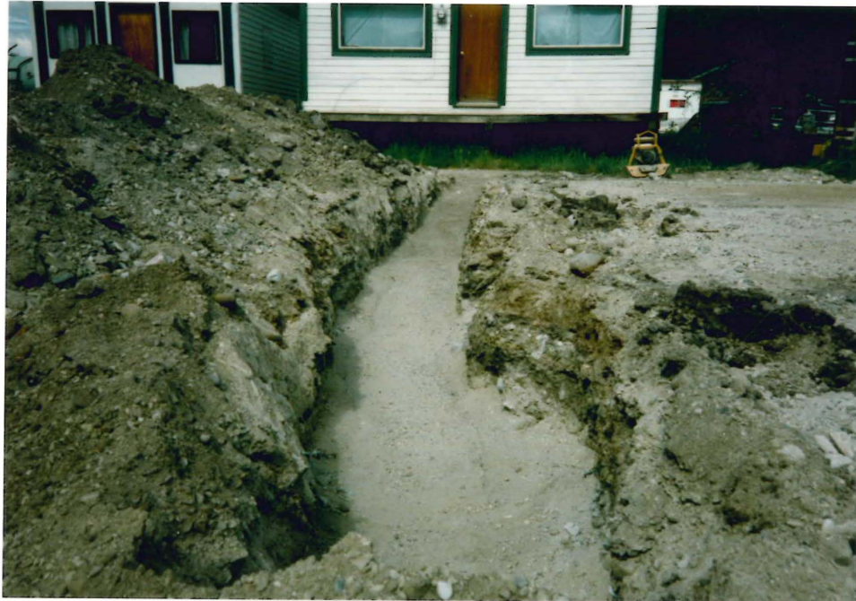
PLATE 5 : First lift of crushed gravel compacted over thermistor cables (Church St., 1985-07-05)
