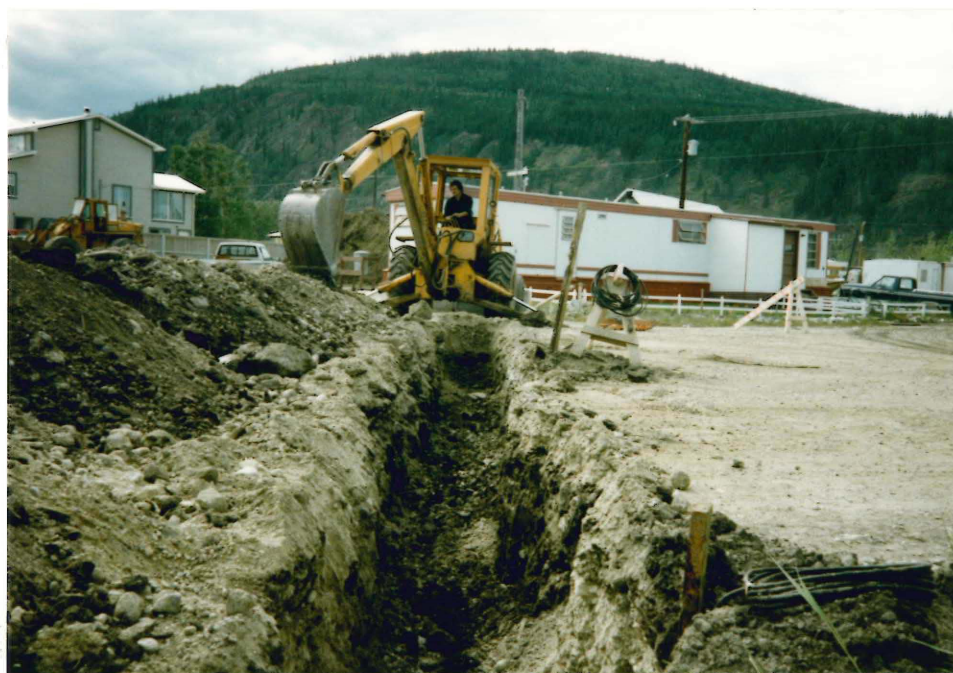
PLATE 1: Installing vertical thermistor cables on 4th Avenue near Church Street (1985-07-04).
