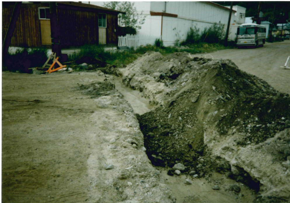
PLATE 4 : Partially backfilled trench showing compacted lifts (4th Avenue and Harper St., 1985-07-05).
