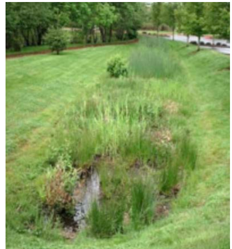
Vegetated dry stormwater pond
