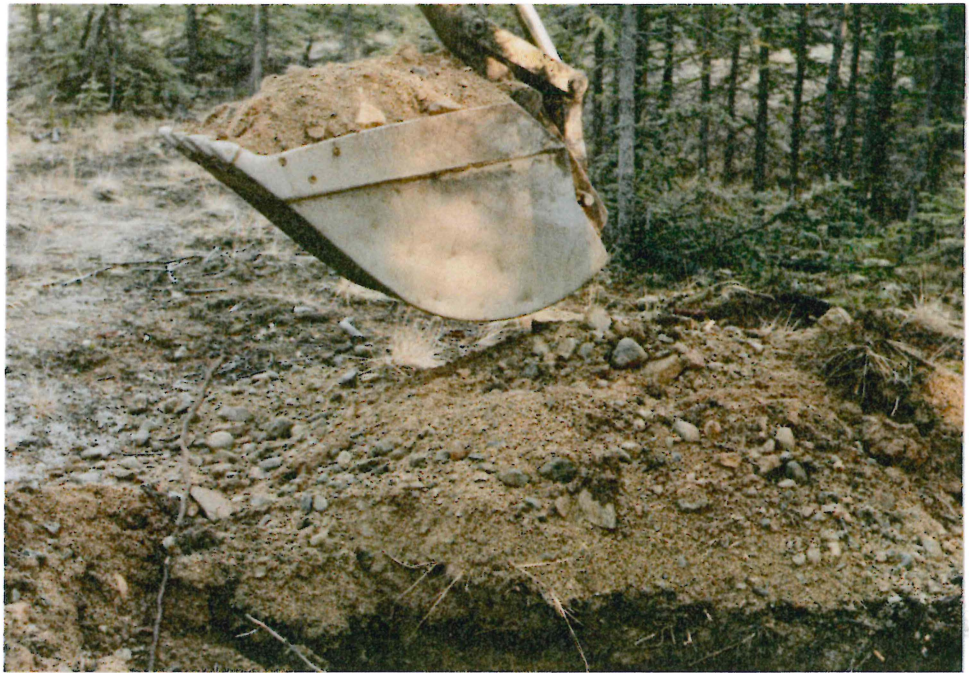
#1-7 TP86-3 EXCAVATED SOIL TO 1.0 m - GRAVEL
