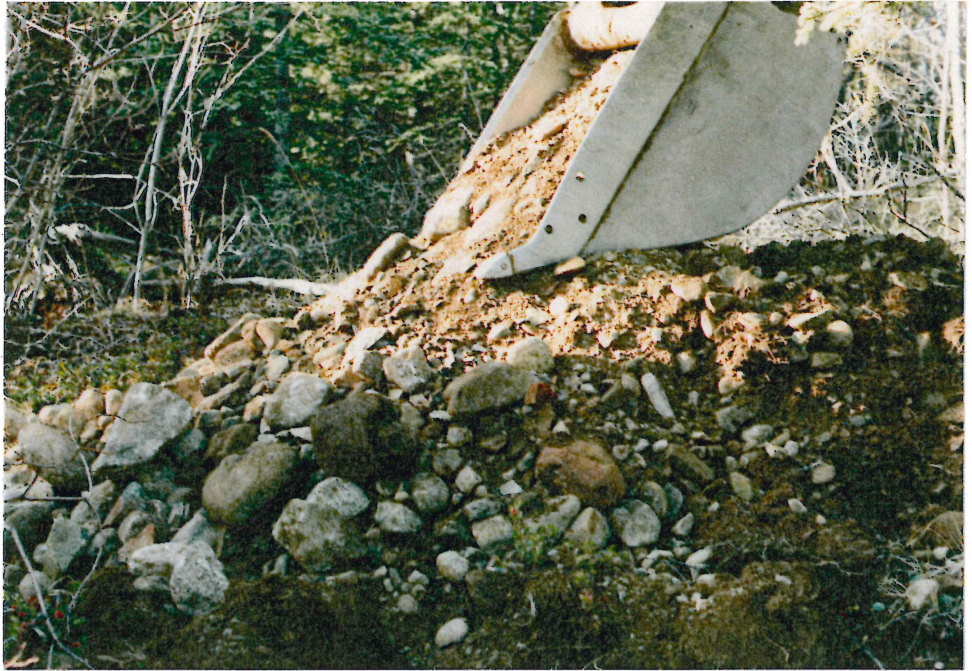
#2-0 TP 86-13 EXCAVATED GRAVELS
