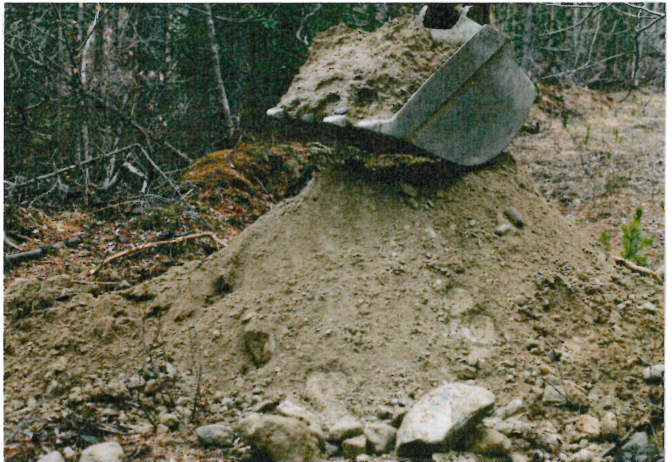
#3-12 TP86-20 EXCAVATED SOIL INCLUDING LAST BUCKET
