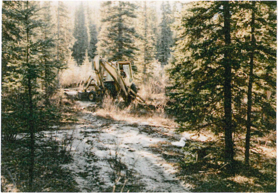
# 1-5 LOOKING WEST DOWN TRAIL TO TP 86-2 (NOTE SWAMPY GROUND BEHIND BACKHOE)
