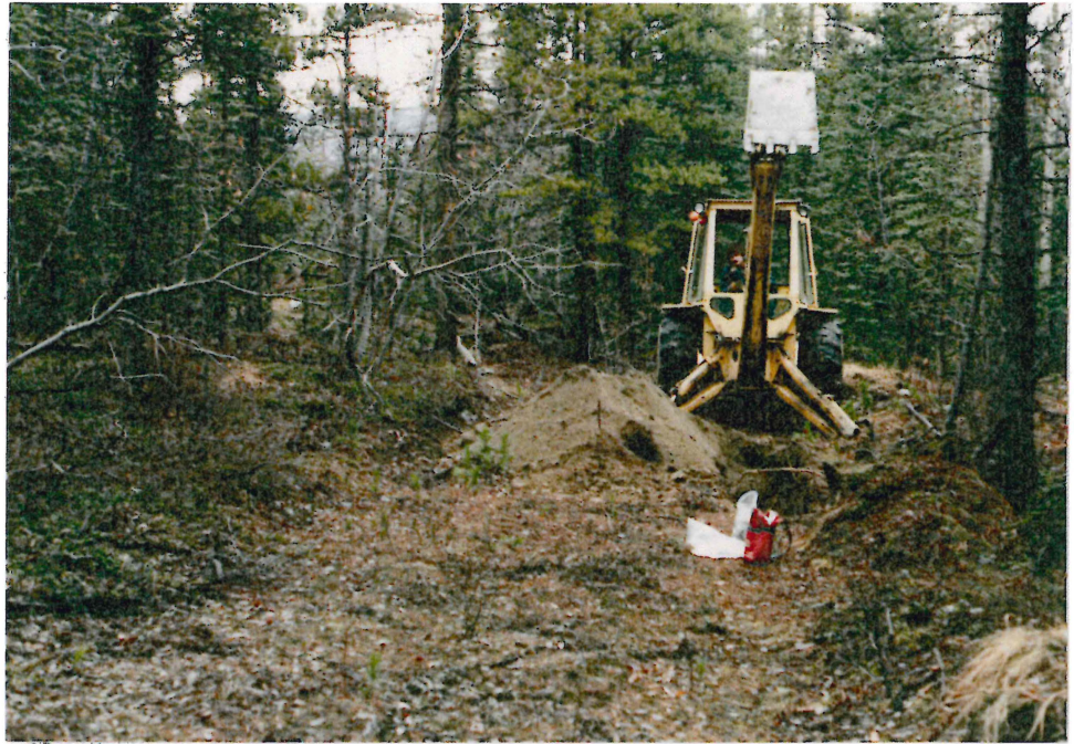
# 3-13 LOOKING NORTH-EAST DOWN ROAD TO TP BG-20
