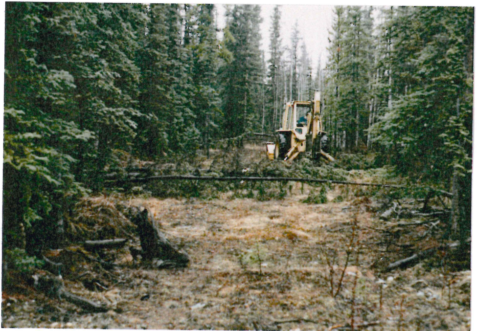
# 3-24 LOOKING NORTH ALONG ROAD TO TP BG-22
