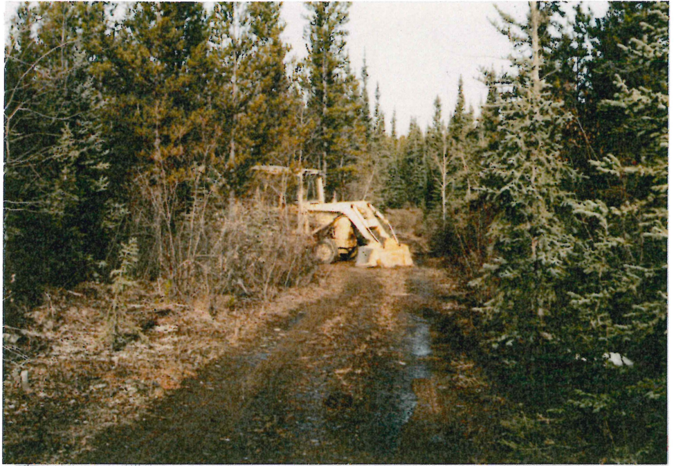
#1-33 LOOKING NORTH ALONG ROAD ADJACENT TO TP 86-11
