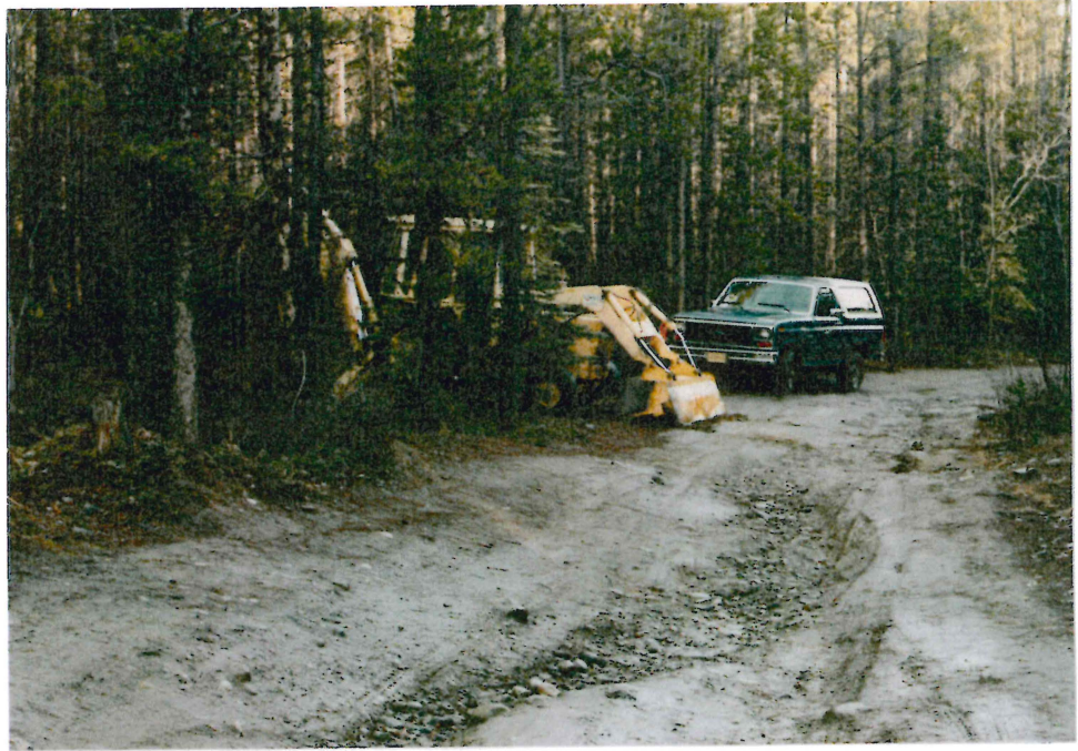
# 1-27 LOOKING NORTH ALONG ROAD ADJACENT TO TP 86-9
