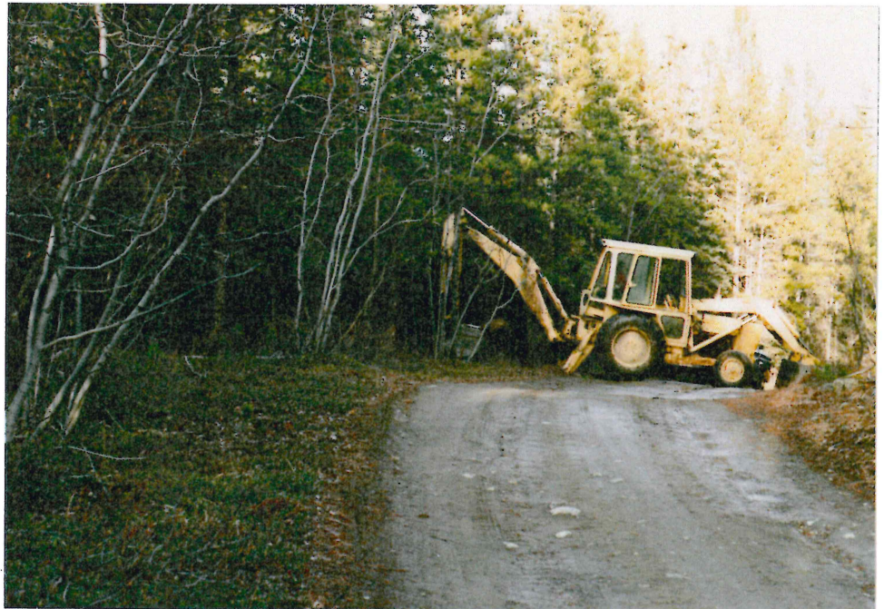
# 2-11 LOOKING NORTH-EAST UP ROAD ADJACENT TO TP BG-16
