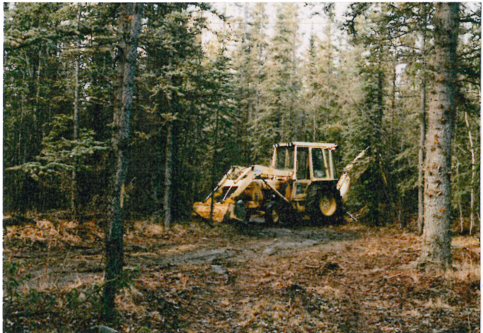
# 1-30 LOOKING WEST ALONG ROAD TO TP 86-10
