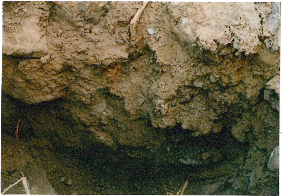
#1-23 LOOKING DOWN TP BG-8 WEST WALL
