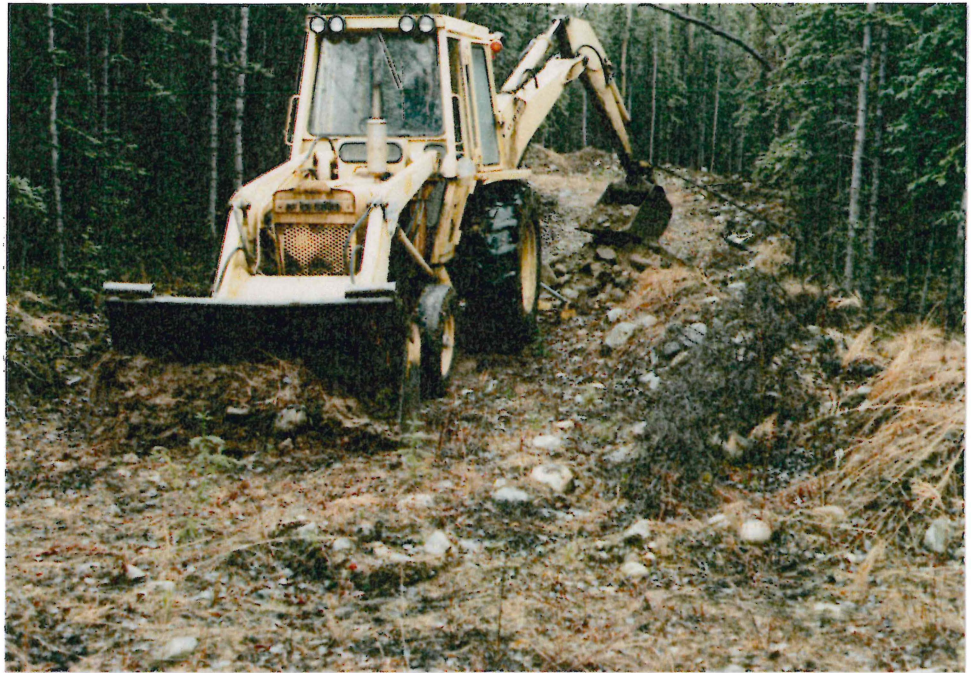
# 3-28 LOOKING SOUTH ALONG ROAD TO TP BG-23, FROM "T" INTERSECTION
