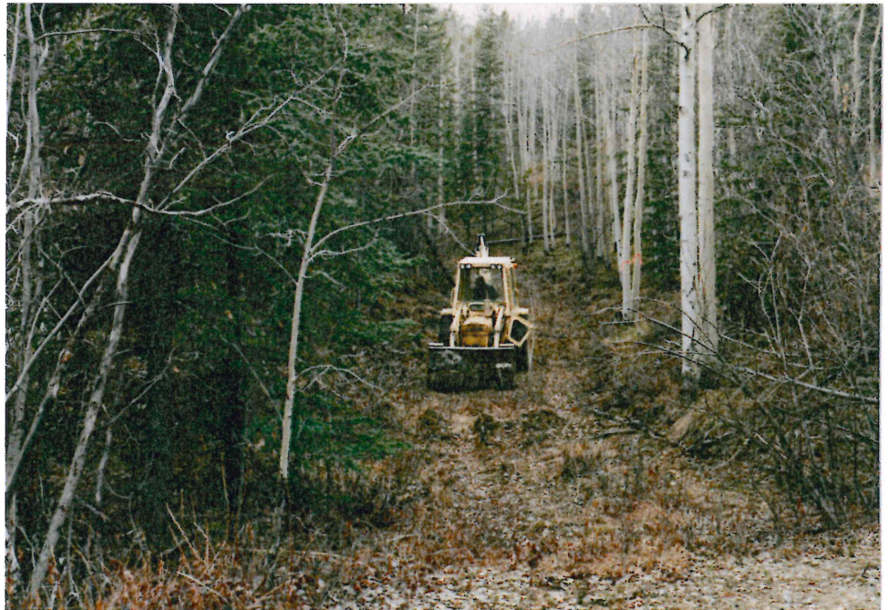
# 3-6 LOOKING WEST ALONG ROAD TO TP 86-18
