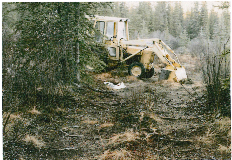
# 1-10 LOOKING NORTH-WEST ALONG TRAIL TO TP 86-4
