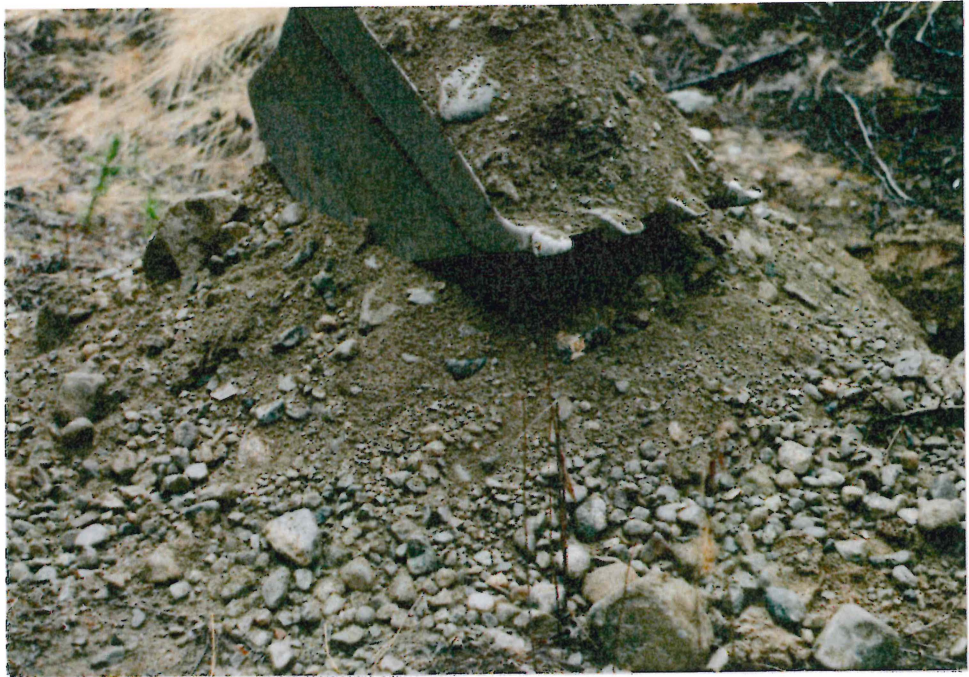
# 3-20 TP 86-21 EXCAVATED SOIL - CLEAN SAND & GRAVEL
