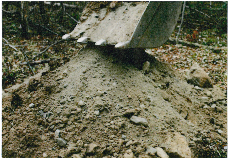
#4-12 TP BG-28 EXCAVATED SOIL
