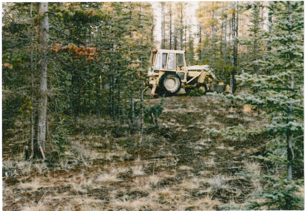
# 1-6 LOOKING NORTH-WEST ALONG TRAIL TO TP 86-3
