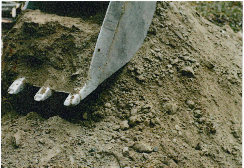
#4-8 TP BG-26 EXCAVATED SOIL
