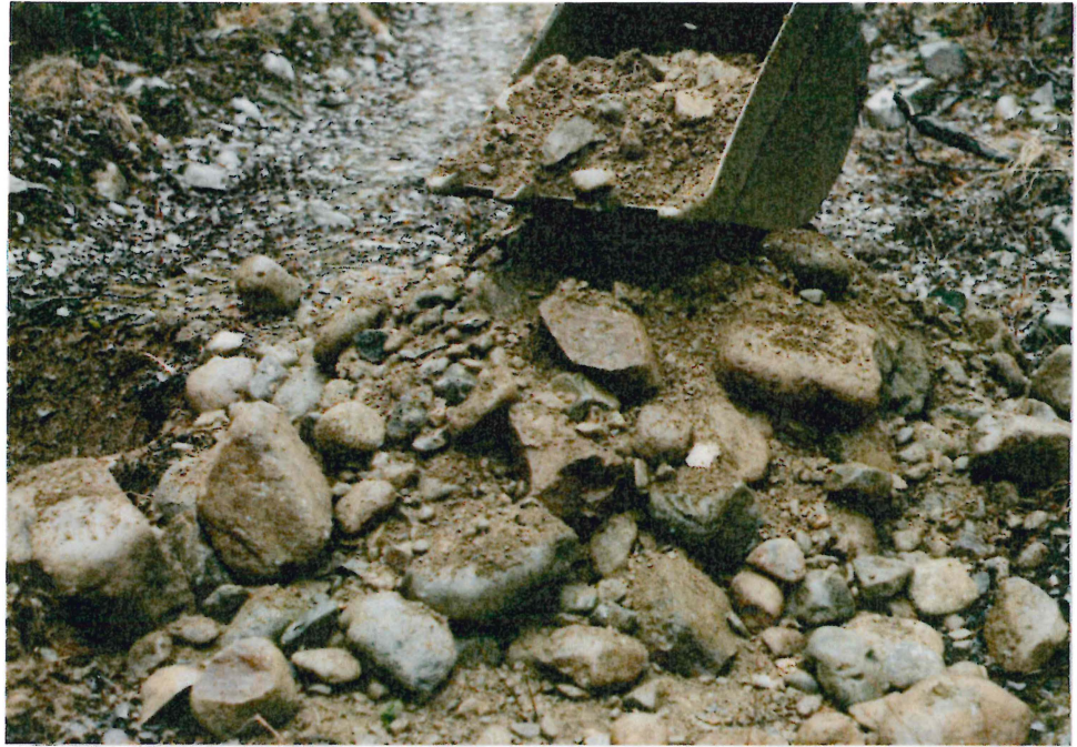
# 3-26 TP 86-23 EXCAVATED SOIL - CLEAN GRAVEL & COBBLES
