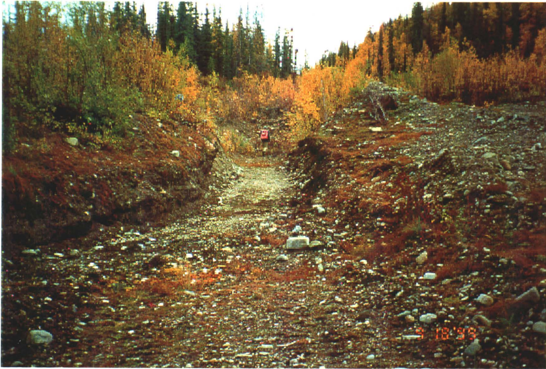
Photo 18-3: Bulldozed trench at second site.
