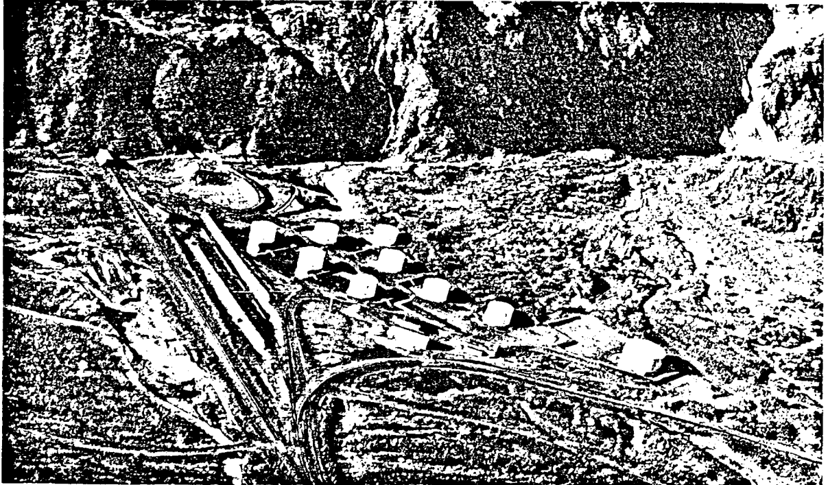
Whittier Tank Farm, located through the Wells Passage in Prince William Sound, contains nine tanks with a total of 275,000 barrels.
