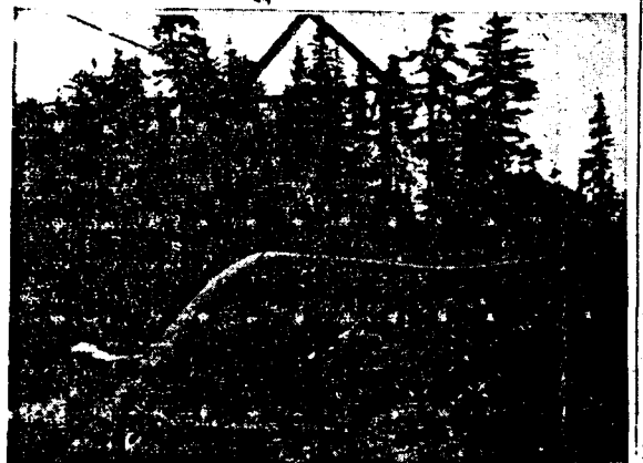
UP AND OVER —This stream bed, now dry, will be a raging torrent in the spring thaws. The heavy steel pipeline had to be bent
