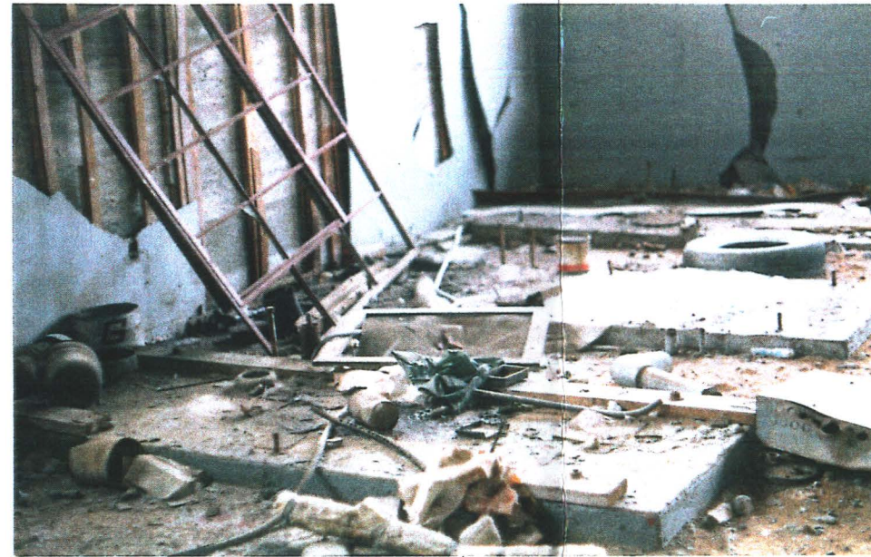
WEST SIDE OF POWER HOUSE
