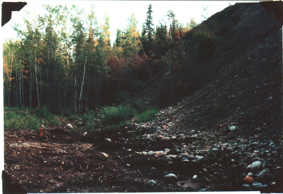
Figure 8. Mayo Landfill - Toe of dump slope with test hole sites flagged.
