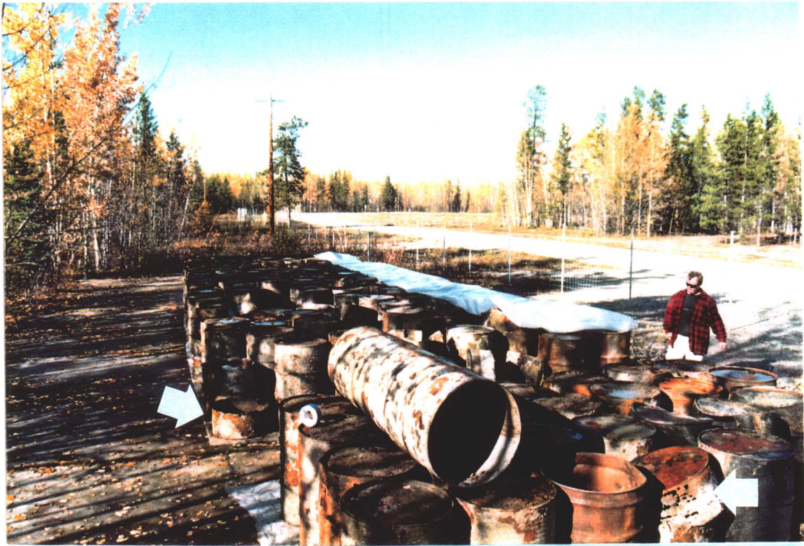
PHOTOGRAPH NO. 13: Plastic sheet being laid over top of stacked barrels. Note poor condition of some of the barrels (arrows).
