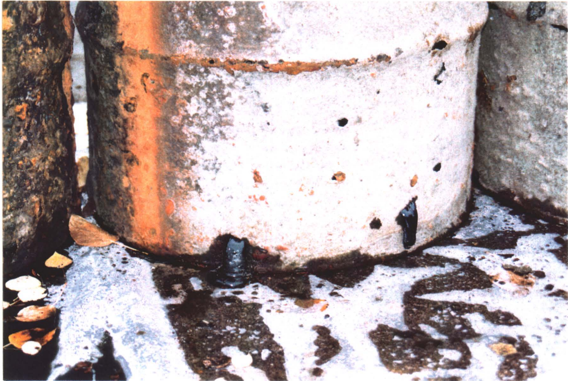
PHOTOGRAPH NO. 17: Black shiny tar-like residue typical of most barrels recovered at the Initial Attack Base. Note higher levels of corrosion damage on the raised rib of the barrel.
