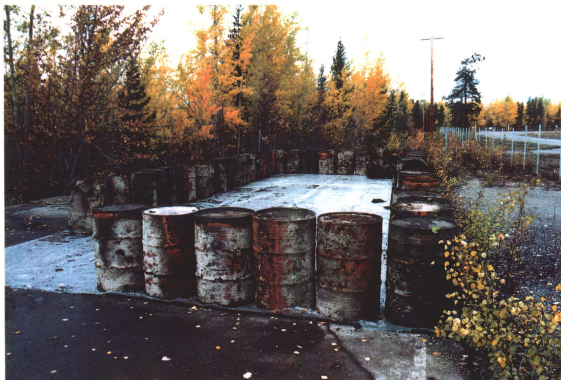
PHOTOGRAPH NO. 12: DIAND storage site. Note plastic ground sheet laid on top of concrete pad.
