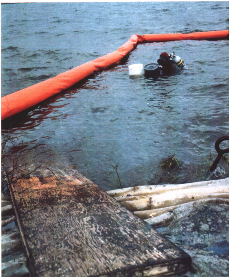
PHOTOGRAPH NO. 10: Diver disconnecting lift buckets inside spill boom prior to barrel removal from water. Note ramp used to roll/lift barrels out of the water up onto the plastic ground sheet.
