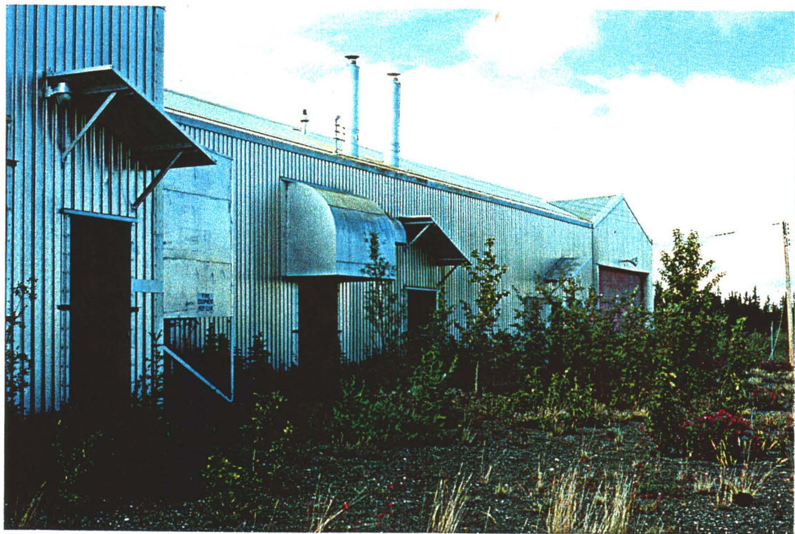
Photo 24: Main building at Destruction Bay. The maintenance garage is at the far end of the building.
