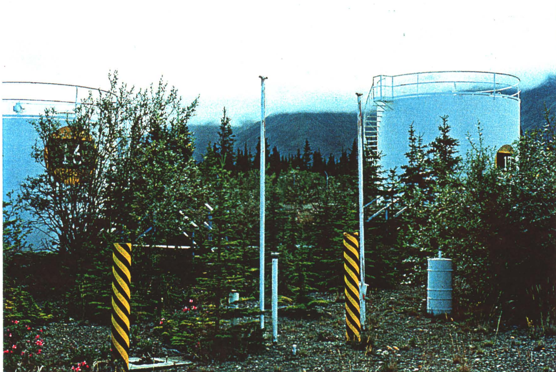
Photo 27: Two AST's on the east side of the main building near the compound entrance.
