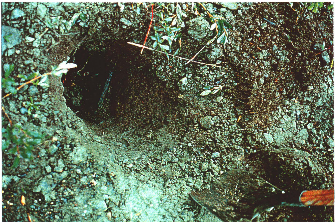
Photo 22: Hand dug excavation into the former landfill exposing waste.
