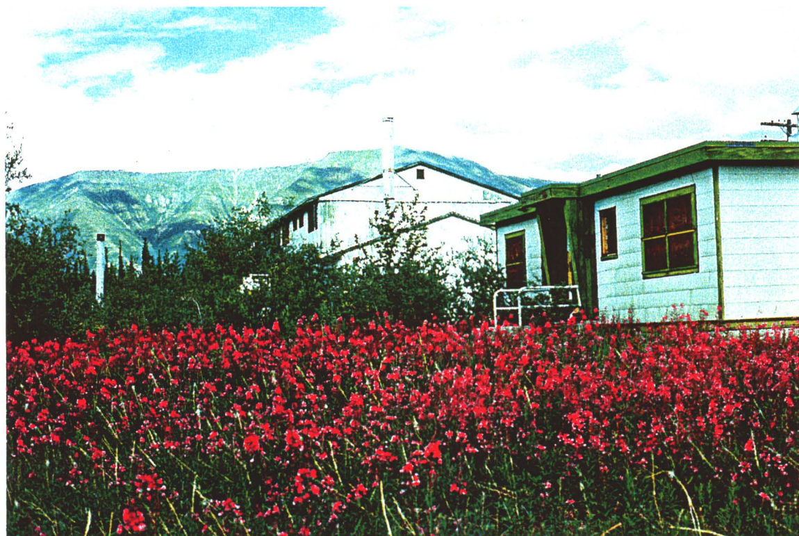
Photo 19: Housing complex at Donjek looking east. Single family dwelling in the foreground and an apartment complex in the background. Note the former incinerator stack to the left of the apartment complex.
