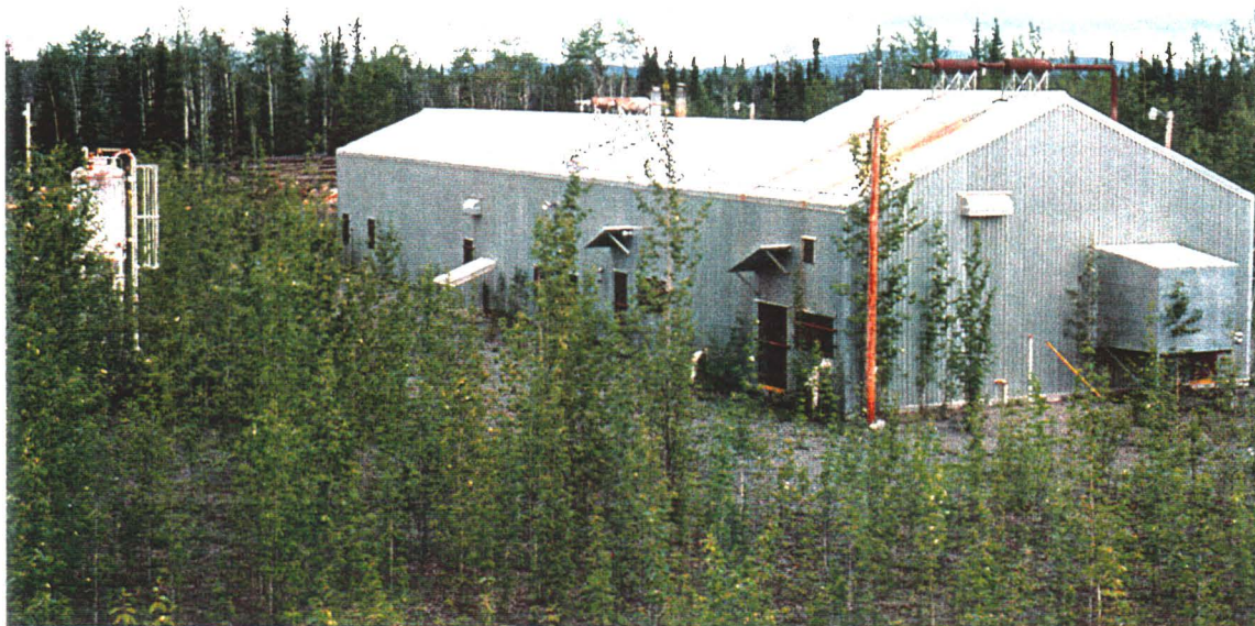
Photo 3: Main building at Beaver Creek looking north.
