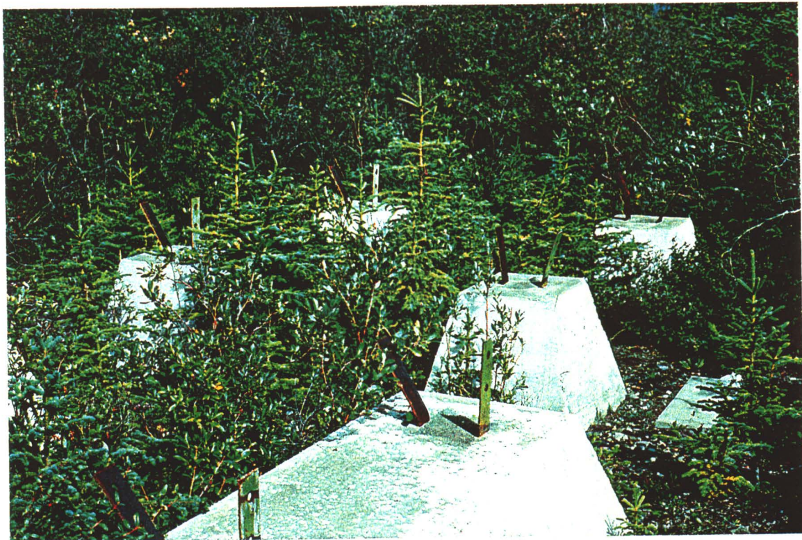
Photo 30: Old foundations located northwest of the former garage along the highway at Destruction Bay.
