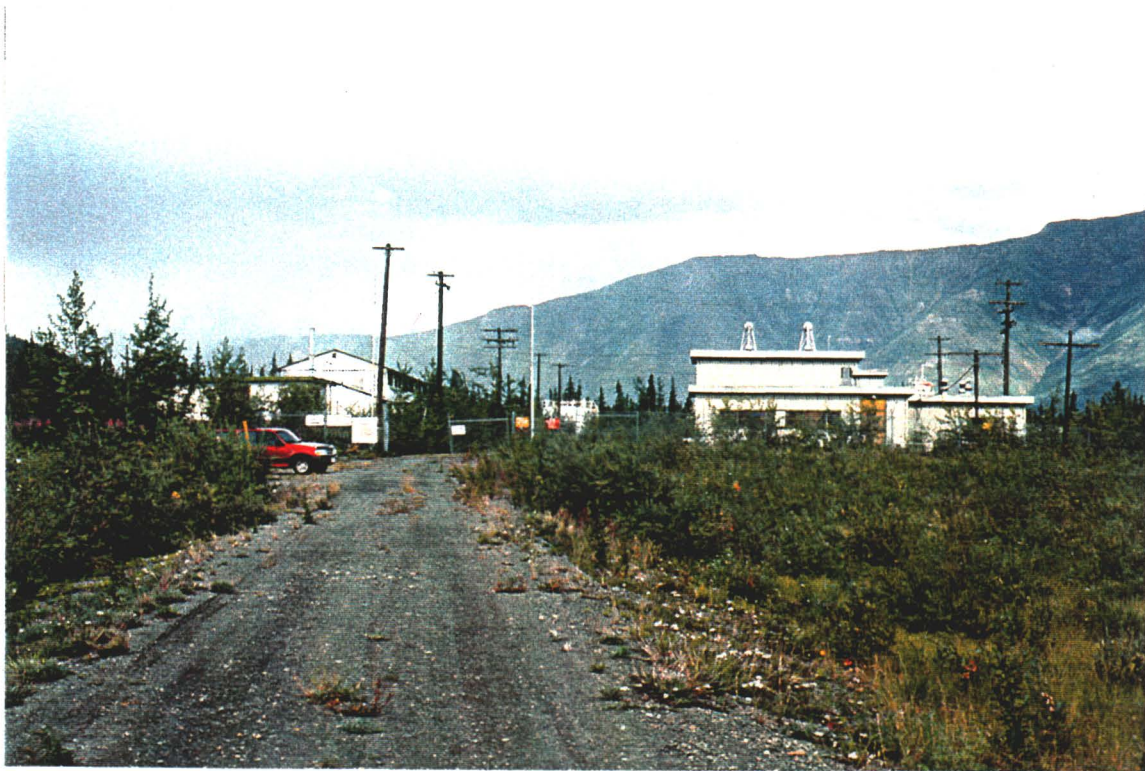
Photo 15: Entrance to Donjek pumping station looking east.
