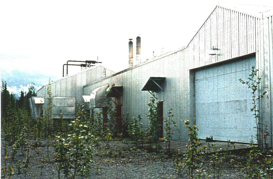
Photo 4: Main building, east side, looking south. Maintenance garage in the foreground.
