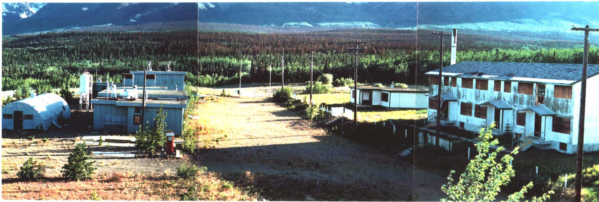
Photo 3.2.3: Haines Junction Pump Station - looking west from the POL tank
