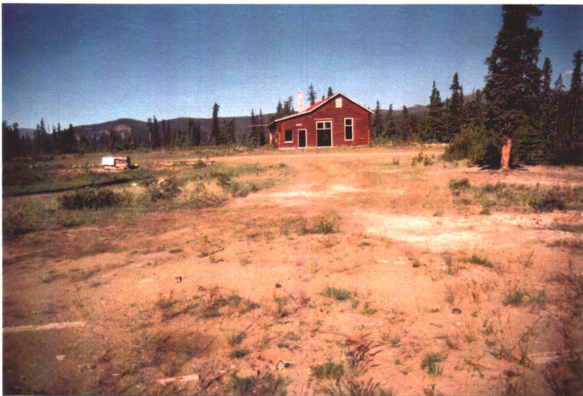
Photograph V-17: The flat area in the foreground was the location of seven POL tanks. The powerhouse can be seen in the background.
