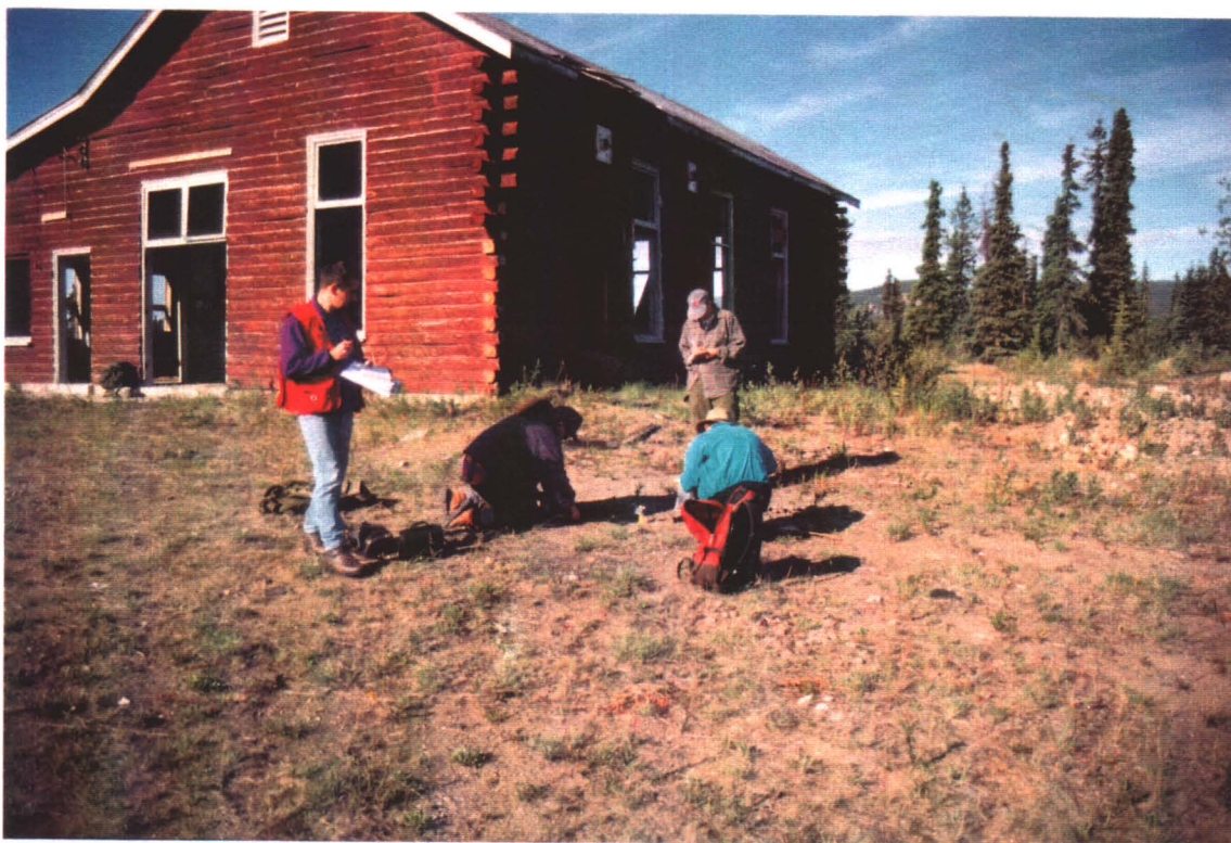
Photograph V-3: View from the northwest side of the powerhouse.
