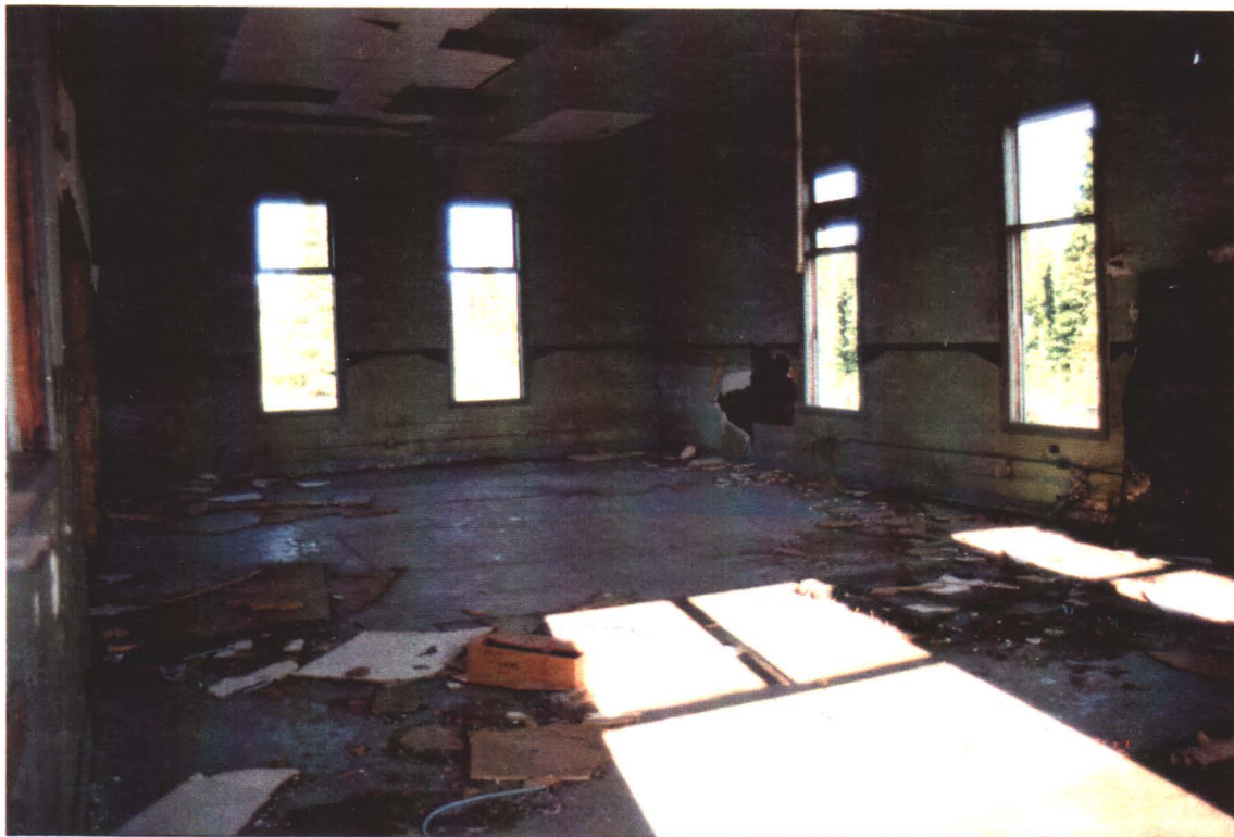
Photograph V-4: Inside the powerhouse in the room that contained the generators.
