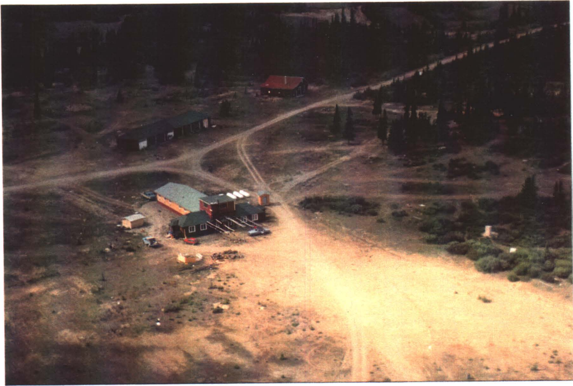
Photograph V-1: Aerial view showing Airways Building, Garage and Powerhouse.
