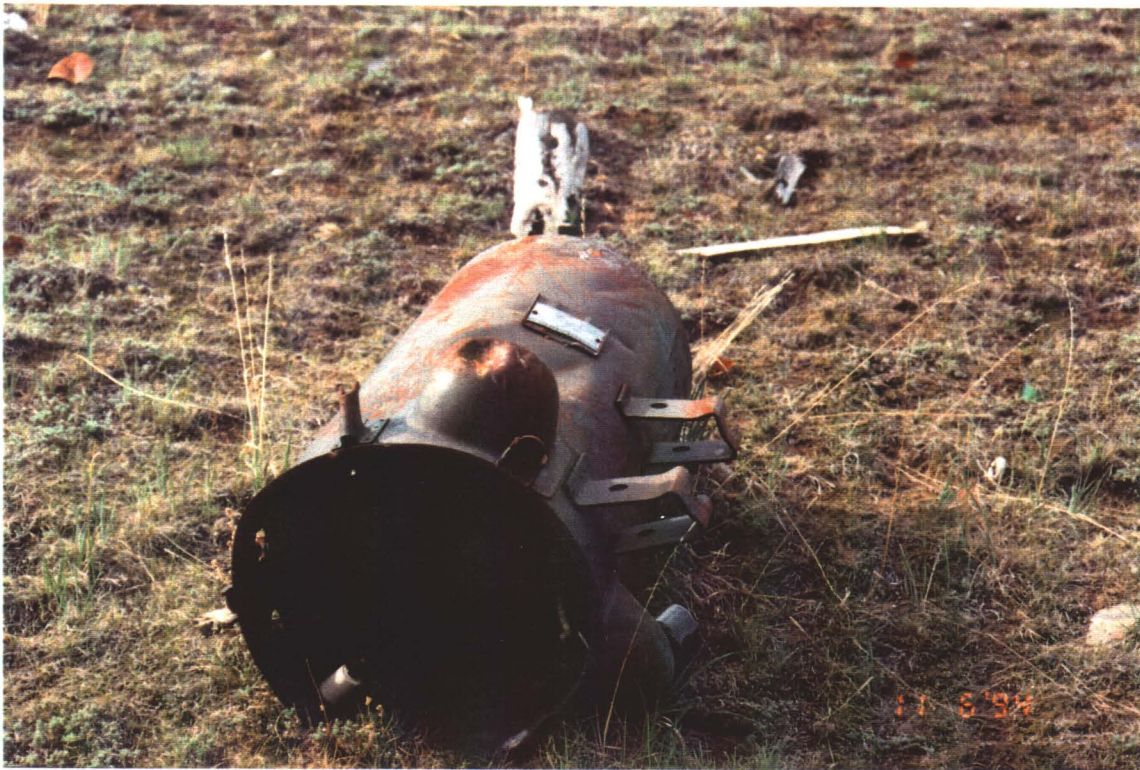
Photograph V-9: Close up view of the transformer in Dump Site 1. This transformer had an oil capacity of 12.5 gallons.
