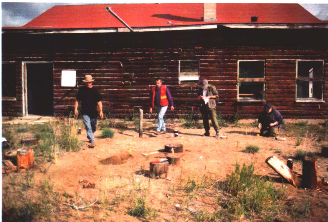
Photograph V-6: The pole stumps are all that remains of the transformer rack that contained four transformers.
