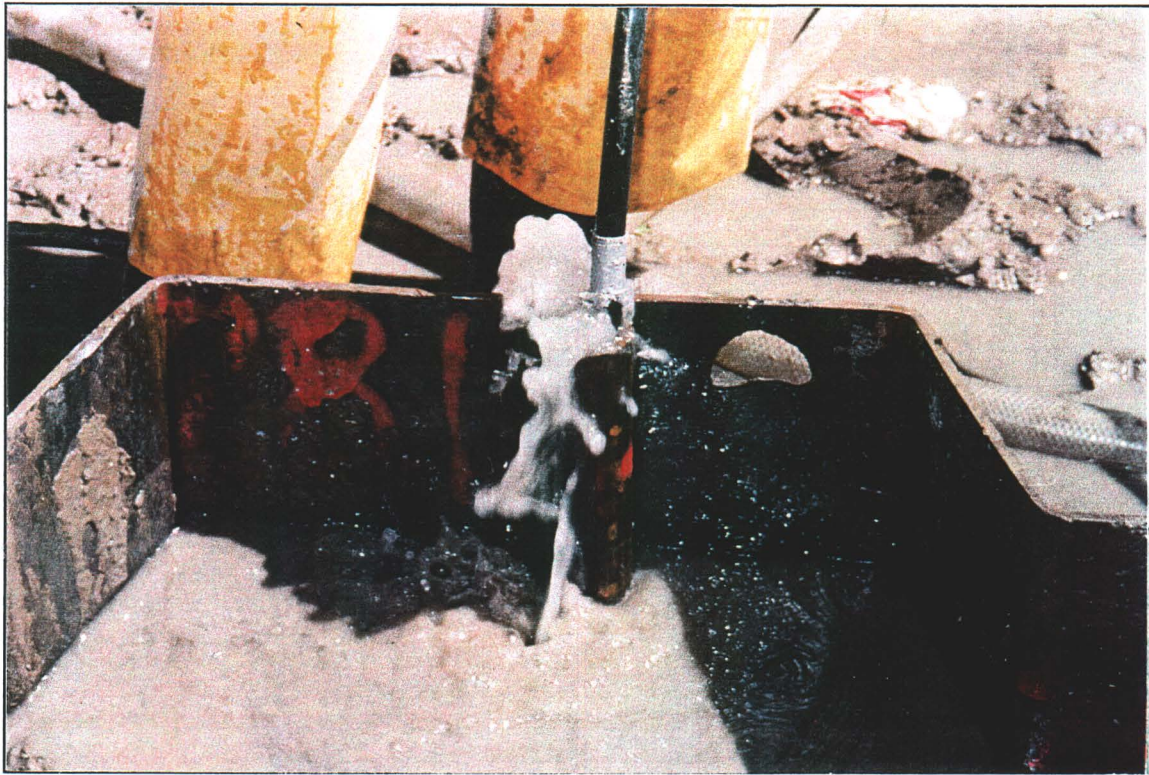
Photo 4: Typical Joint Flushing
