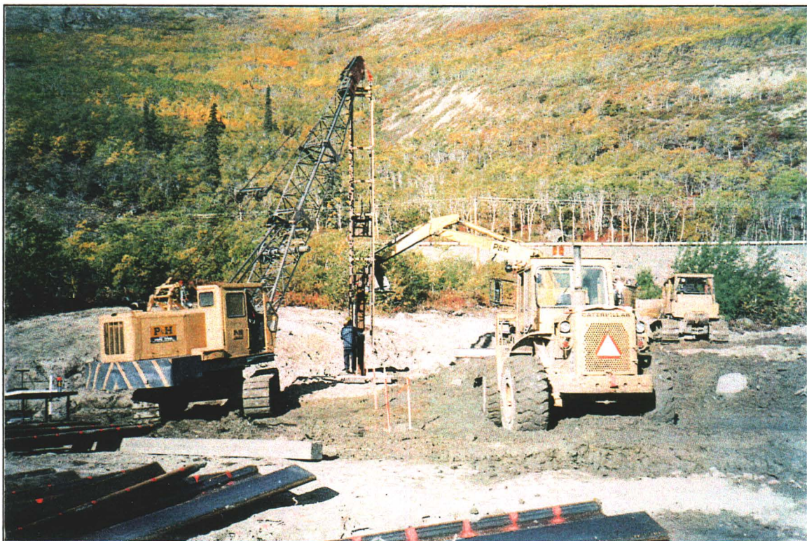
Photo 1: Pile Driving Equipment
