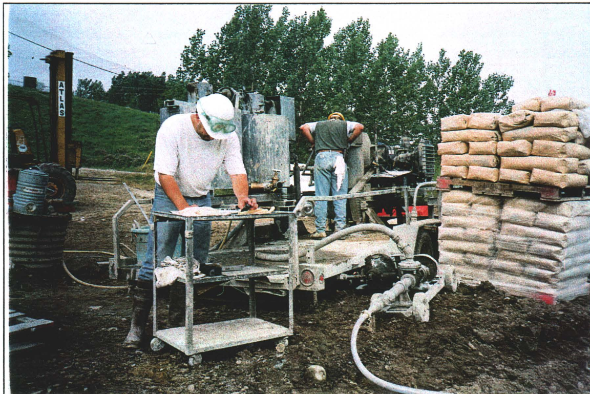
Photo 2: Typical Grouting Equipment
