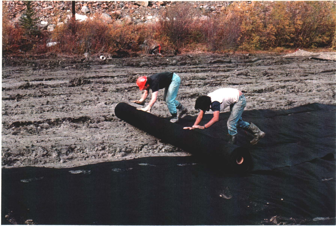
Photo 9: Labourer Placing Geotextile 2 October 1995
