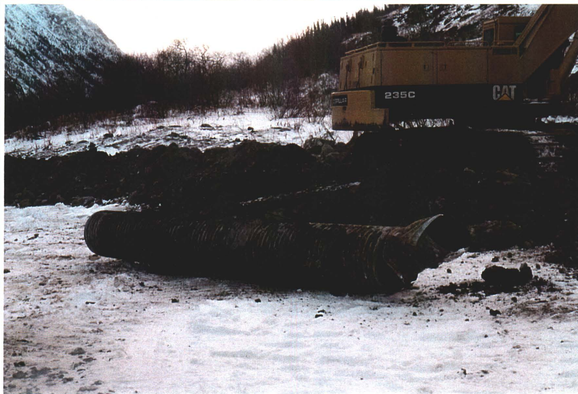
Photo 17: Removal of Section of Old Pipe at Connection Location
