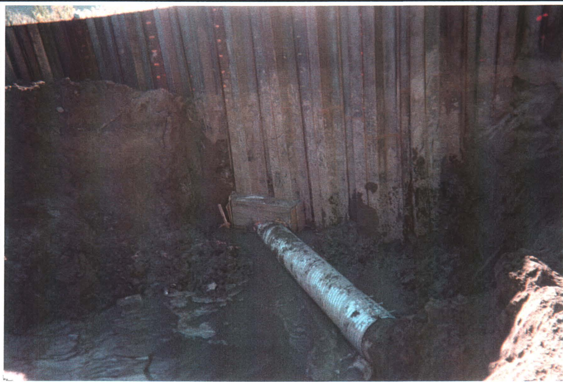
Photo 14: Highway Culvert Repair 17 September 1995
