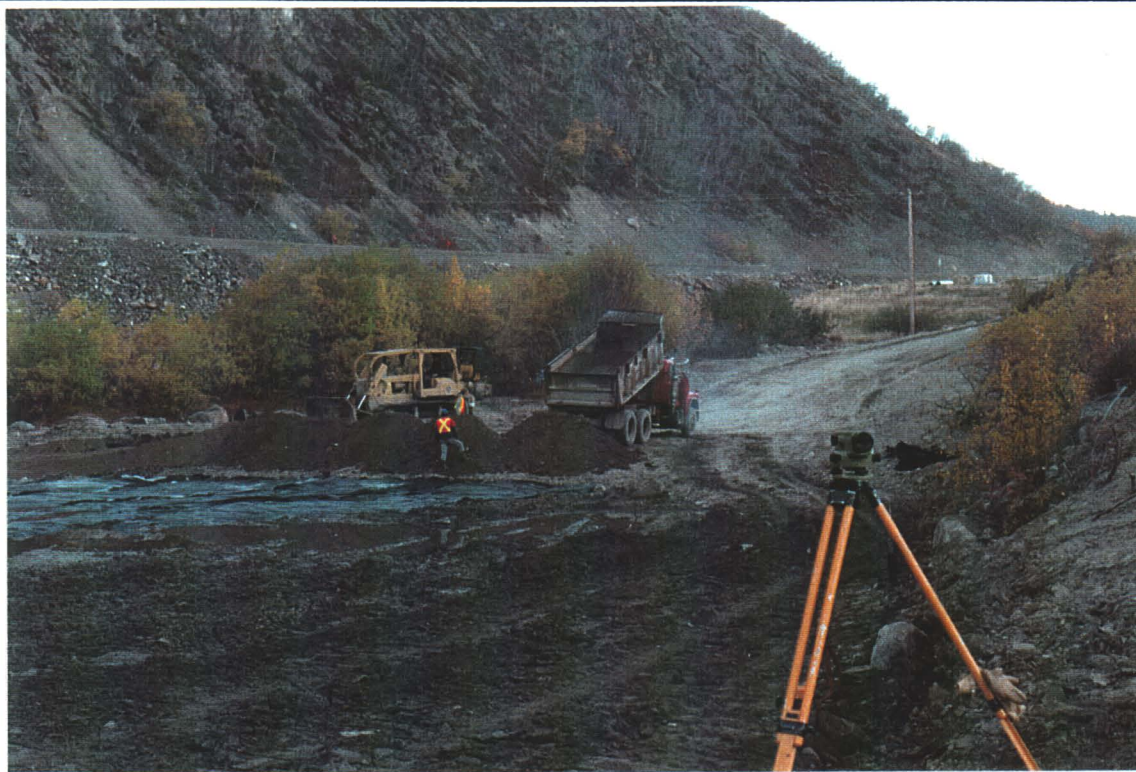
Photo 5: Hauling and Placing of Clay Cap Material 19 September 1995
