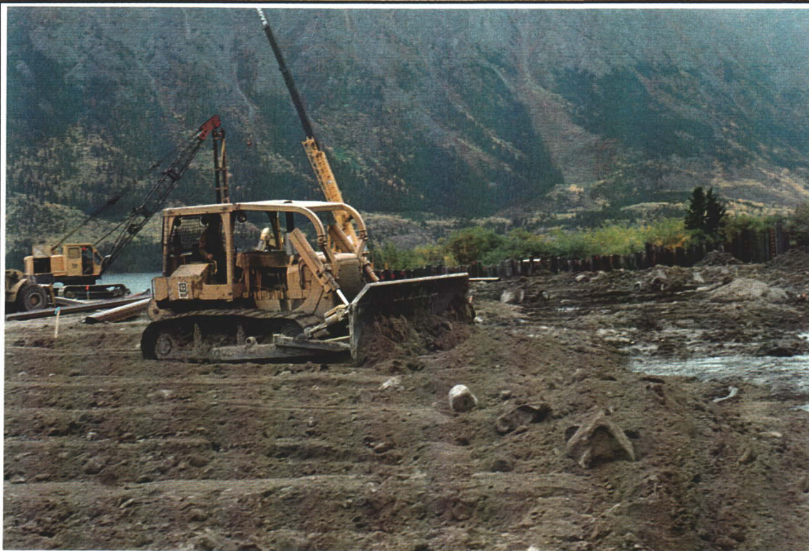
Photo 6: Placing Clay Layer above Geotextile 2 October 1995
