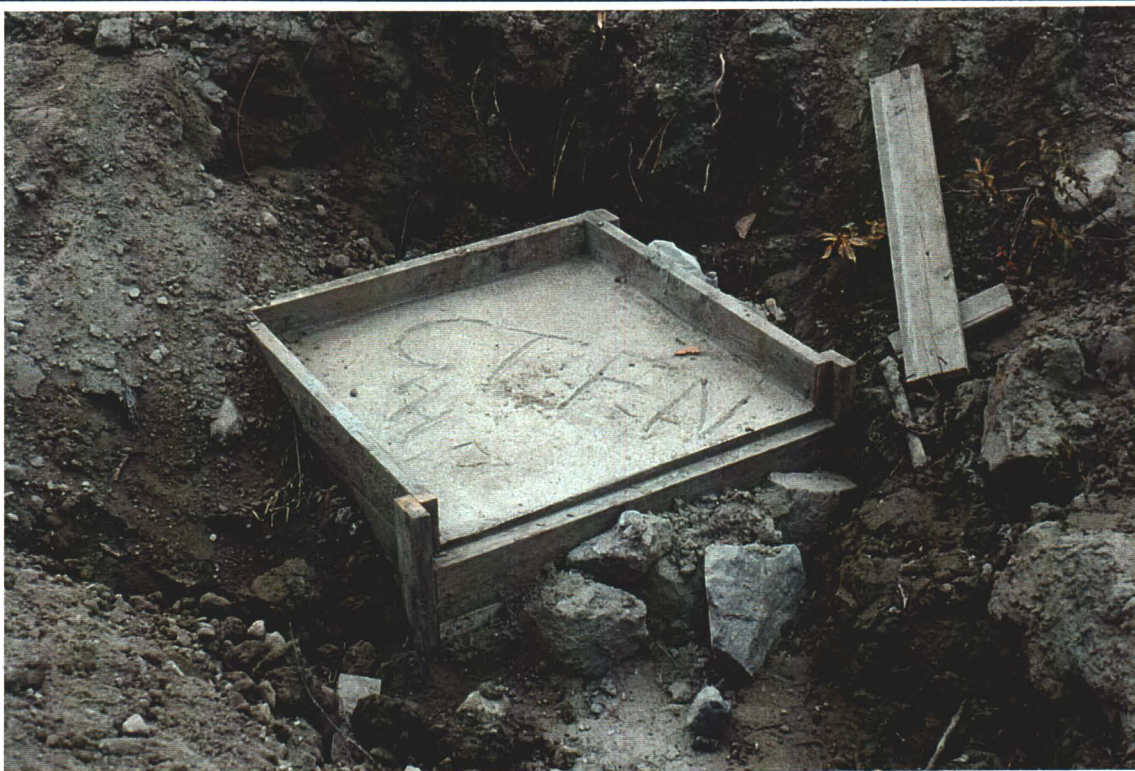
Photo 12: Concrete Plug at Inlet of Decant Pipe 8 September 1995
