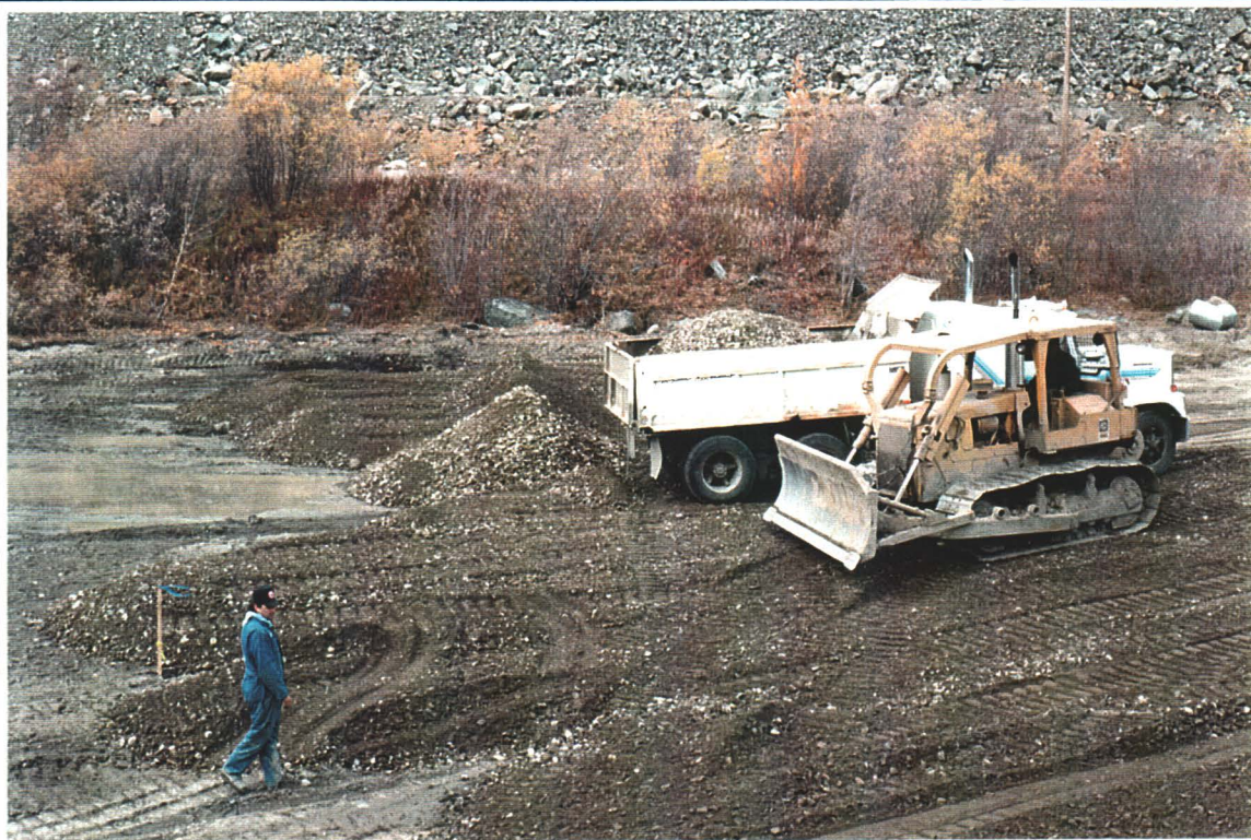
Photo 10: Hauling and Placing of Capillary Break Material 11 October 1995
