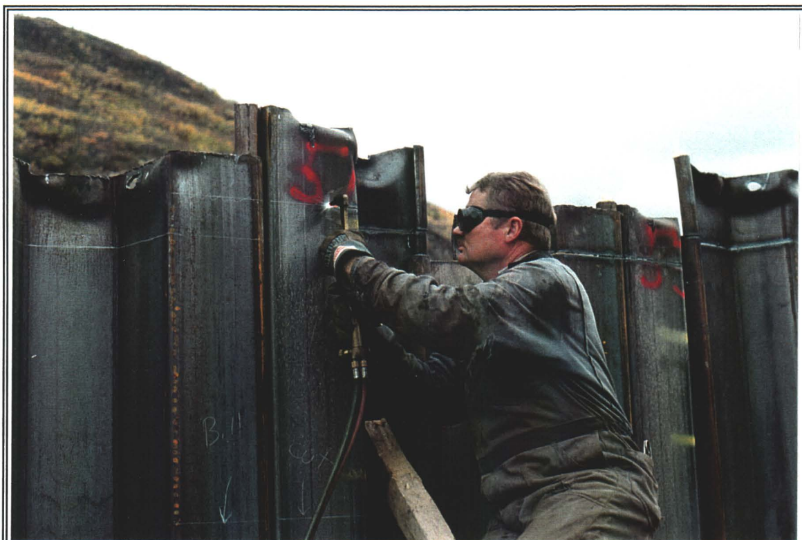
Photo 3: Welder Cutting Top of Wall to Design Elevation 8 September 1995
