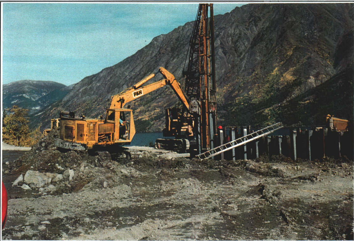
Photo 1: Waterloo Barrier Installation 5 September 1995
