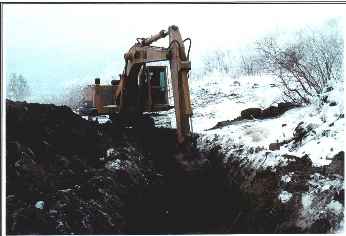
Photo 15: Excavation for HDPE Pipe
