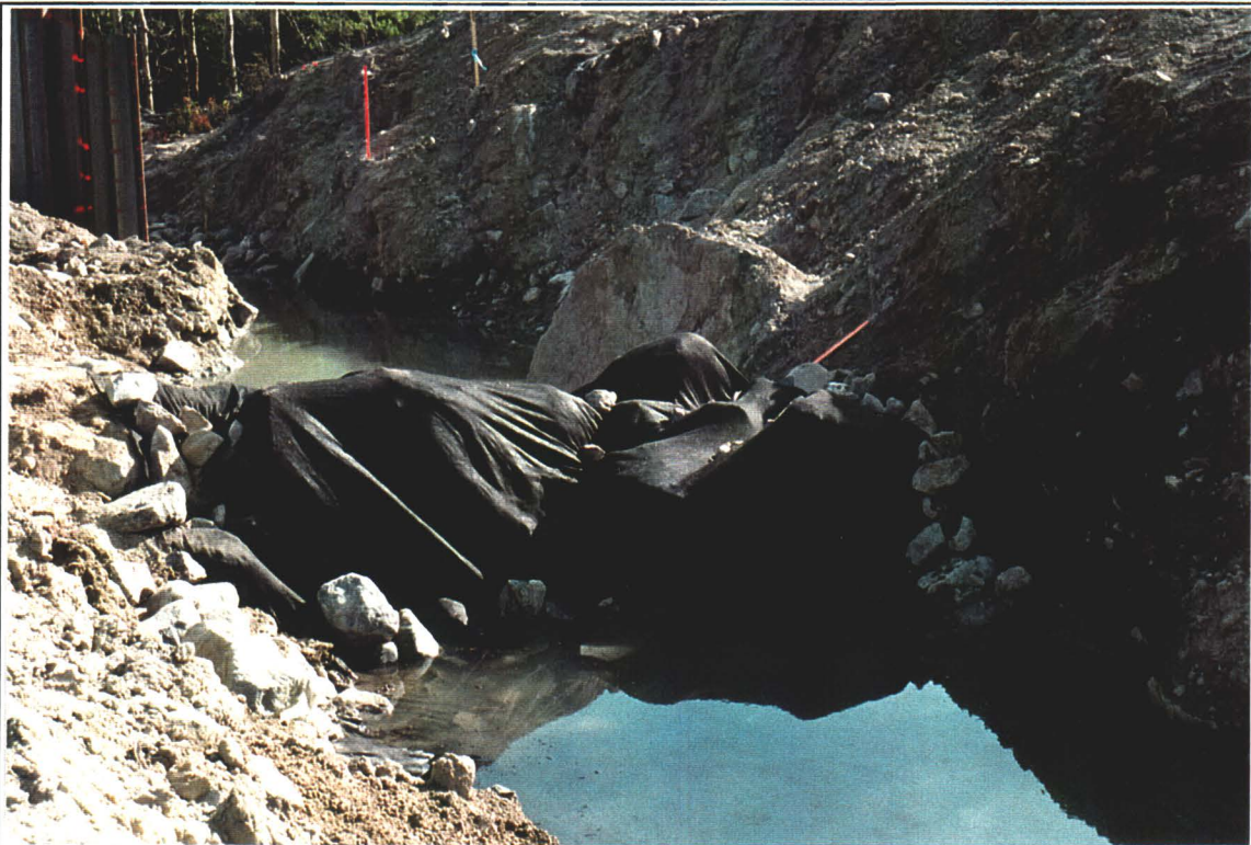
Photo 13: Filter Dike in Temporary Drainage Ditch 5 September 1995
