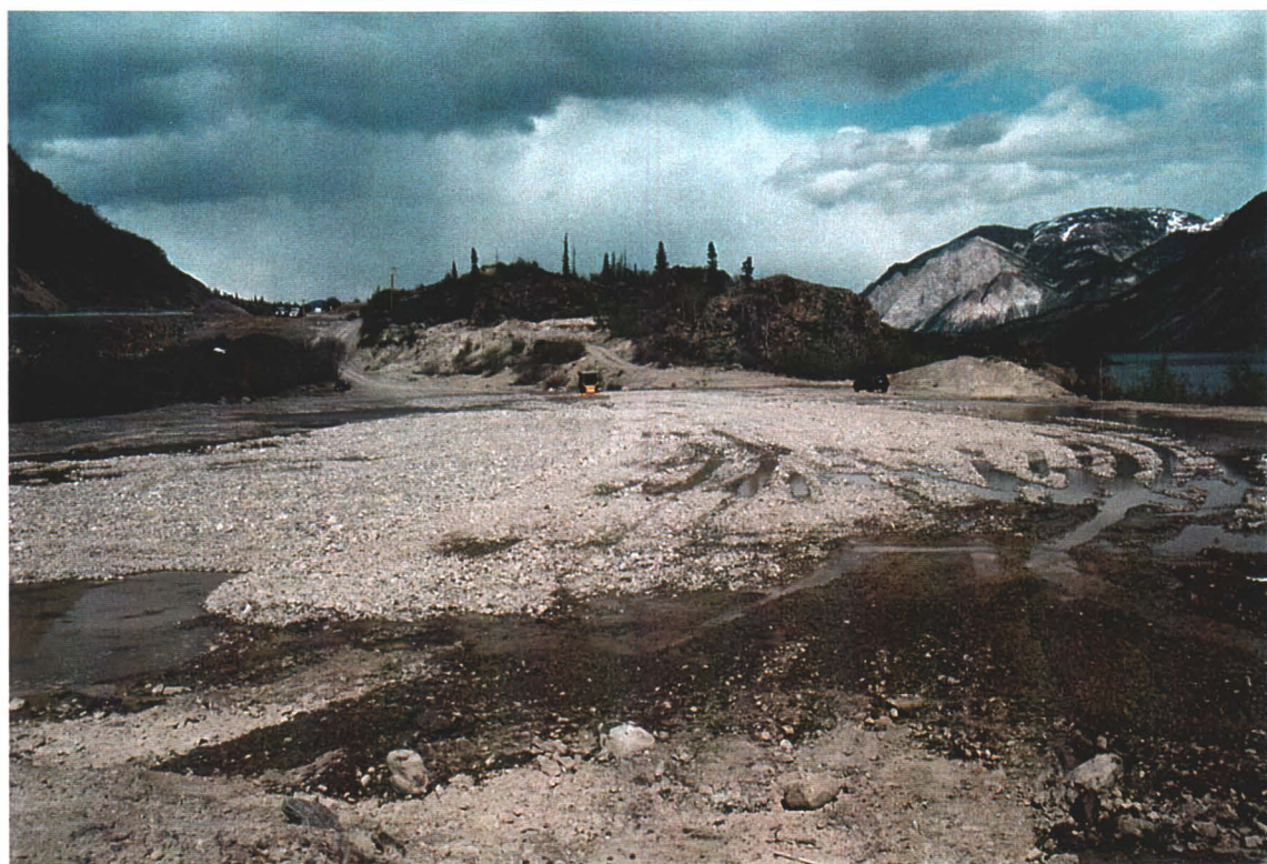
Photo 23: Coarse Material placed in December, 1996
