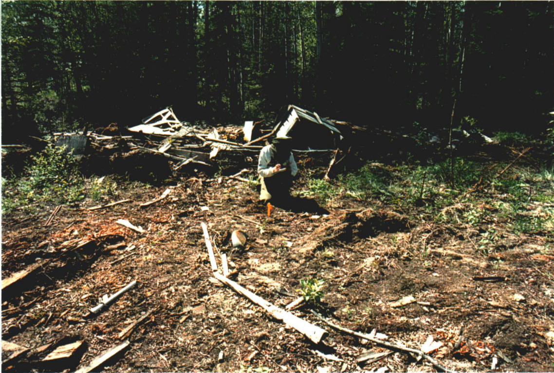
Photograph III-32: The remains of the collapsed storage shack with sample location G6159 in the foreground.
