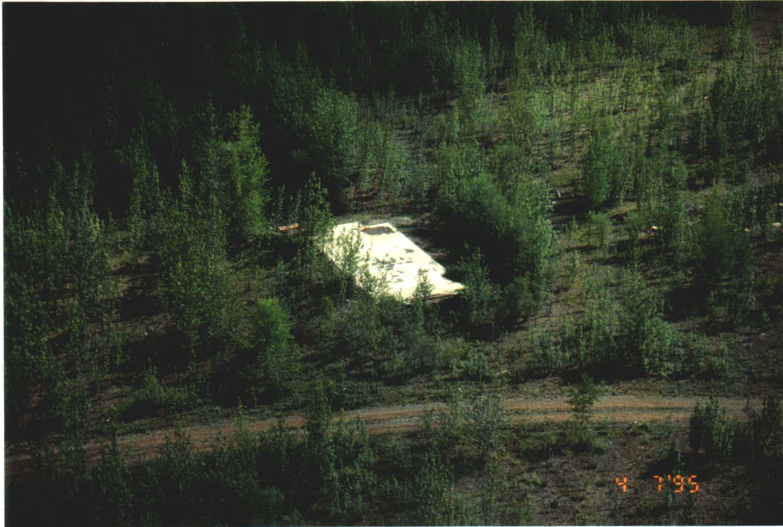
Photograph III-11: Aerial view from the north of the warehouse foundation with Snag Road in the foreground.
