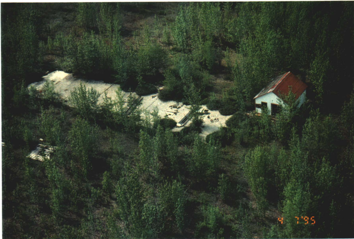
Photograph III-24: Aerial view from the east of the fire hall next to the garage foundation.
