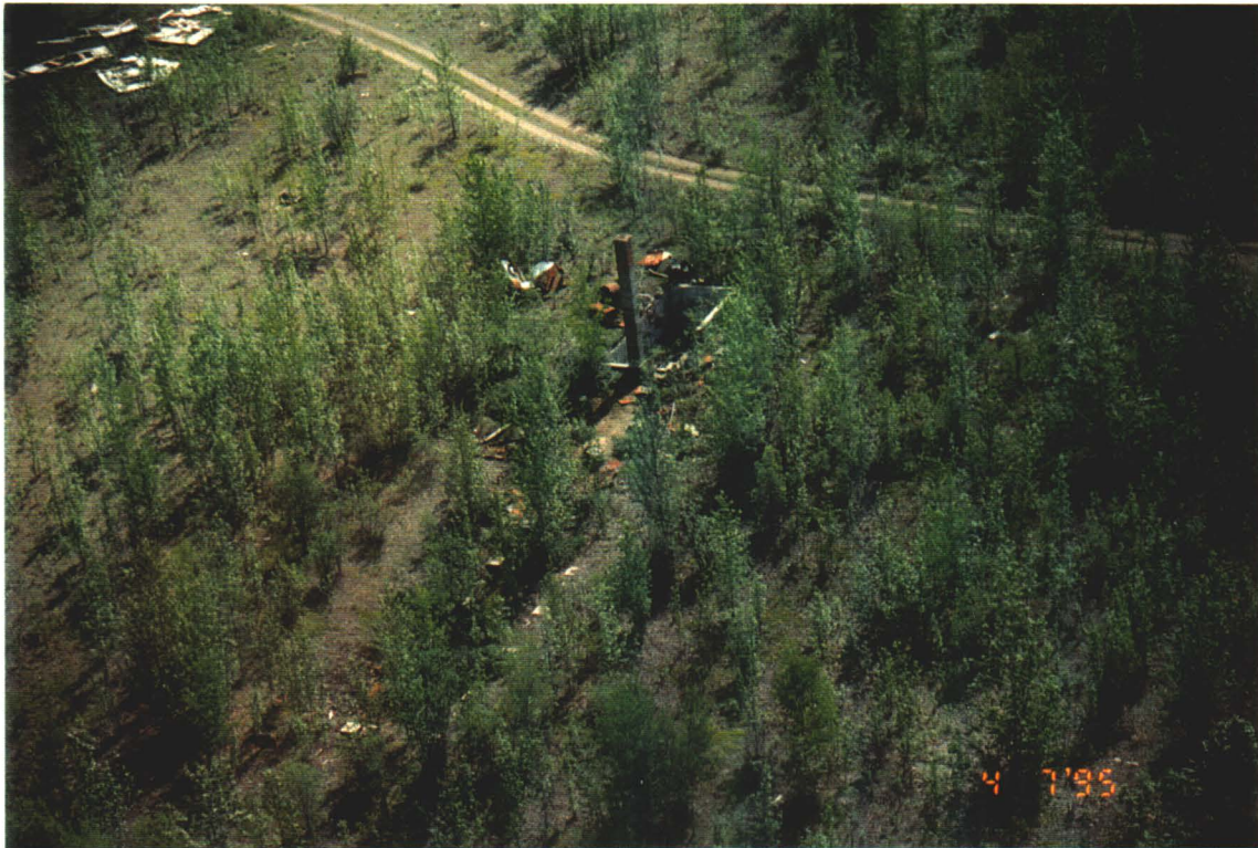
Photograph III-6: Aerial view of the concrete foundation, chimney and pairs of concrete supports marking the former site of the DOT barracks building.
