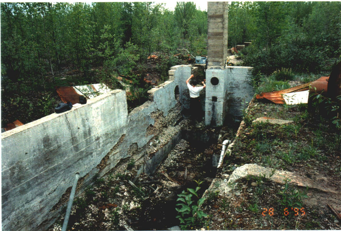
Photograph III-7: DOT Barracks Building basement as viewed from the south.
