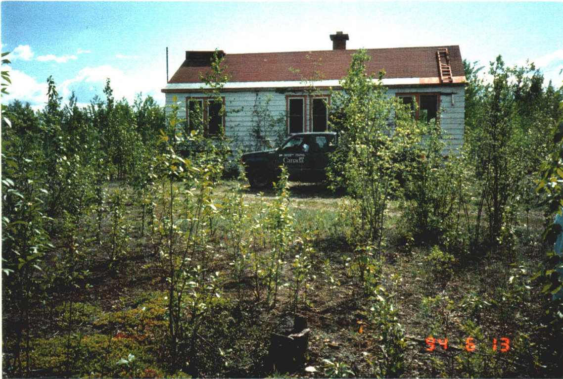
Photograph III-2: The tower building as it appeared during the preliminary investigation of Snag Airstrip in 1994.
