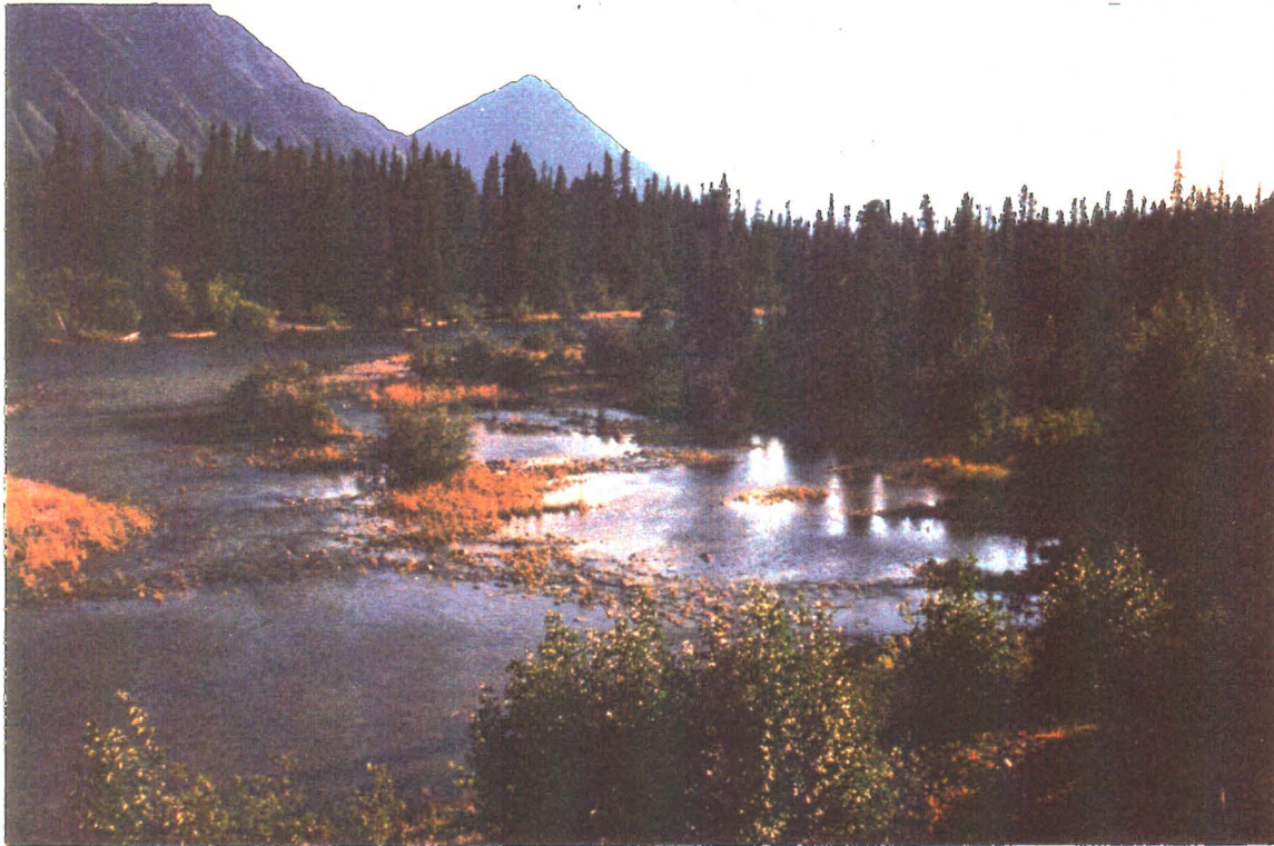
Photograph 39-P1: Upriver view of the Kathleen River as seen from the Haines Highway bridge over it. Site 39 is on the right.
