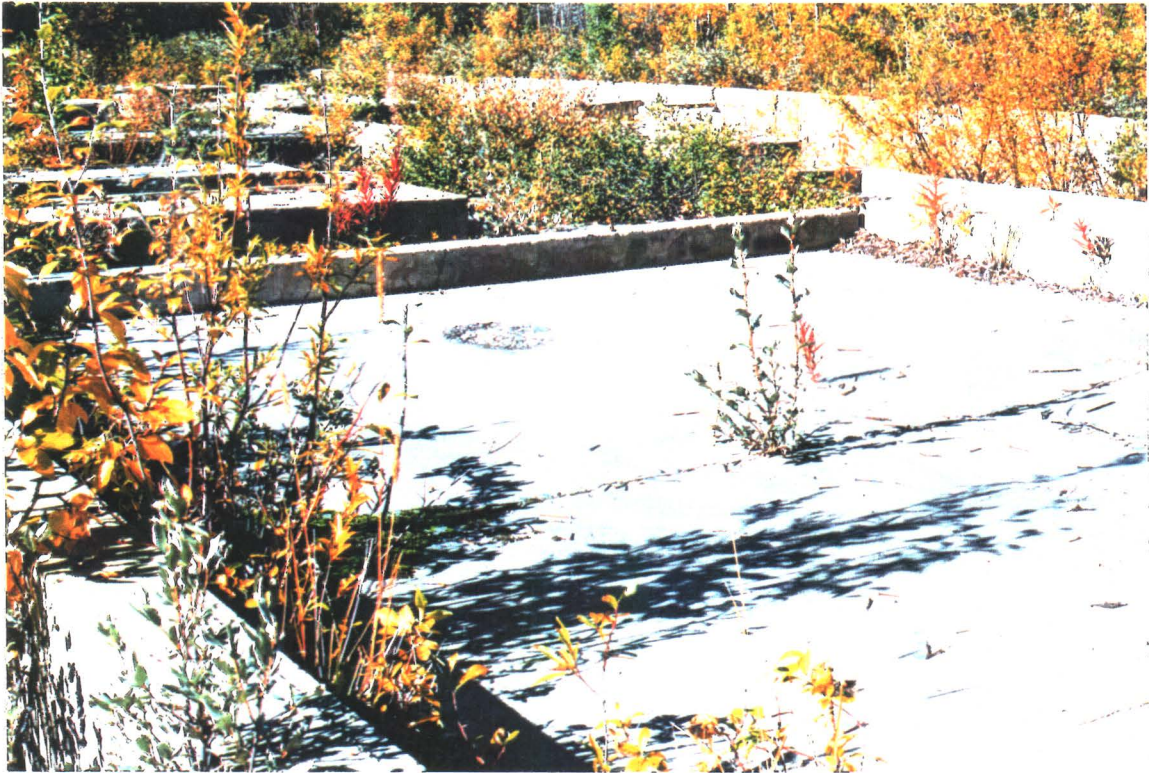
Photograph 30-P4: View of the concrete foundation facing northwest.
