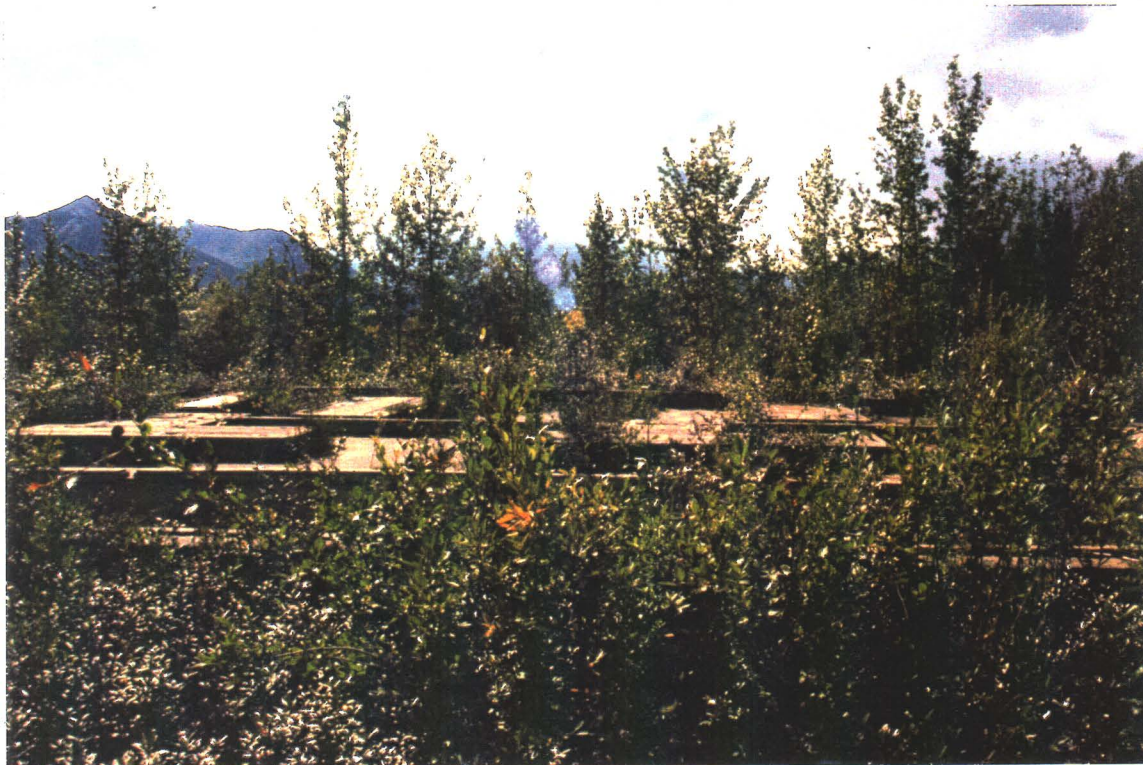
Photograph 30-P5: View of the concrete foundation facing south.
