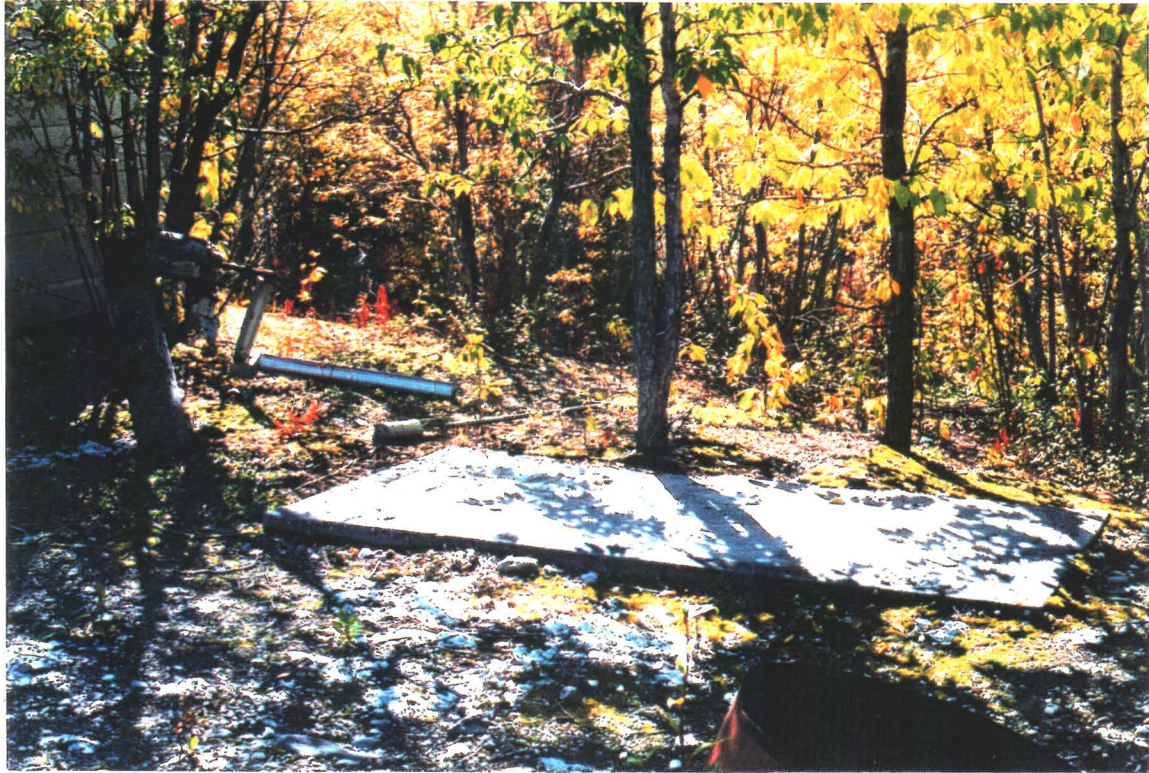
Photograph 30-P3: Small concrete pad to the east of the pumphouse. The left side of this pad was sample site 30-S24.
