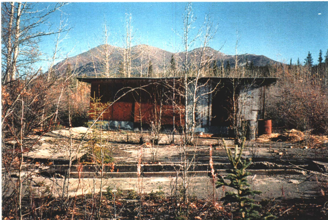
Photograph 4. Oil change pit and shed on subject site. September 1996.
