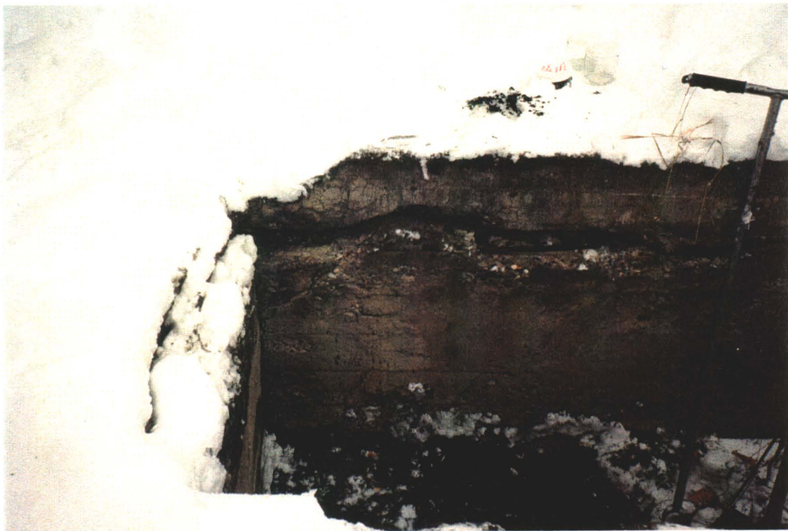
Photograph 9. Interior of oil change pit on subject site. October 1996.
