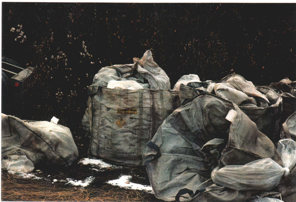
Photograph 12. Ammonium nitrate leaking from sacks in the highway construction materials storage area on the subject site. September 1996.
