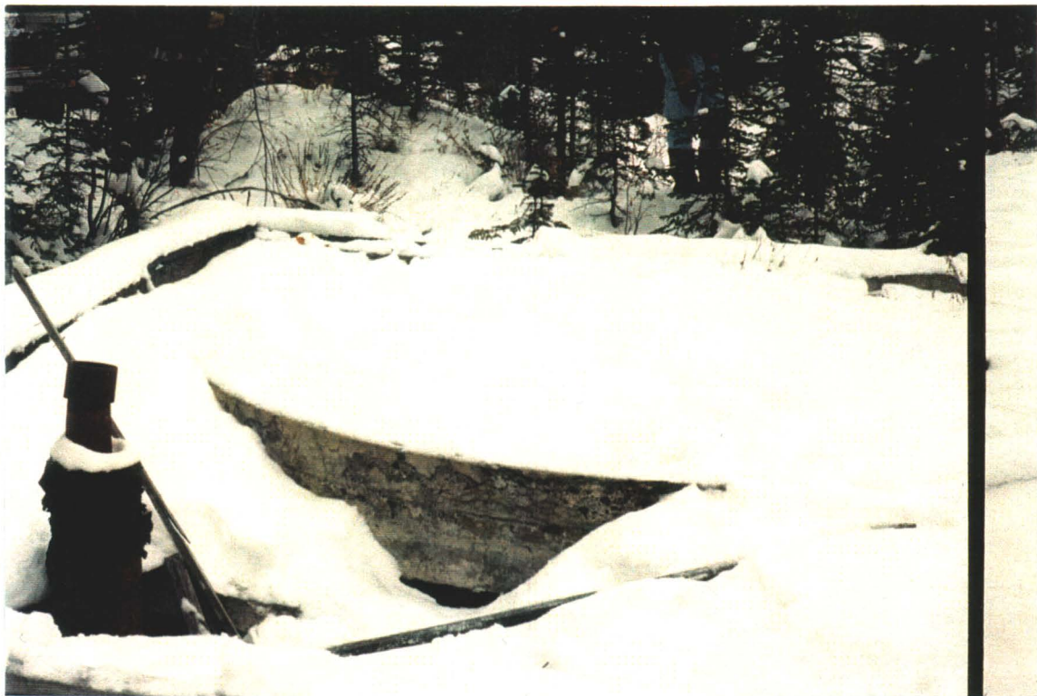
Photograph 7. View of Canol Pump Station G, MP 1166. October 1996.
