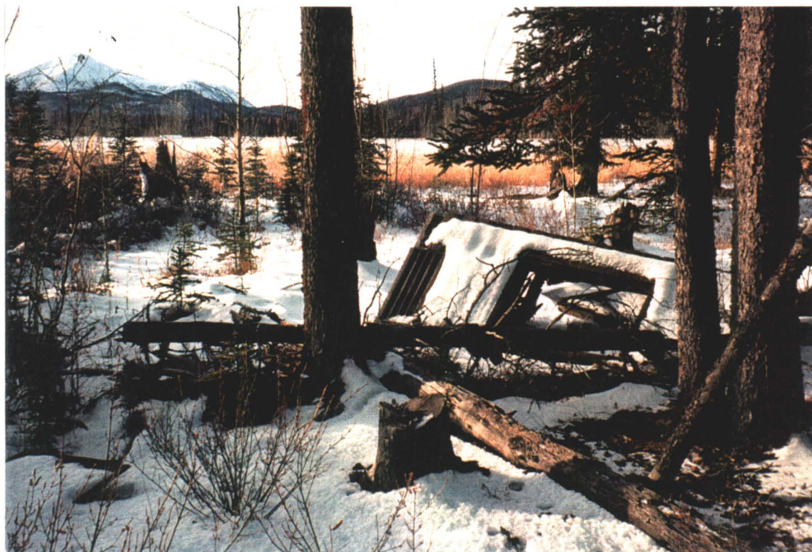
Photograph 21. Building Debris on Northern Side of the Alaska Highway, Bear Flats - White River Site. October 1996.
