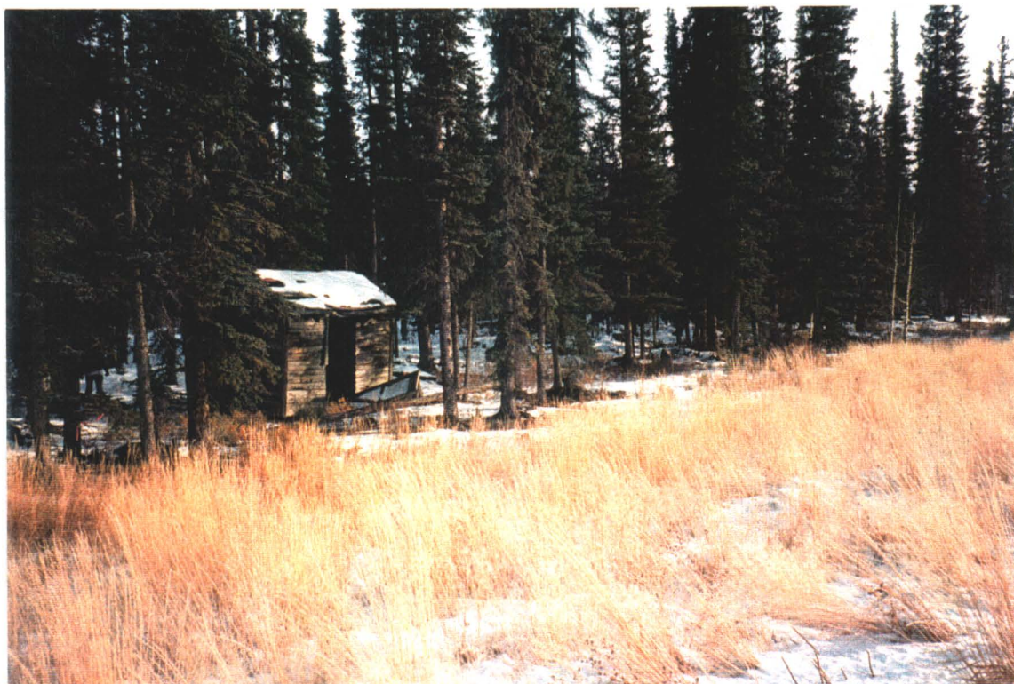
Photograph 22. Abandoned Building on Northern Side of the Alaska Highway, Bear Flats - White River Site. October 1996.
