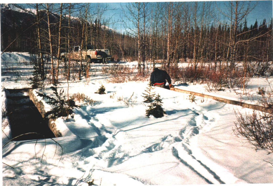
Photograph 20. Oil Change Pits, Bear Flats - White River Lodge, MP 1167.5. October 1996.
