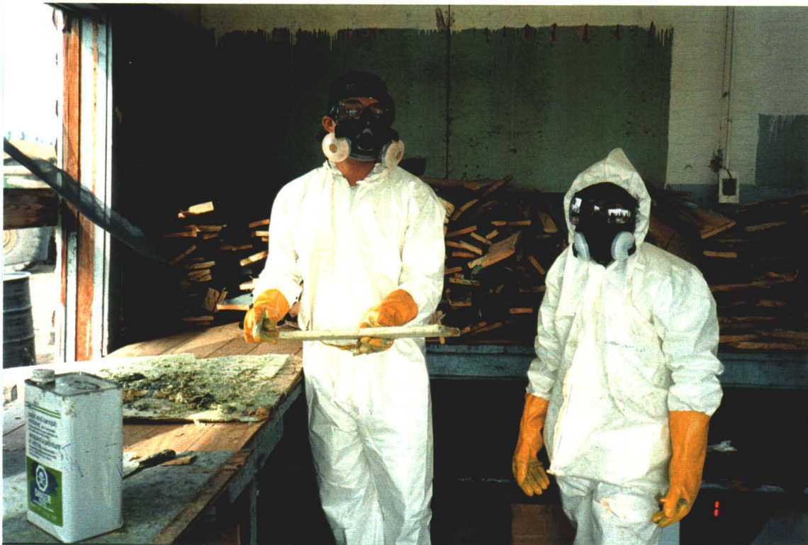
Photograph IV-4: Powerhouse wooden plank during chemical paint stripping.
