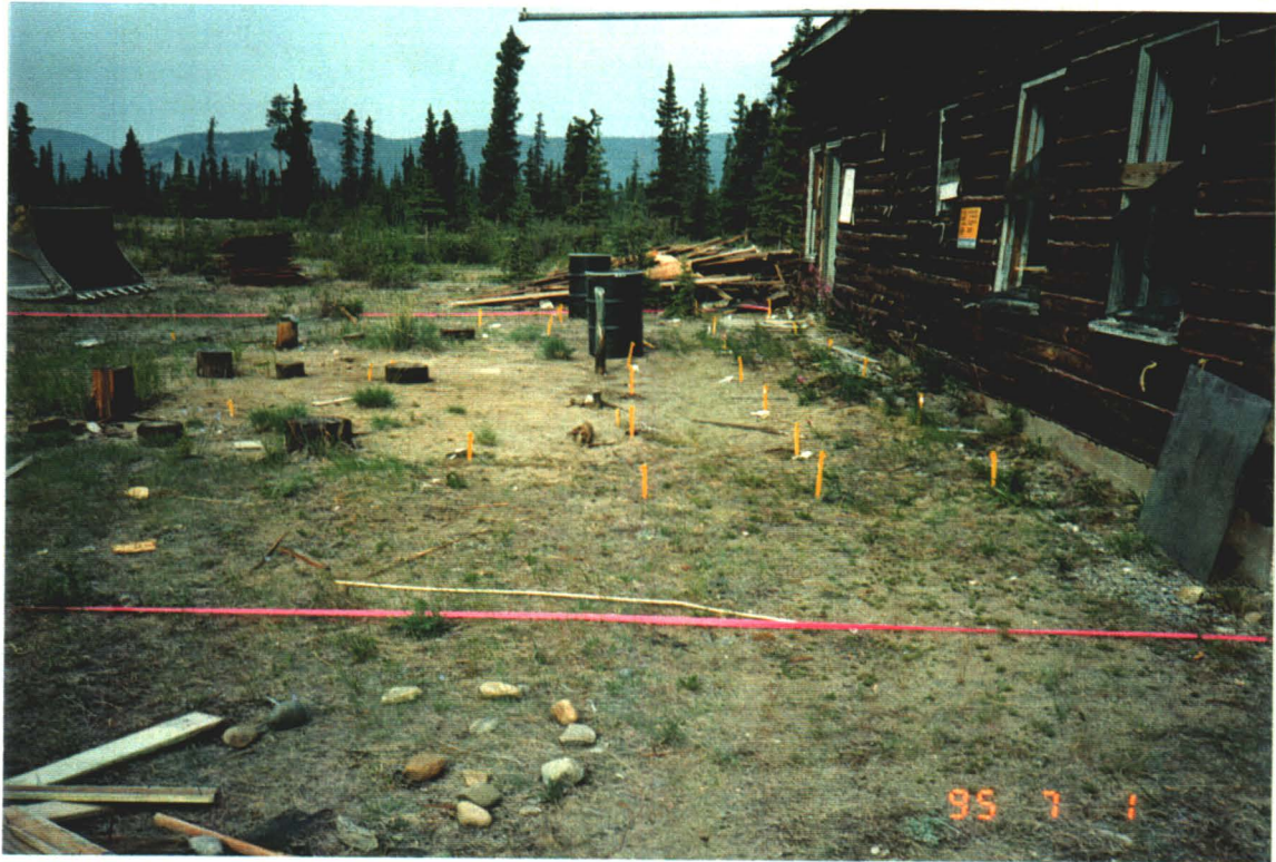
Photograph III-4: Delineation and demarcation of contaminated area at AA108 and AA115 the powerhouse south stain.
