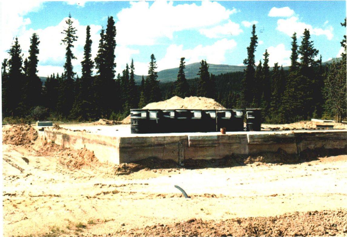
Photograph IV-9: Barrels awaiting shipment off site, temporarily stored on powerhouse concrete pad.
