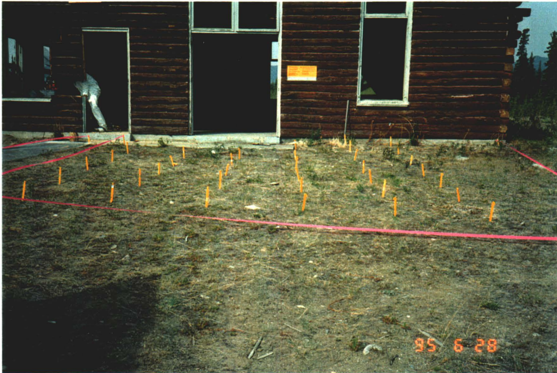
Photograph III-1: Delineation and demarcation of contaminated area at AA101, the powerhouse east stain.
