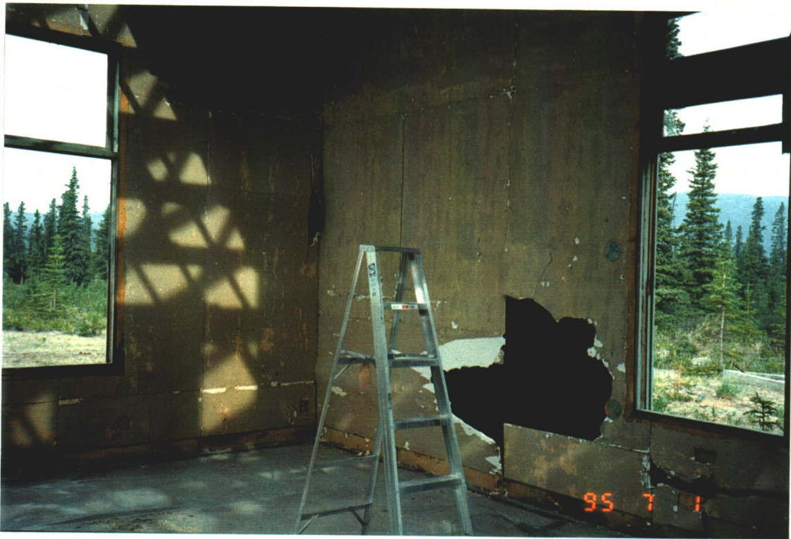
Photograph IV-3: Powerhouse walls after physical paint stripping.
