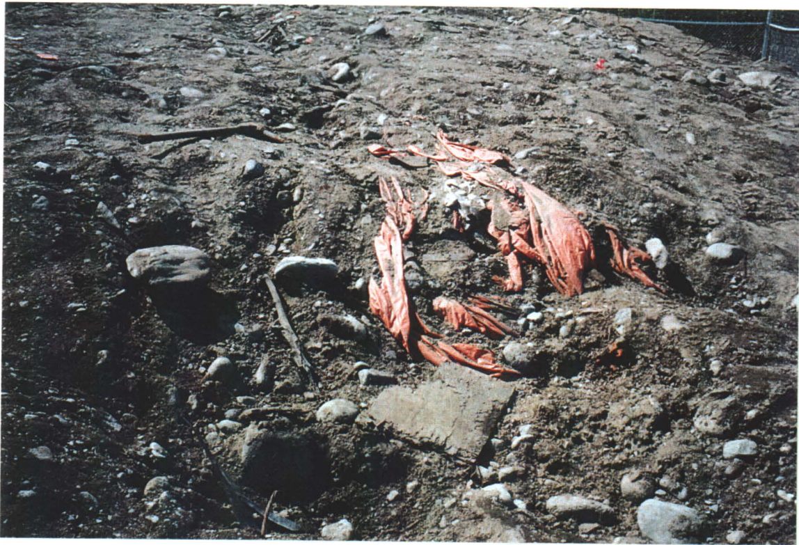
Photograph 2.3: Surface of contaminated soil at the Temporary Storage Facility showing rocks, tarpaulin, wood and metallic debris
