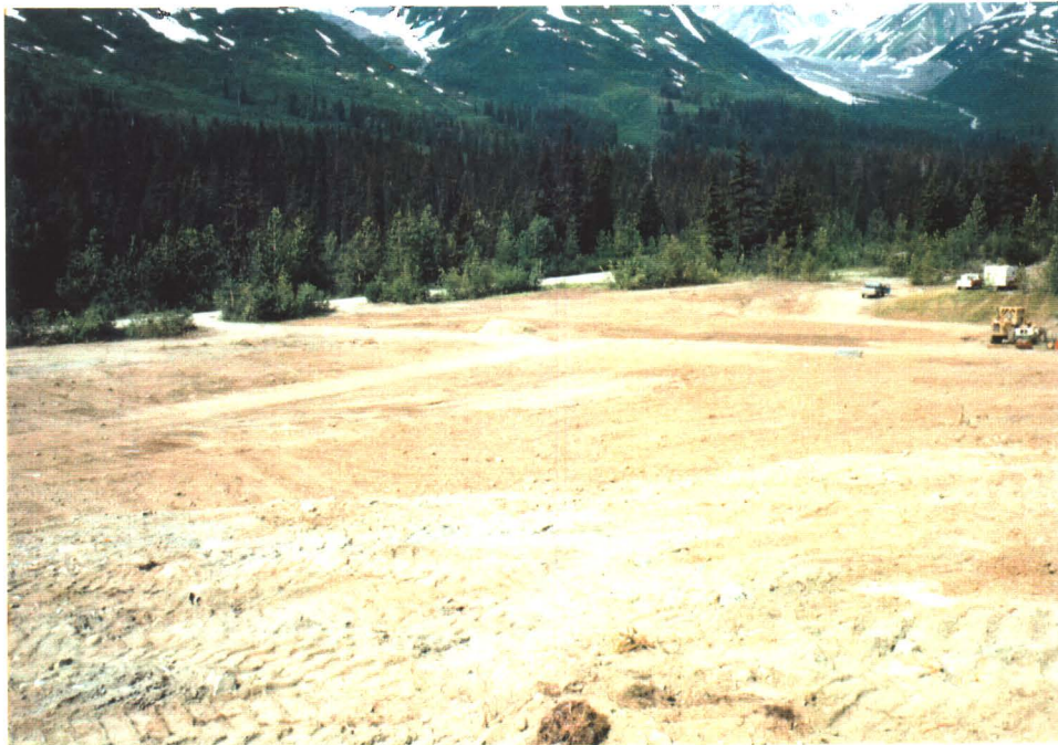
Photograph 2.4: Grading following demolition activities at Border Station
