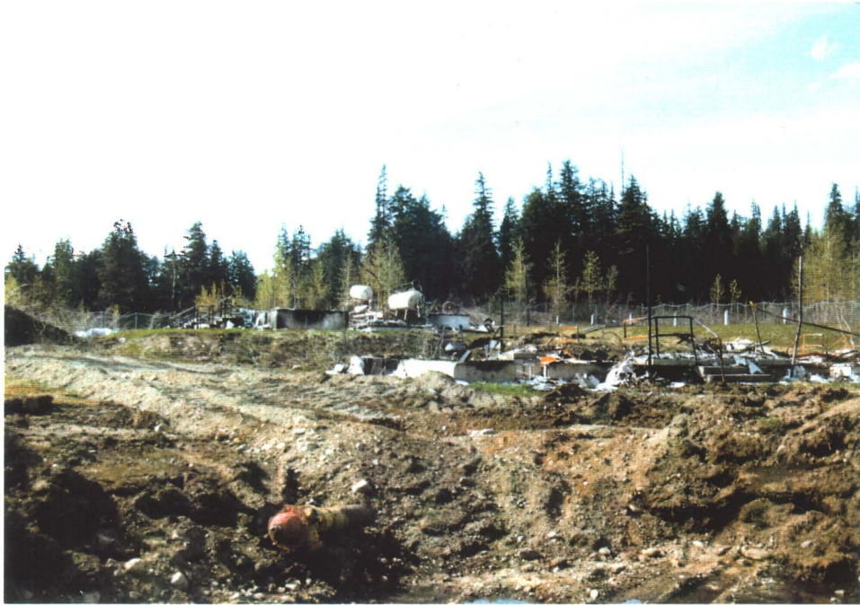
Photograph 2.3: Removal and demolition of facilities at Border Station.
