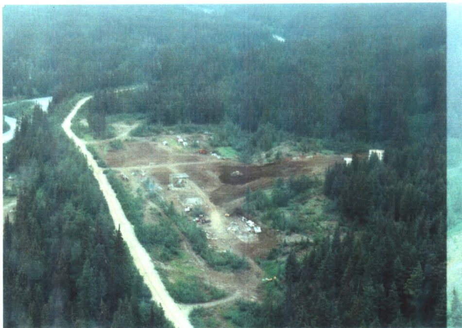
Photograph 2.2: Aerial view of salvage operations at Border Station.
