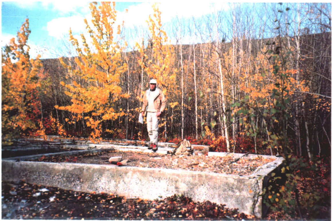
SITE 17C - Canol pump house foundation
