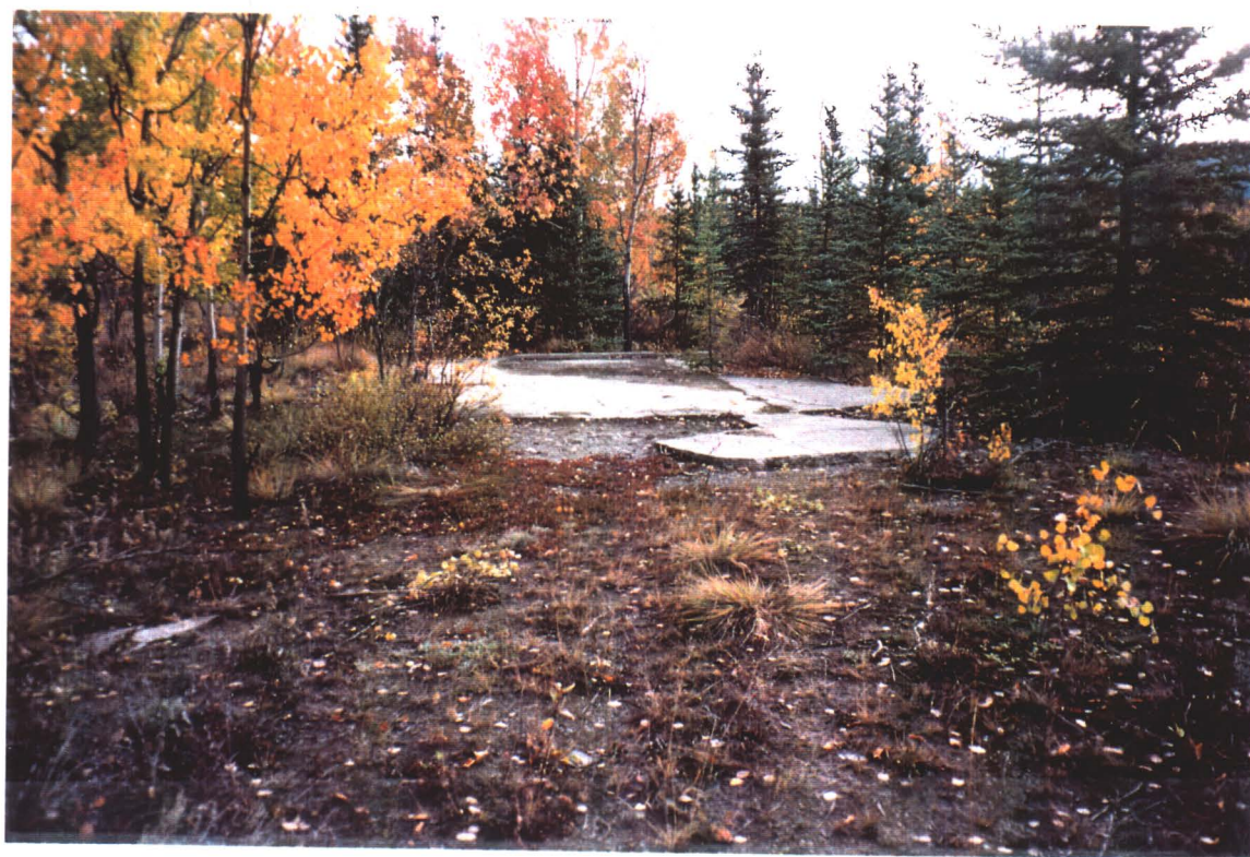
SITE 16 - Concrete foundations
