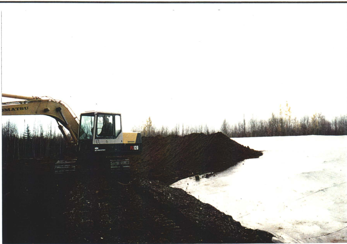
PHOTO 14: Containment Cell - Coverage of containment cell with layer of topsoil.
