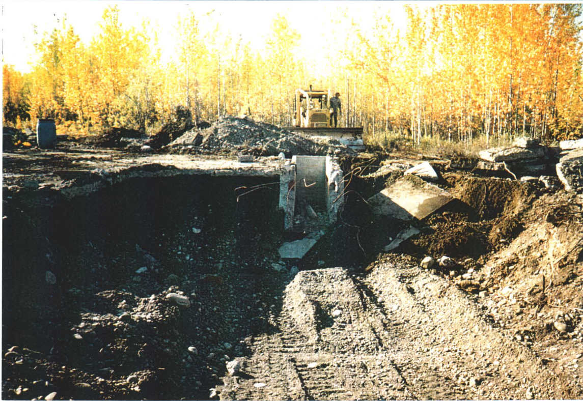
PHOTO 6: Garage - Photograph of large concrete garage pit with sump removed
