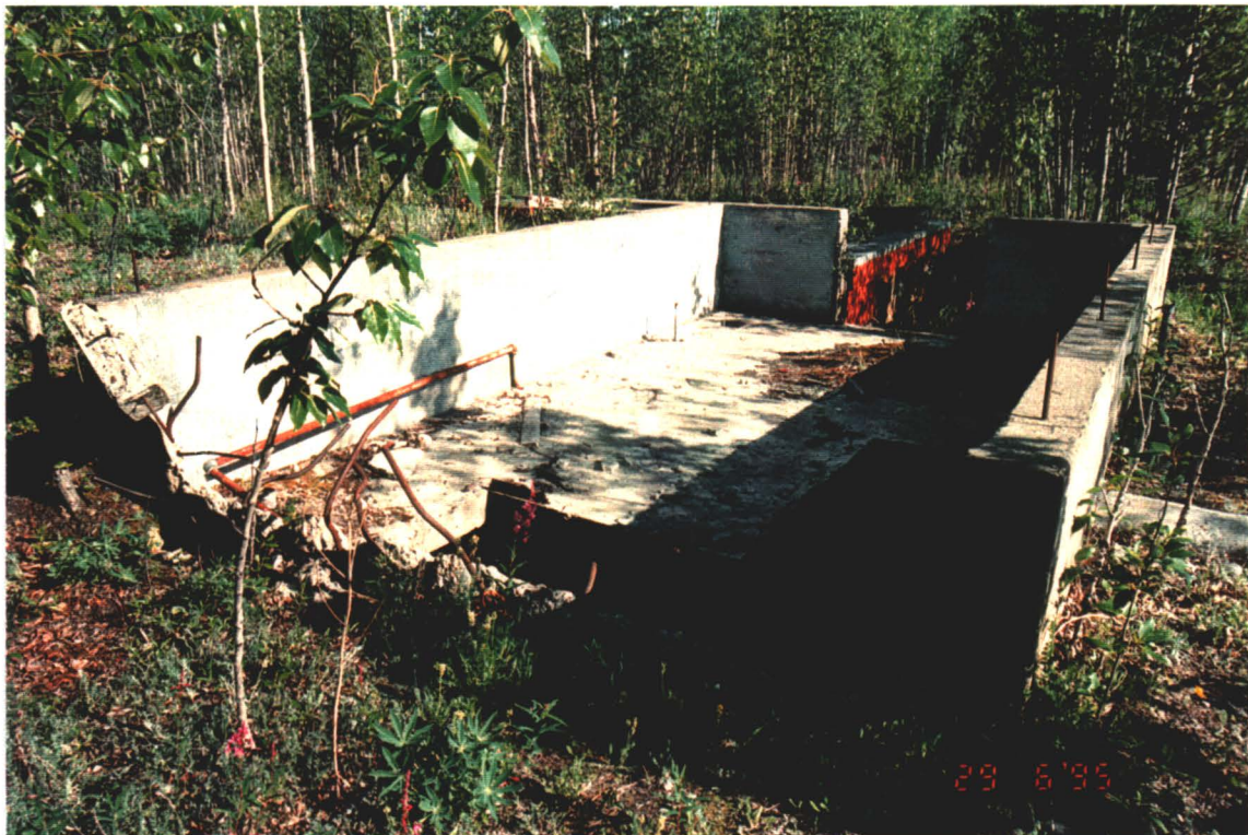
Photograph III-9: A close-up of the Pump House Foundation prior to cleanup.
