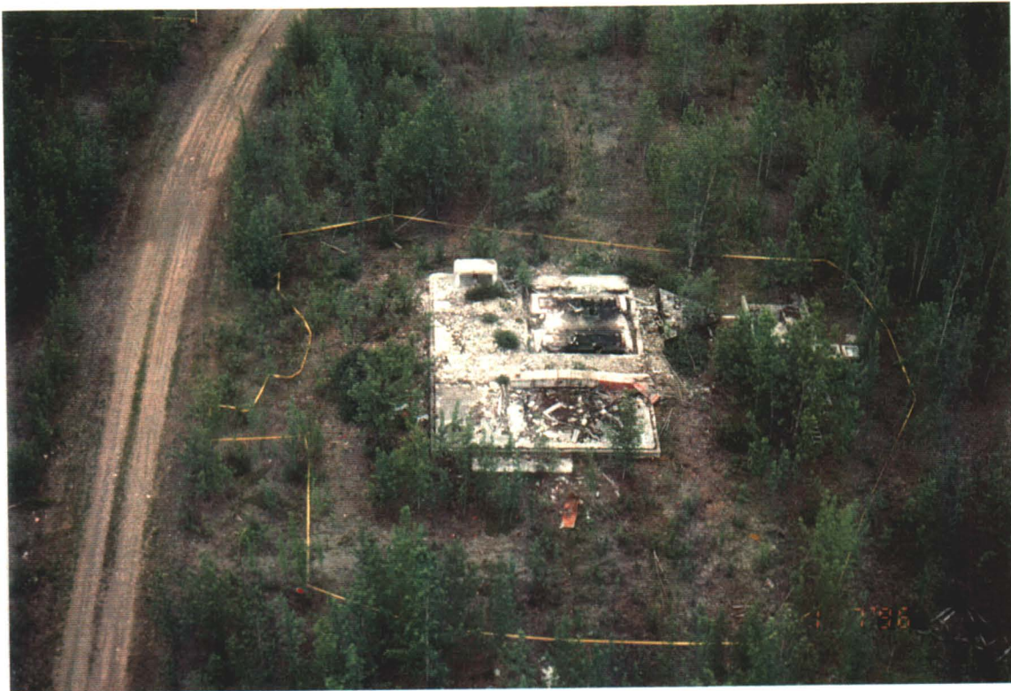
Photograph III-8: The Powerhouse and Pump House Foundations as they appeared in 1996 before their cleanup.
