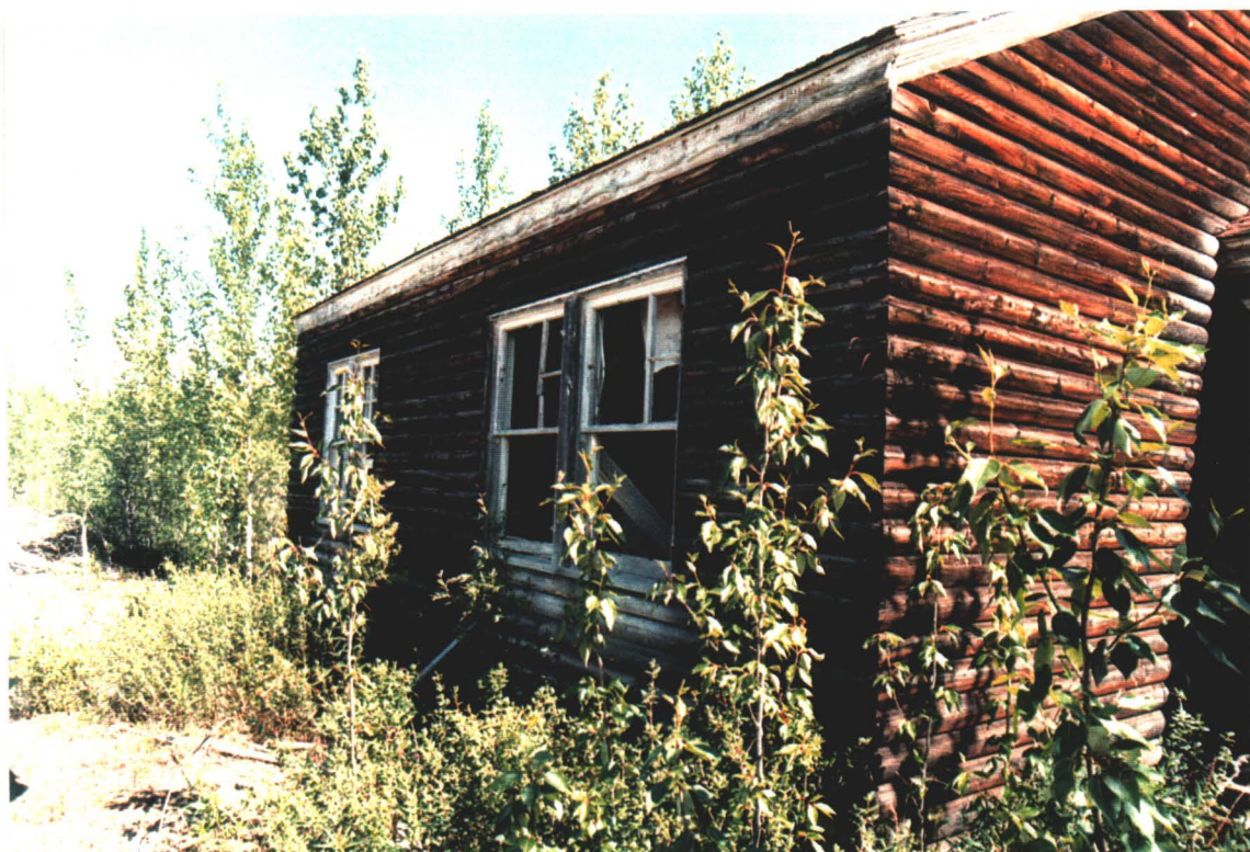
Photograph III-13: The Married Quarters as they appeared prior to cleanup in 1996.
