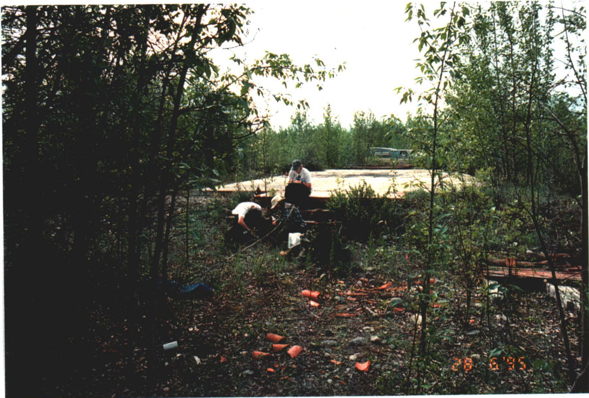
Photograph III-6: The Warehouse Foundation as it appeared prior to cleanup.
