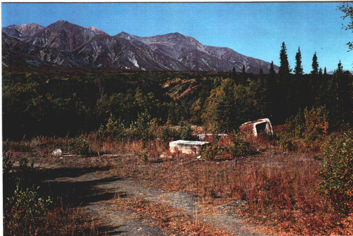
The site looking west. Remnants of old foundation are located in centre of photograph.
