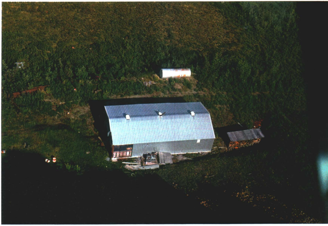
Photograph # 13: Shop, core rack, generator, ST - 1.
