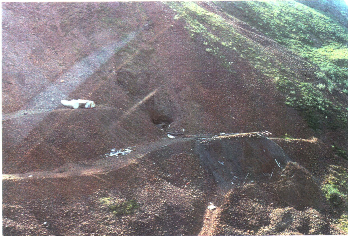
Photograph # 6: Same as above. Note recent land slide onto tanks.
