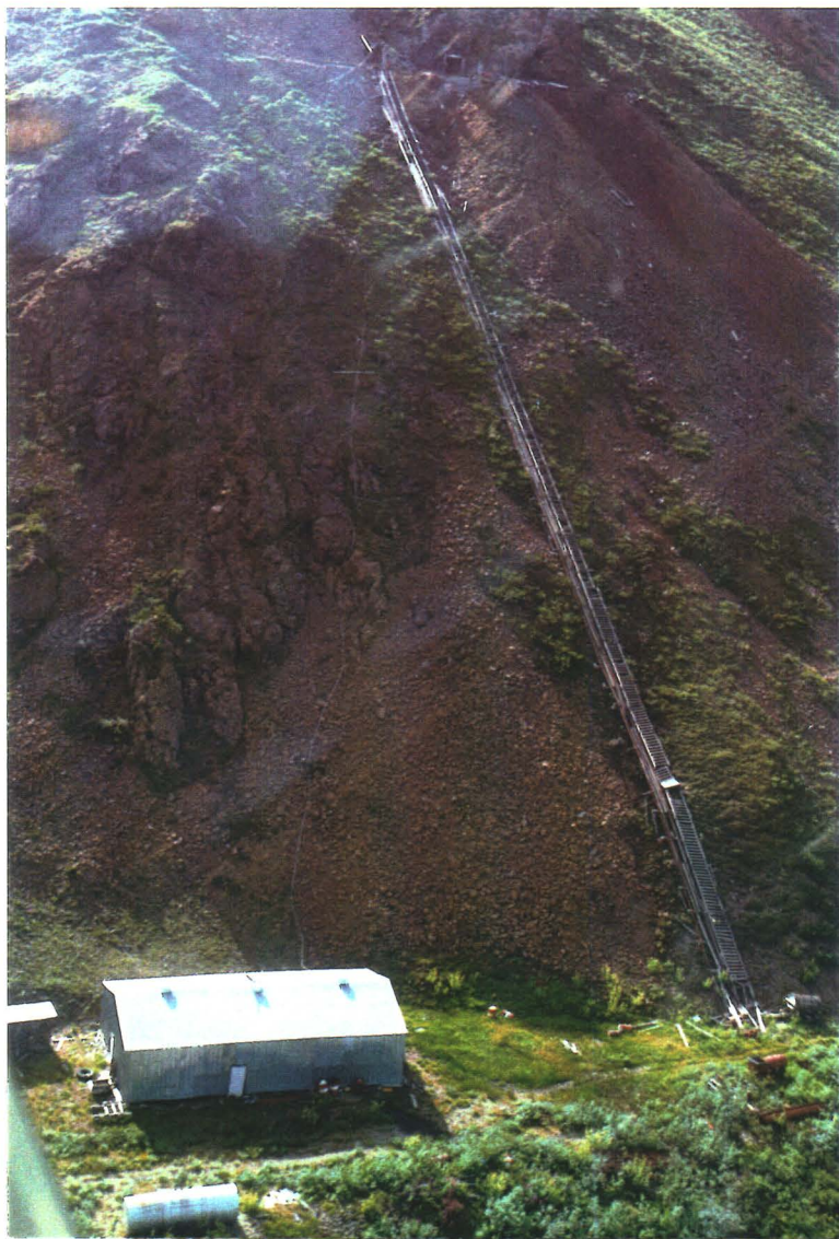
Photograph # 7: 3880 Adit, shop.
