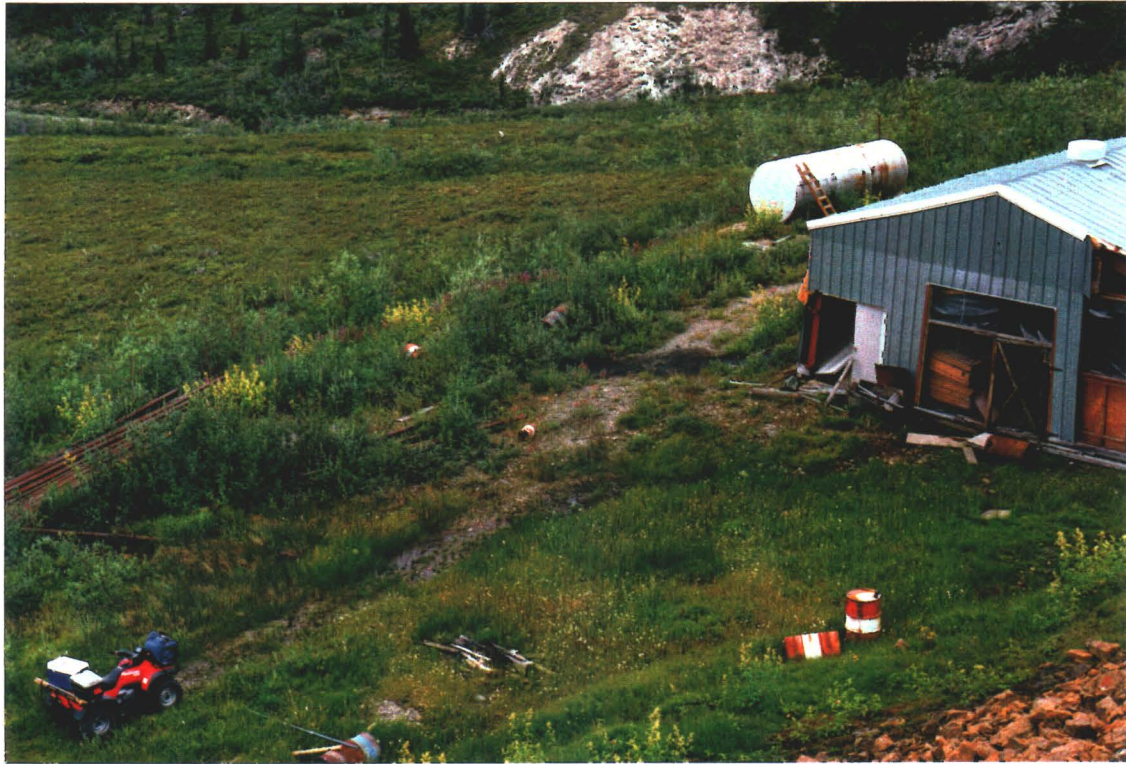
Photograph # 9: Shop, storage tank ST - 1 at left side.
