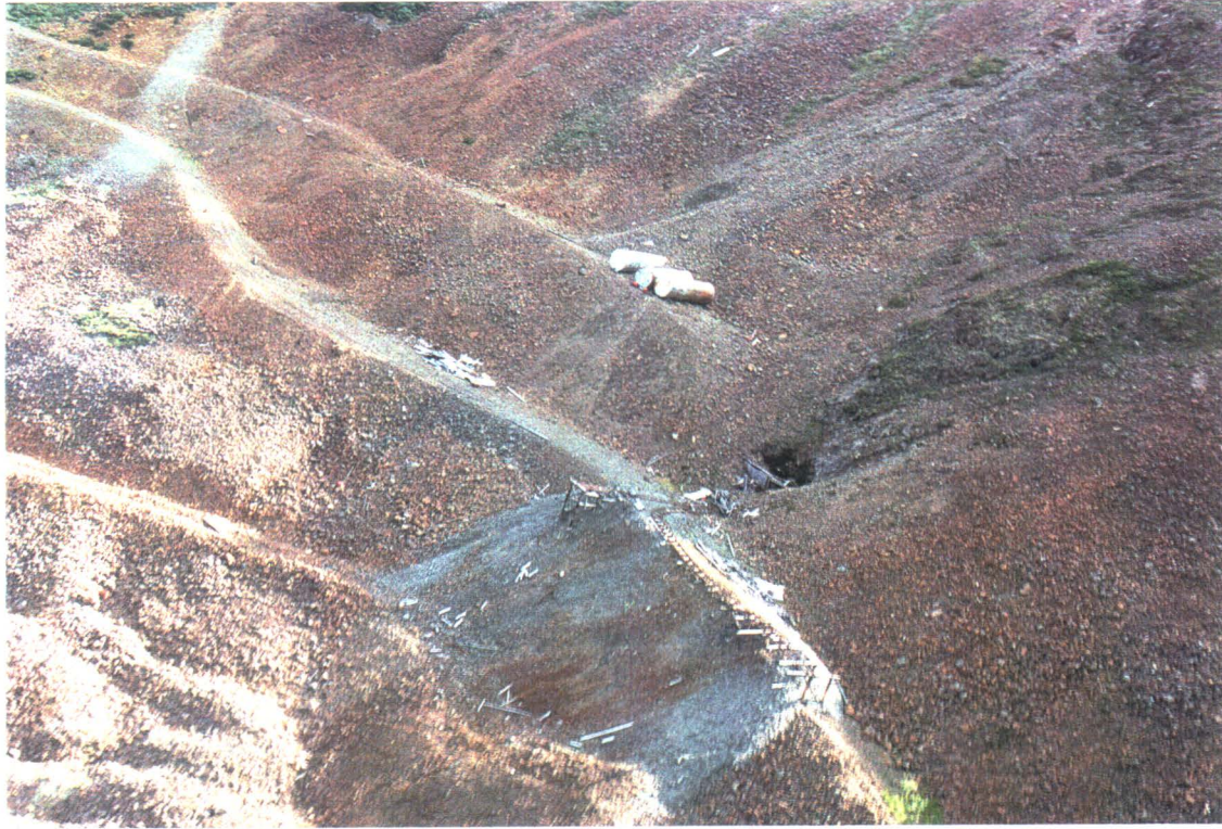
Photograph # 5: 3680 Adit, Storage tanks ST 5, 6, and 7. Contain 66,170 litres diesel fuel.
