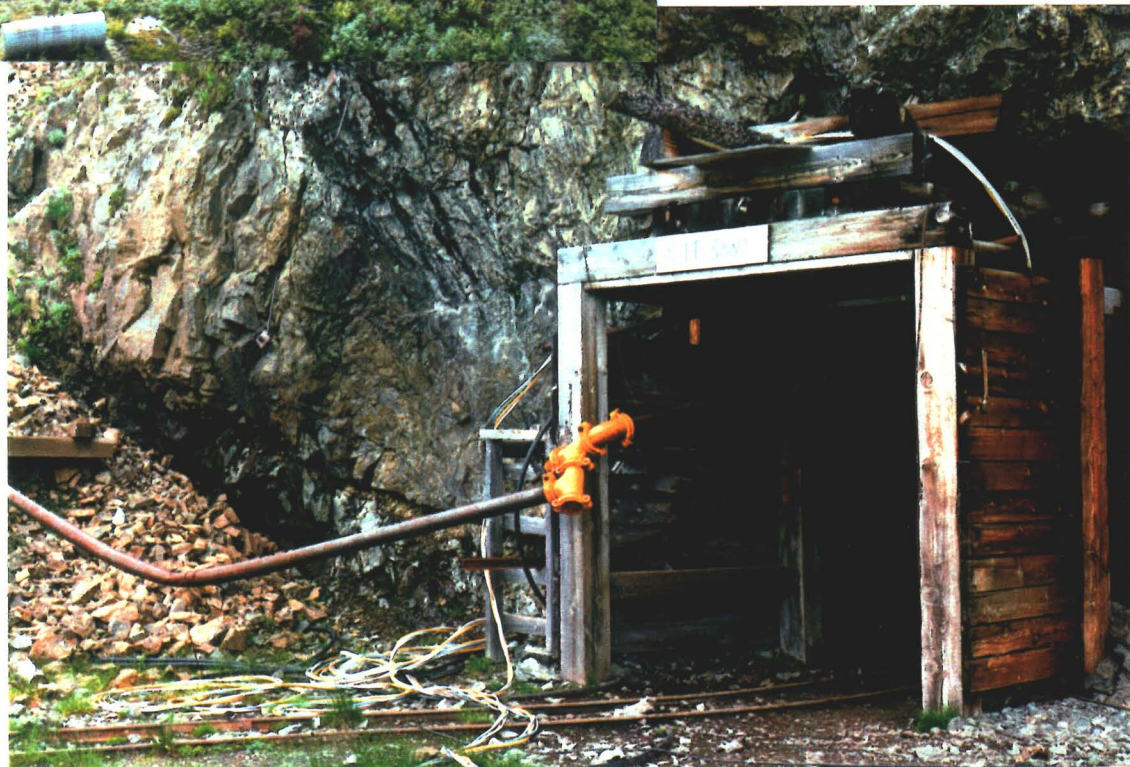
Photograph # 8: 3880 Adit opening.
