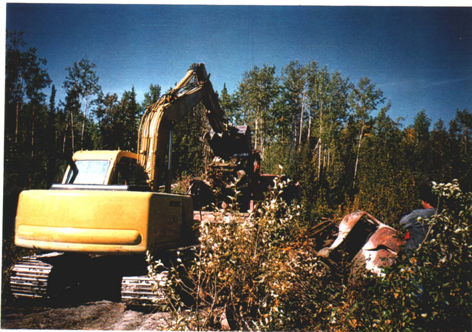
Photo # 9 - Removal of debris during heavy equipment clean-up operations.
