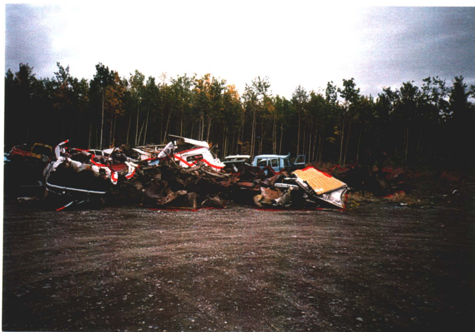
Photo # 10 - A portion of surficial debris removed near completion of heavy equipment clean-up operations. Photo taken at Haines Junction landfill.
