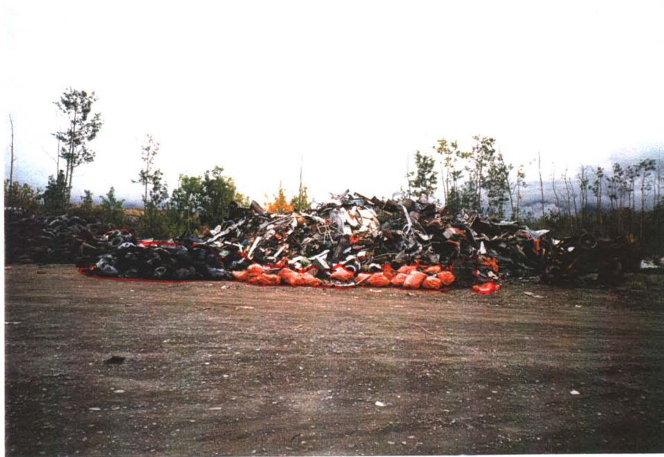
Photo # 6 - Surficial debris removed near completion of hand clean-up operations. Photo taken at Haines Junction landfill.
