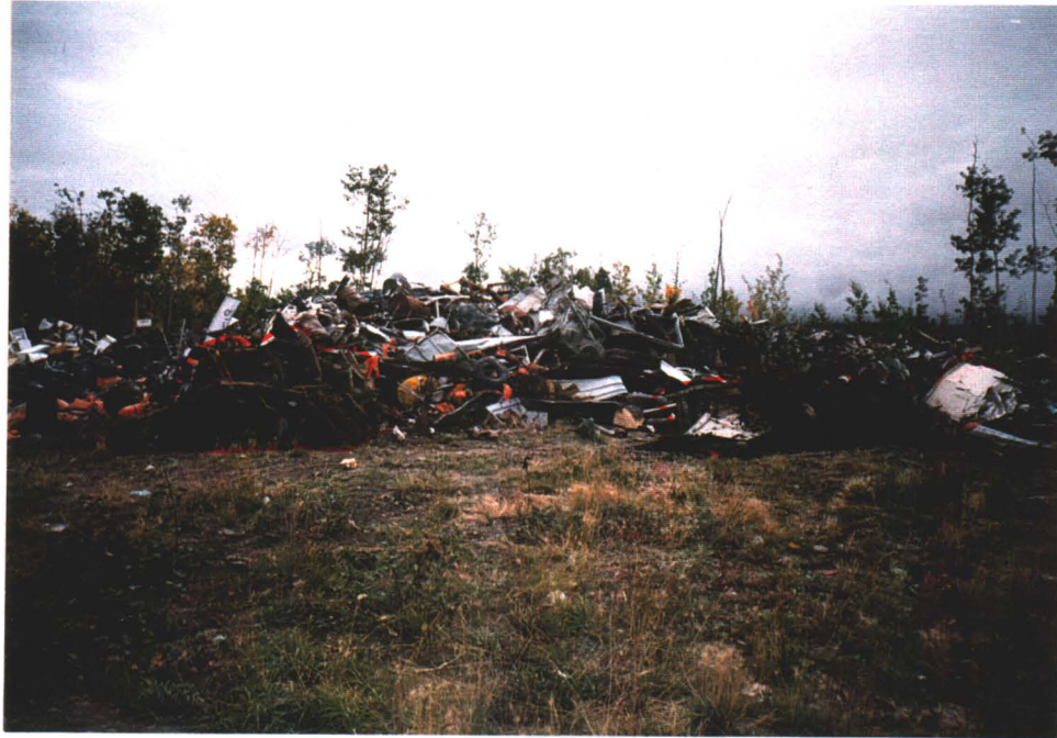
Photo # 11- A portion of surficial debris removed near completion of heavy equipment clean-up operations. Photo taken at Haines Junction landfill.
