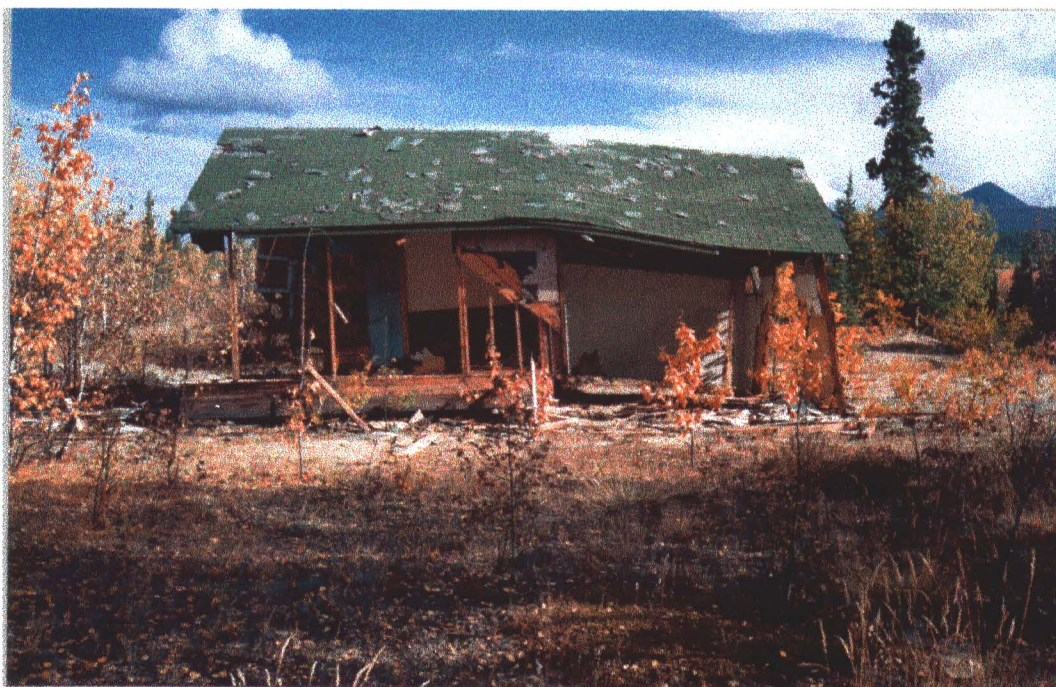
Photograph 03 - Takhini River - Exterior wall scavenging, looking east.
