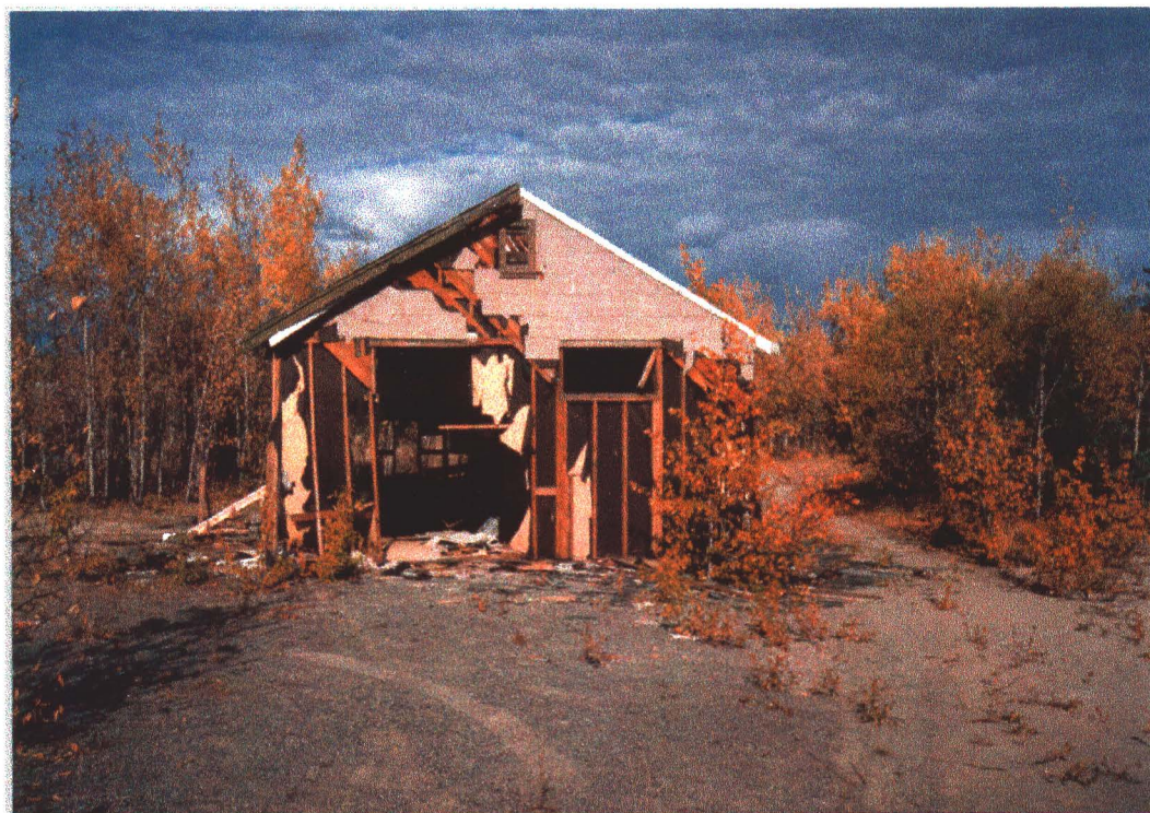
Photograph 02 - Takhini River - Exterior wall scavenging, looking north.
