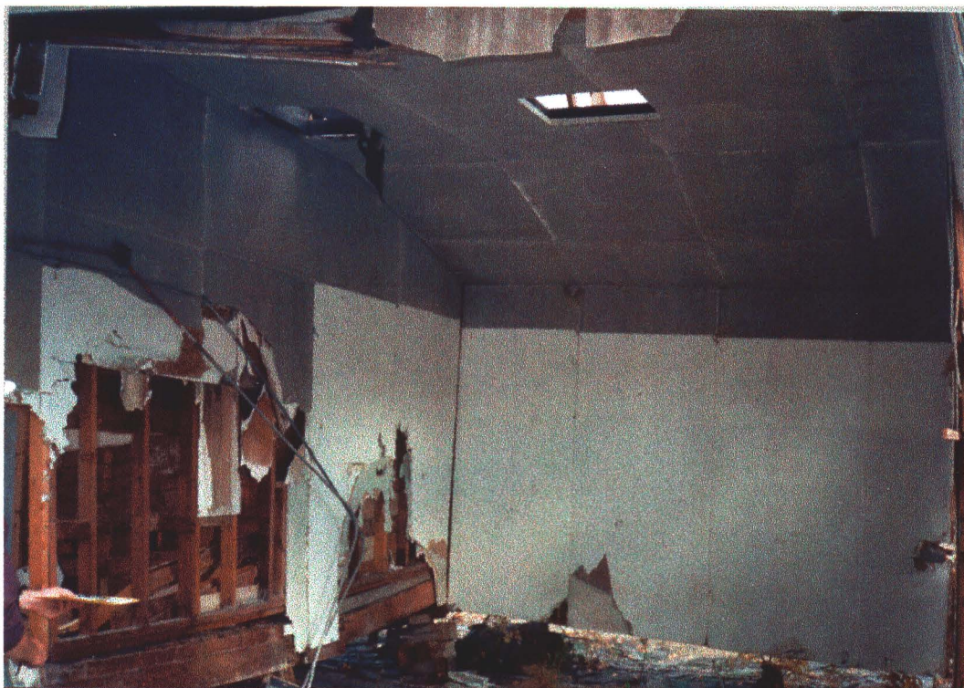
Photograph 04 - Takhini River - Grey asbestos board above drywall, looking east.
